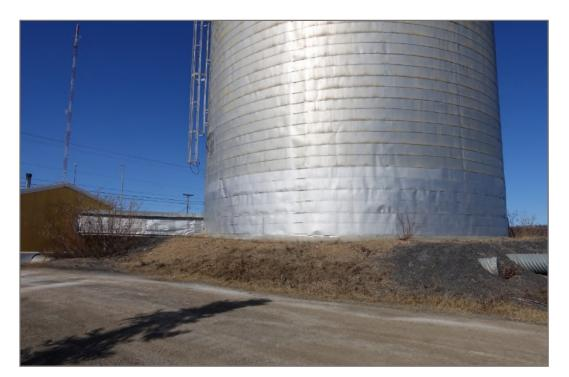
Photo 26: Looking northeast at sloughing on west side of tank pad, with much more material lost than on sides with pipes extending out. (Photo credit: Stantec 2017)
