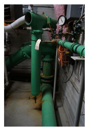
The existing reheat piping was modified by the Town and replaced with PVC pipes. The tie-in point for water reheat system to the new potable water tank is not available in the existing piping. The design should incorporate adding a tie-in point for the water reheat to the new tank.
