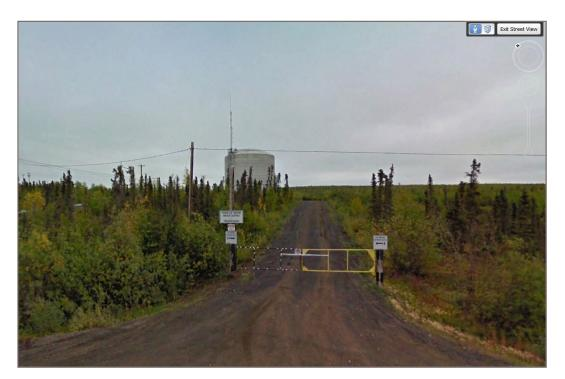
Photo 6: Looking east from Marine Bypass Road at gated entry to tank access road. Culvert under access road is just west of gate. Overall drainage at south site is west towards Marine Bypass Road, then south through culvert. (Photo credit: Google Earth 2017)
