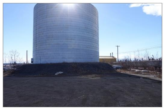
Photo 25: Looking west at sloughing of east side of tank pad. Variation in fill cover and pipe angles also visible. (Photo credit: Stantec 2017)
