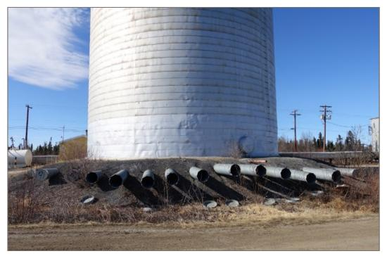
**Photo 23:** Looking north at ventilation pipes in tank pad, valve house in background left and filter plant in background right, with utilidor. Note variation in fill cover and pipe angles. (Photo credit: Stantec 2017)
