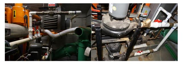
The Town indicated that the existing utilidor to the Valve House (Building #2) has experienced issues recently with freezing of pipes. The Town requested Stantec to consider rehabilitating the utilidor or replacing it with insulated pipes.
