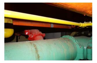
The piping for the new potable water tank to be consistent with the existing piping and use the same butterfly valves with lever operator. The Town will provide the existing butterfly valve make and model to Stantec.
