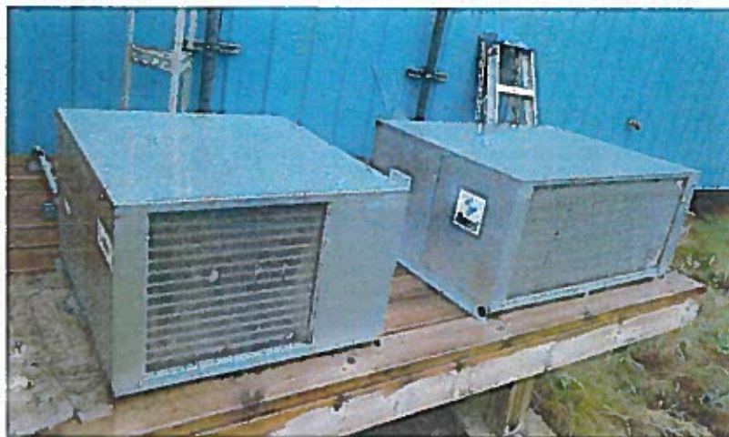
Photo 37 - Cooler/Freezer Condensors
