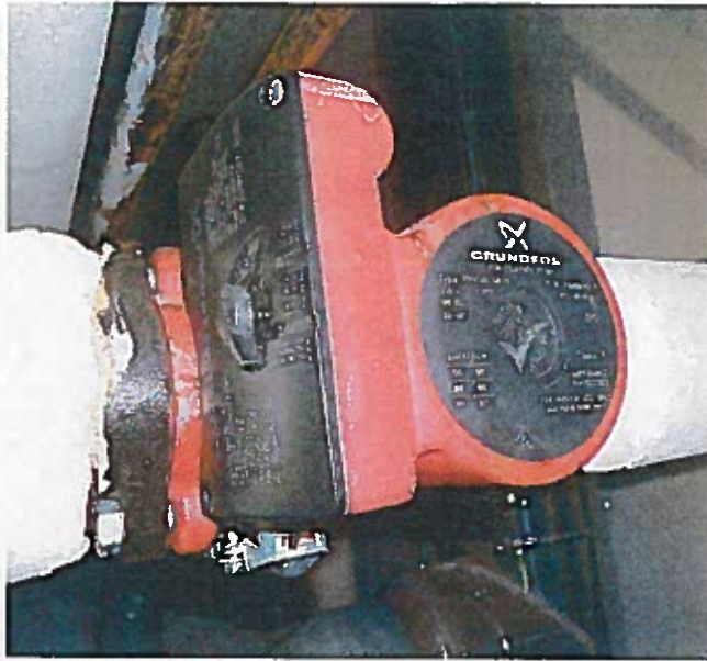
Photo 21 - Boiler Circulation Pump
