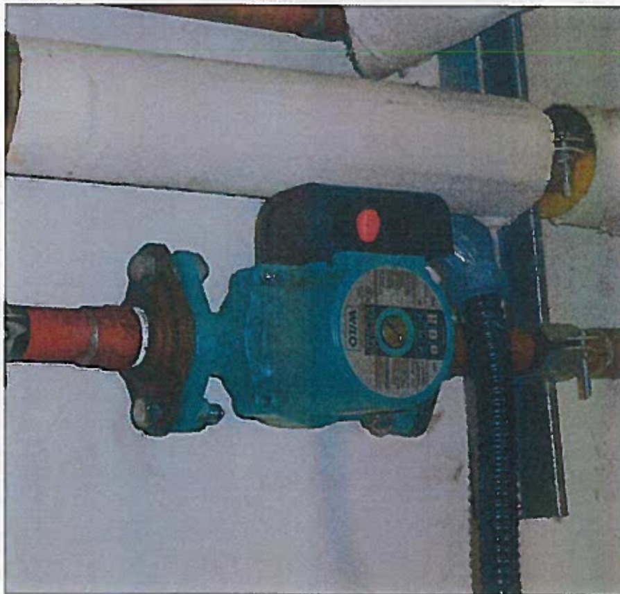
Photo 22 - Domestic Hot Water Circulator
