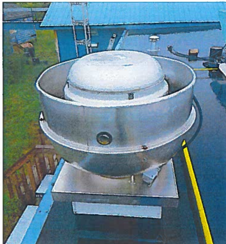
Photo 28 - Range Hood Exhaust Fan
