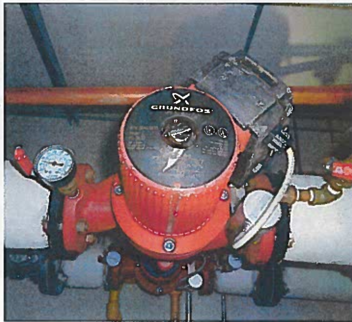
Photo 20 - Primary Circulation Pump
