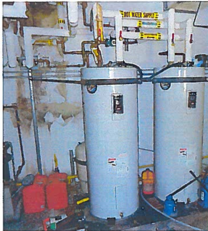
Photo 32 - Electric Hot Water Tanks
