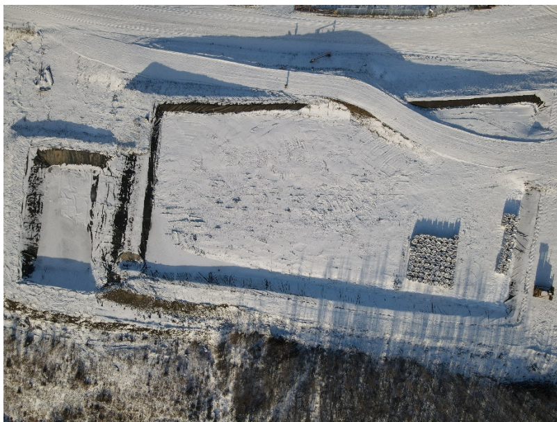
Photo 1: Constructed Facility, October 12, 2021
