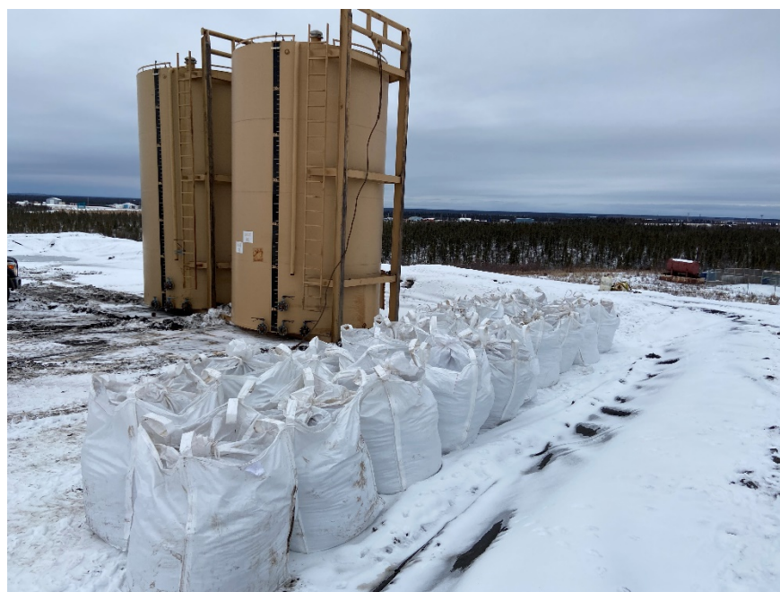
Photo 2: Facility ASTs, October 12, 2021
