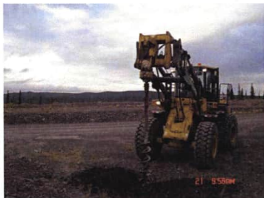
Photo 38 : Drilling borehole for monitoring well installation 02-MW06-01 at APEC 02, FFTA.
