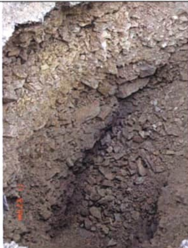
Photo 7 : View of test pit sidewall at 01-TP-06-24.
