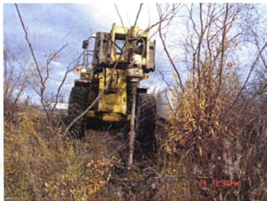
Photo 39 : Drilling borehole for monitoring well installation 08-MW06-01 at APEC 08, Shell Lake.
