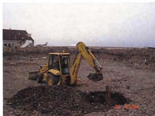
Photo 40 : Monitoring Well 01-MW06-01 was installed inside a test pit due to collapsing material during drilling.
