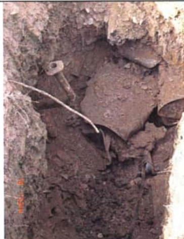
Photo 35 : Debris encountered at test pit 10-TP06-03.
