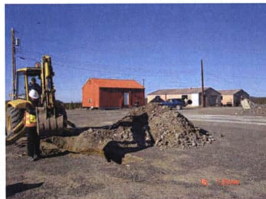
Photo 5 : View toward west at 01-TP06-21. Sampling soil from bucket for deep samples.
