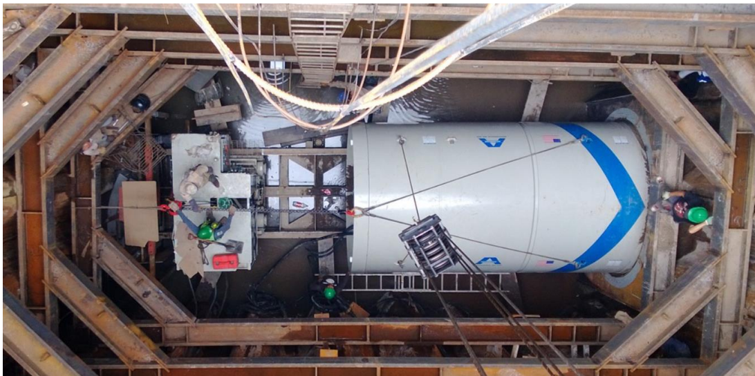
Figure 11. 5200 Press Unit Setup on Rails
