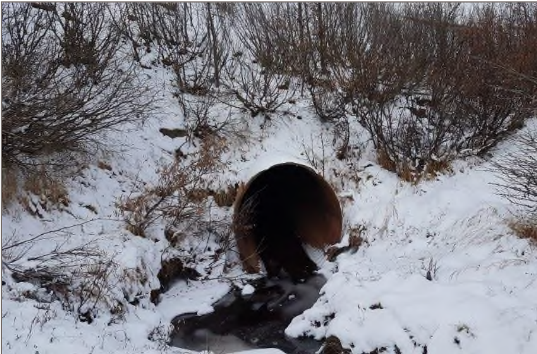
Photo 6: Closeup of the lower 1.8 m diameter culvert on the north side of the highway embankment.
