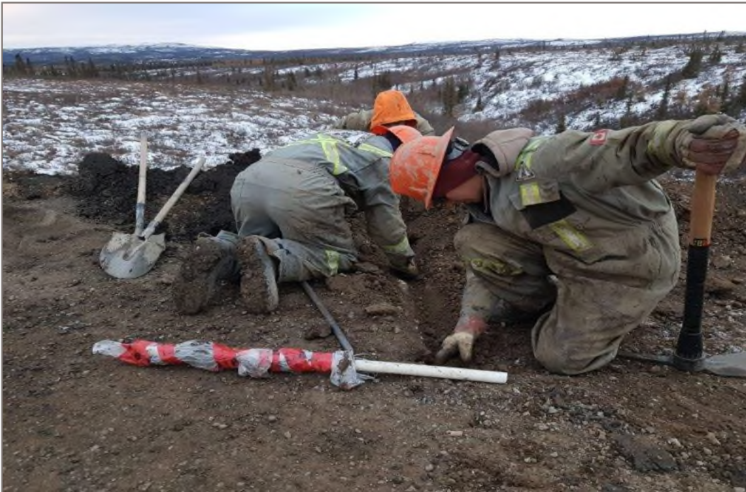
Photo 8: Clearing thermistor cable trench for BH-04.
