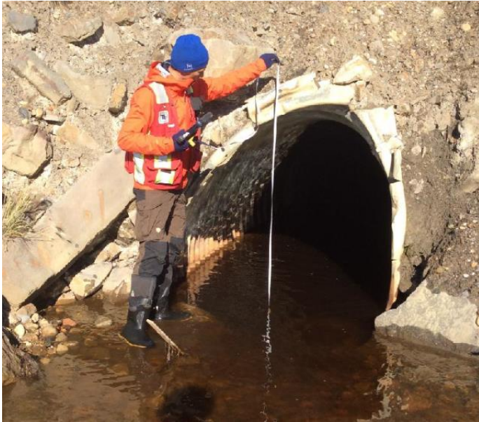
Photo 99: Crossing 33/25 distorted outlet.
