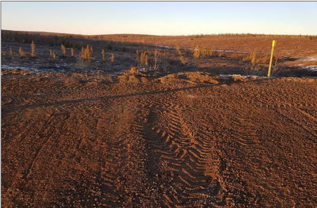
Photo 20: Highway backfilled from thermistor cable trenching for BH-05, facing north.
