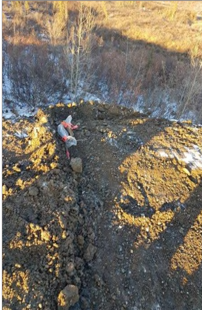
Photo 21: Thermistor cable trench for BH-05.
