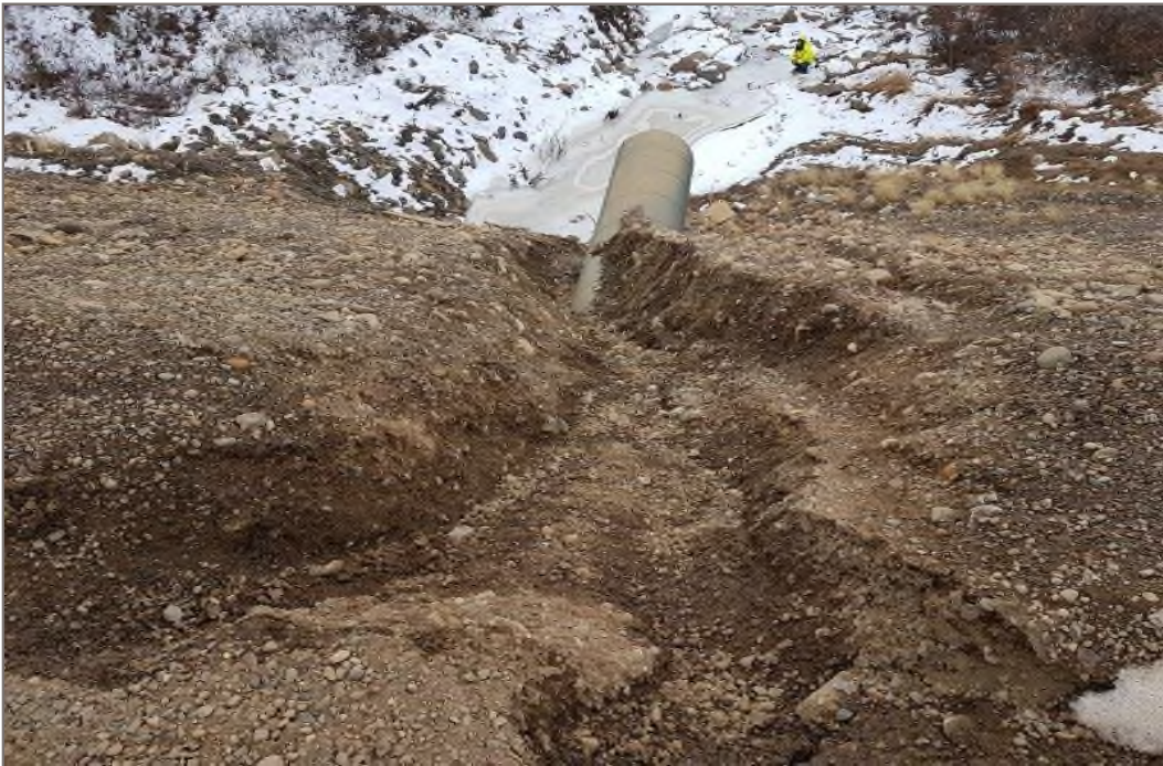
Photo 4: Erosion above top culvert on south side of embankment.
