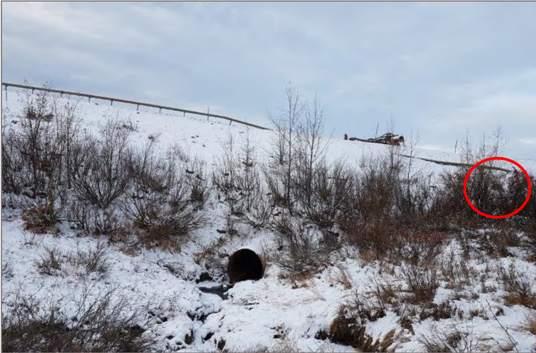
Photo 5: Both culverts on the north side of the highway embankment; view looking south. The larger lower 1.8 m culvert is centred in the photo. The upper 1.2 m culvert is circled.
