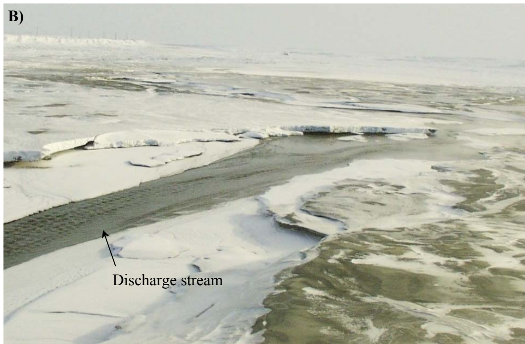
Figure 1.11: A) View (looking northwest) of Dyke C, in July 2001. The arrow indicates the location of the discharge spigot. Note the low angle fan created by the processed kimberlite fines discharging into the LLCF. Also note the water that is flowing over the fan. B) View (looking south from Dyke C) of the discharge stream from spigot in March 2001. Note how the stream spreads over the surface of the fan in the upper part of the photo.
