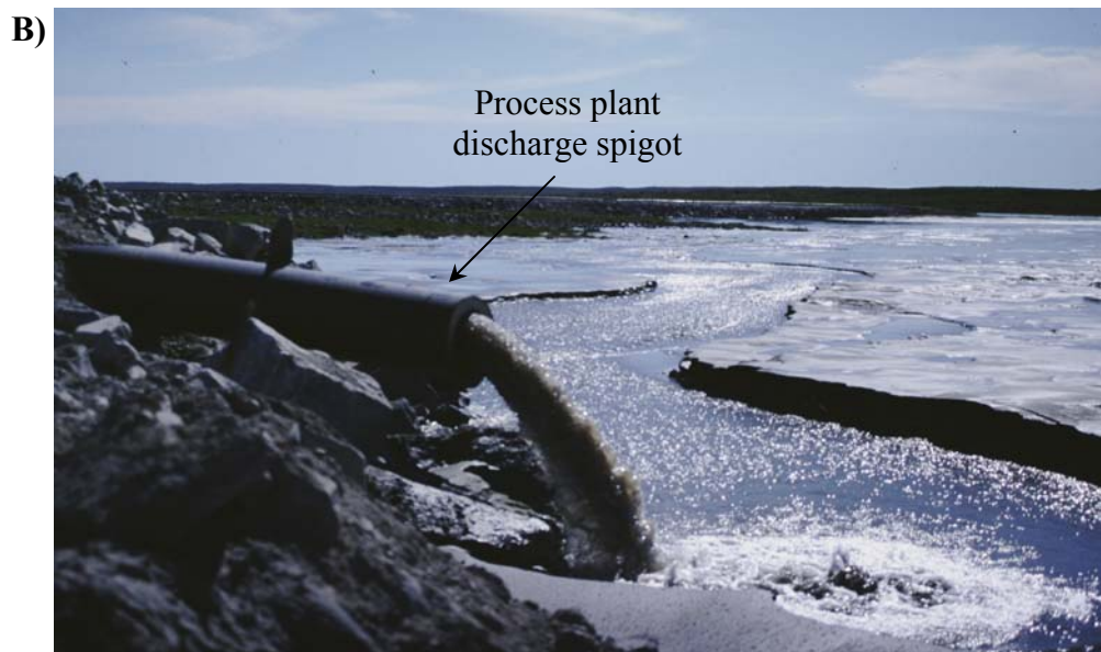
Figure 1.5: A) Coarse kimberlite reject pile adjacent to the mineral processing plant. From here, this material is hauled to a sub-aerial disposal site. B) Spigot discharging kimberlite fines and process water from the mineral processing plant to the kimberlite containment facility. The fines are hydraulically pumped at a solids content of approximately 40% to 50%.
