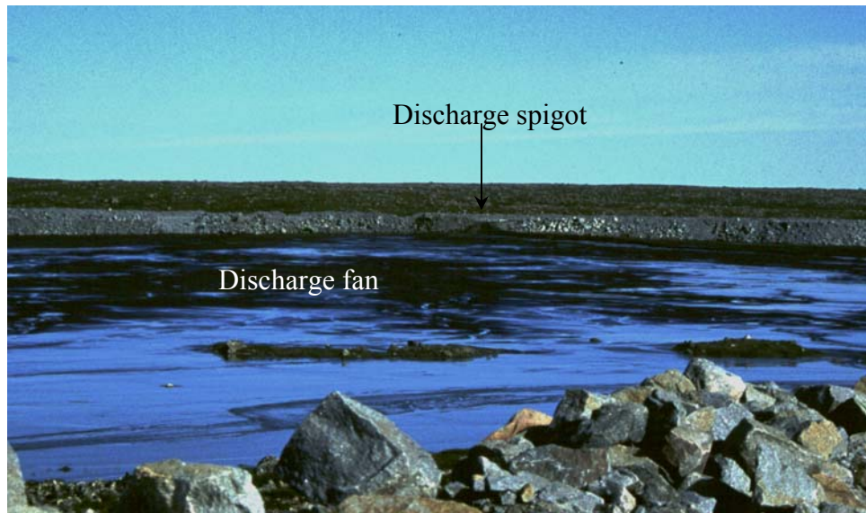
Figure 3.8: A) Spigot discharging process plant effluent into the LLCF. Samples of this material were collected by placing a plastic 10-gallon bucket into the discharge stream. B) View of Dyke C, looking north, and the low-angle fan created from the process plant discharge.
