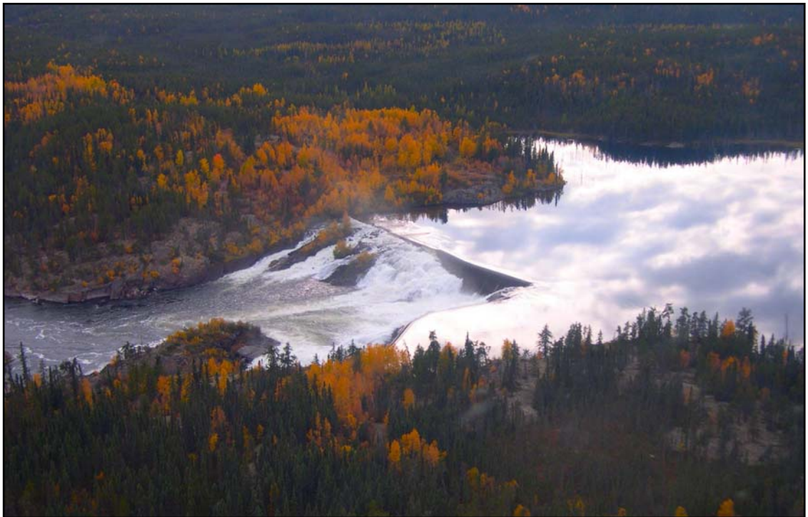
Plate 8-5: South Valley Spillway
