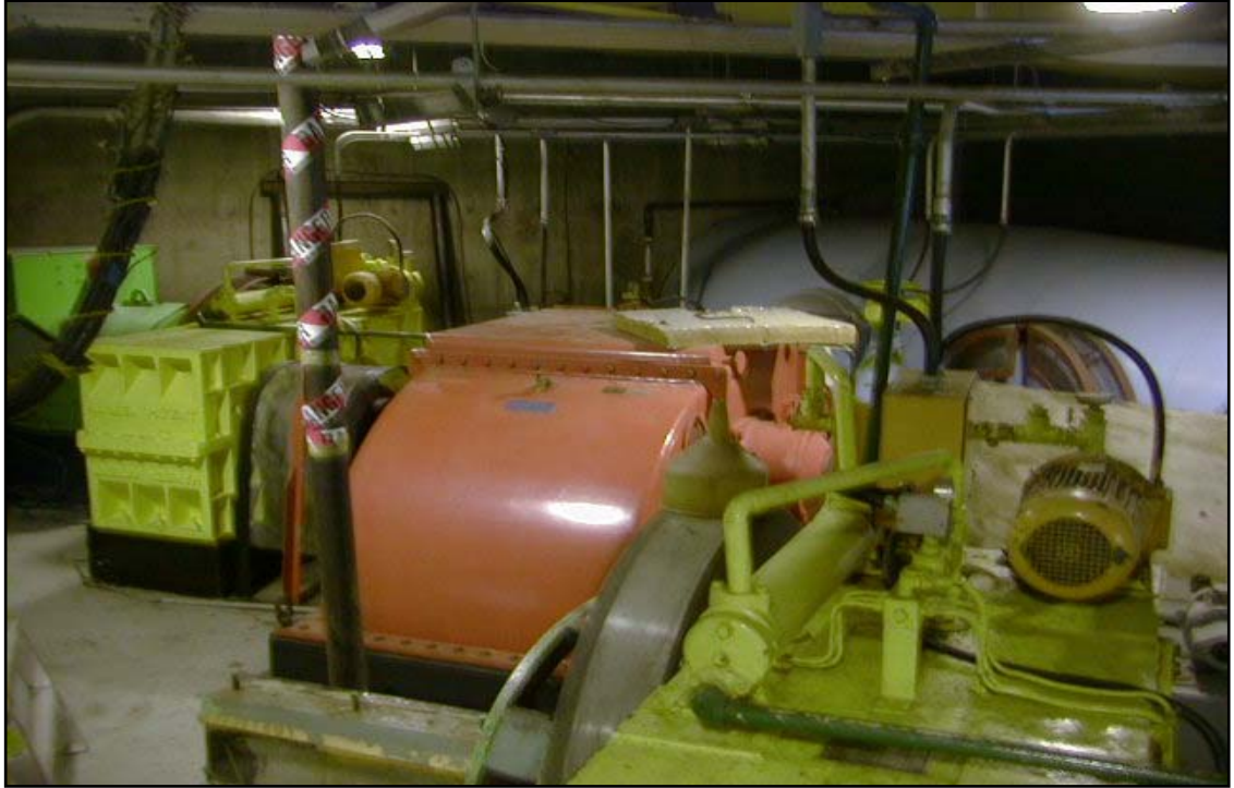
Plate 8-12: Ossberger Turbines
