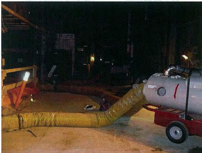
Photo 12 – Warm air provided during pour and curing
