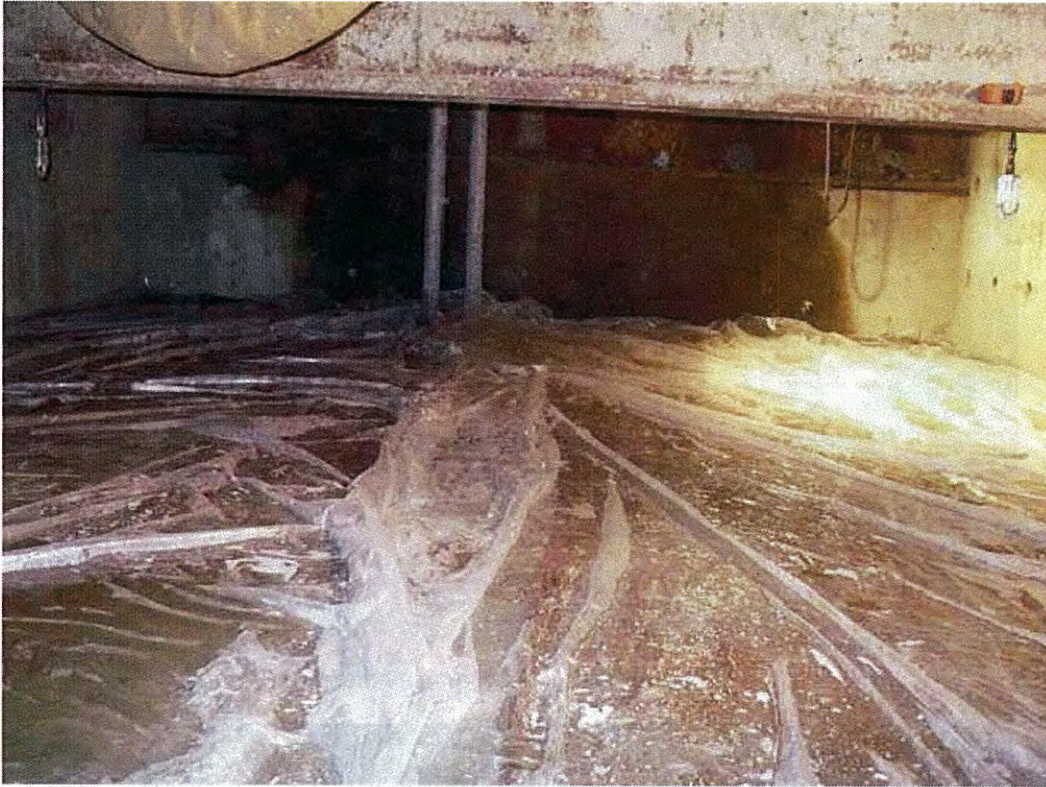
Photo 13 – Concrete curing under burlap and polythene
