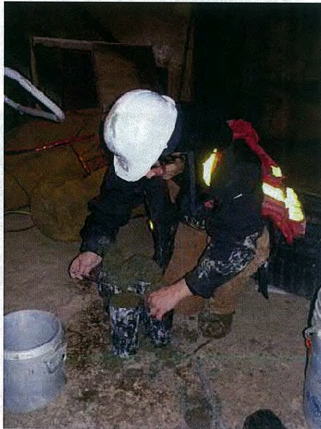
Photo 10 – Cylinders being cast
