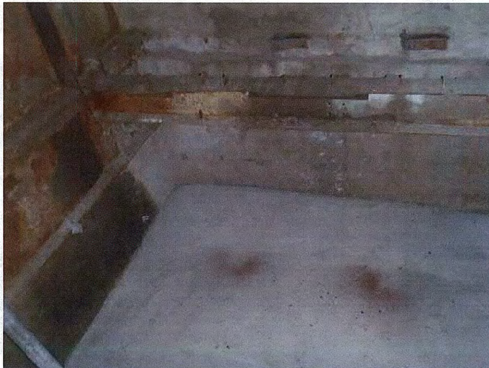
Photo 16 – Rob Shaft Concrete Cap
