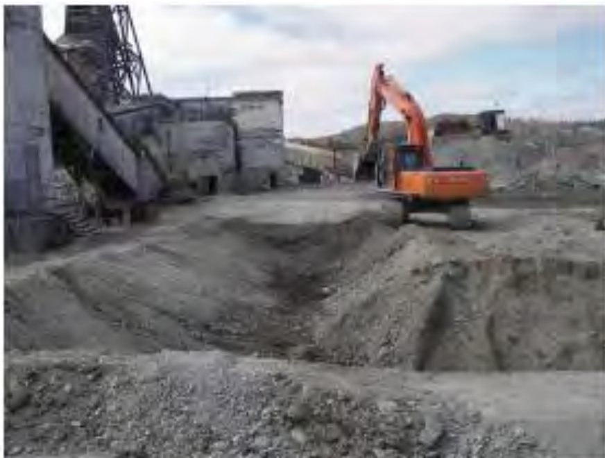
Figure 13. Removing contaminated soils [PR#348 p32]
