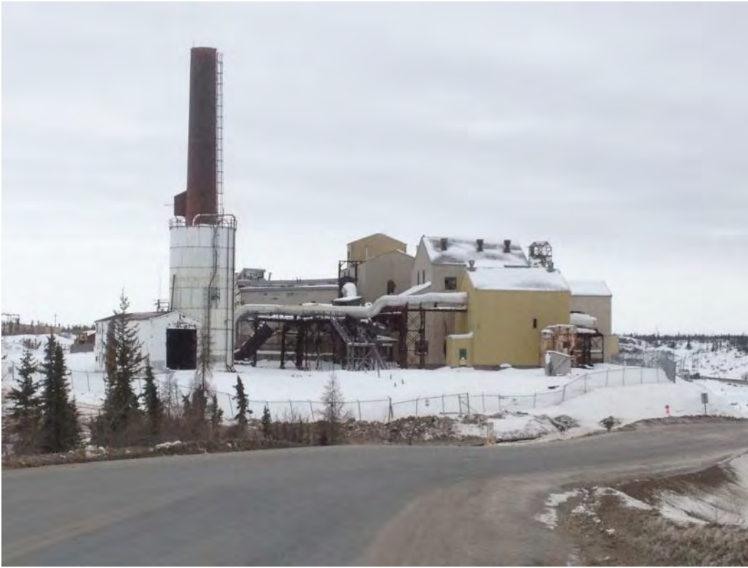
Figure 11: Giant Mine roaster complex (photo: Review Board)
