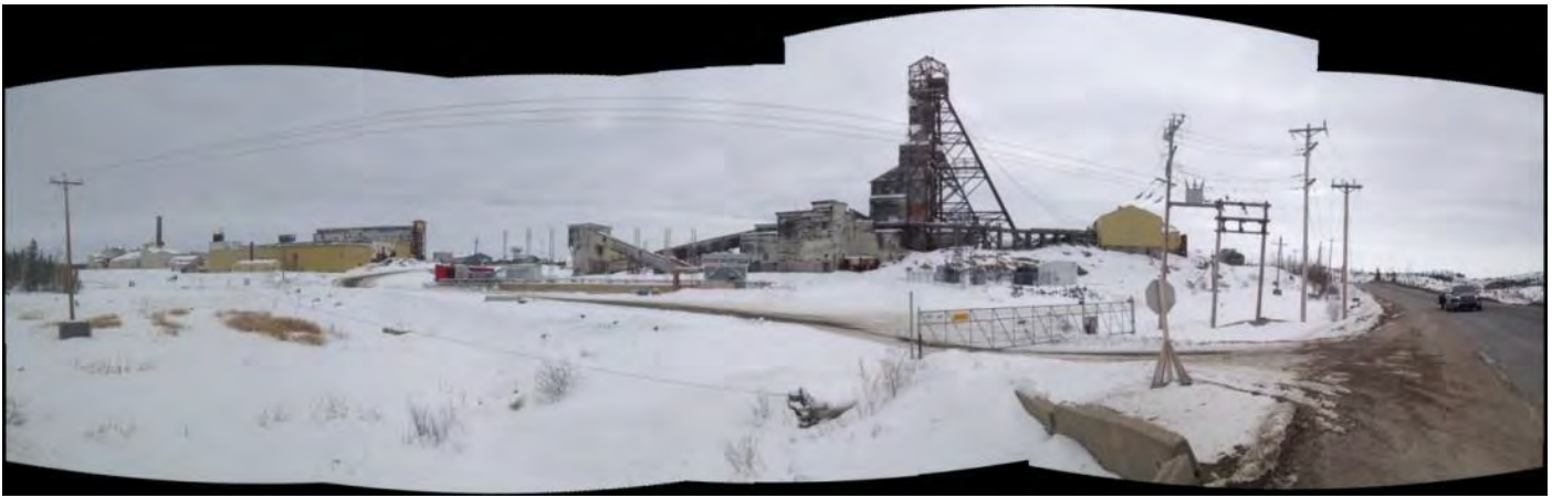
Figure 10: Buildings and infrastructure at Giant Mine
