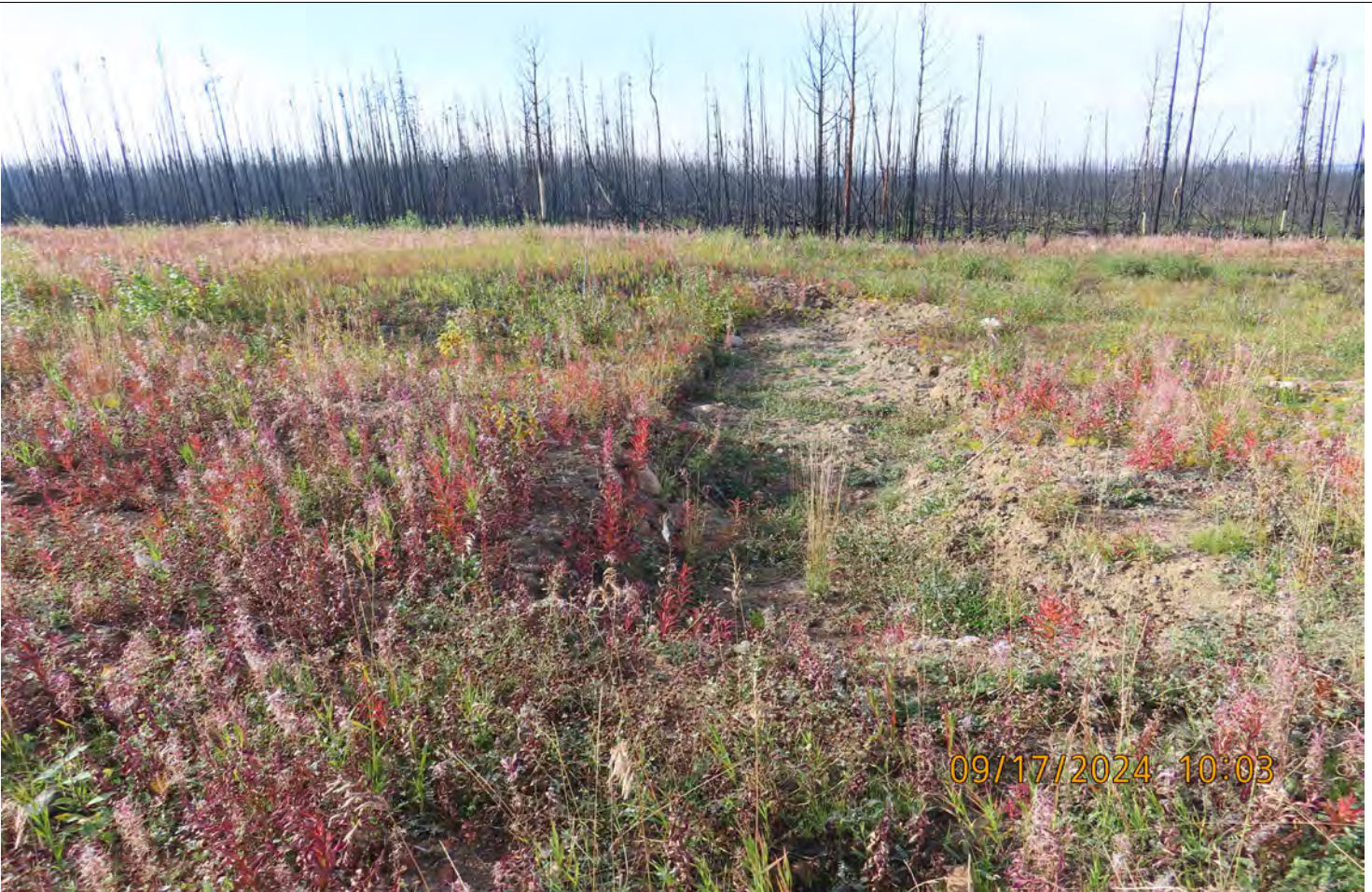
Figure 30 Wellsite A-73 – Backfill required following winter abandonment work
