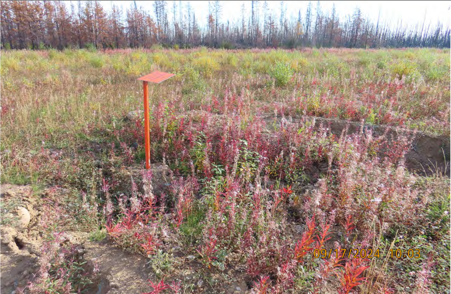
Figure 30 Wellsite A-73 – Backfill required following winter abandonment work
