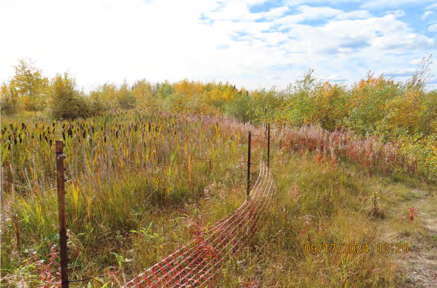
Figure 28 Battery camp – Sewage lagoon snow fencing not properly attached to posts
