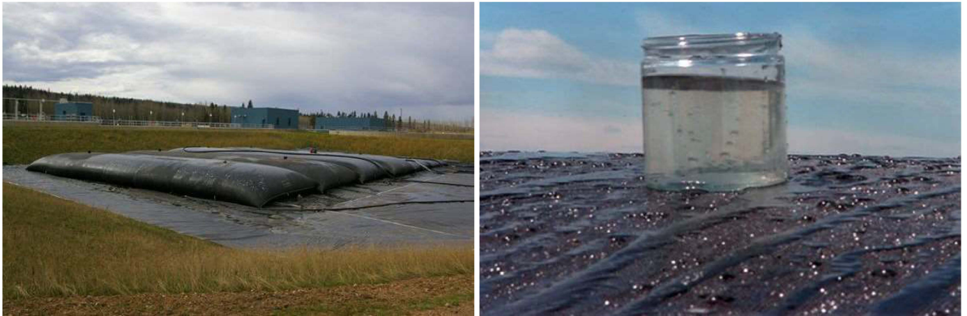
The first picture shows dewatering tubes at a municipal WWTP. The second picture shows filtrate from a Geotube that was processing sludge from a municipal anaerobic lagoon.
