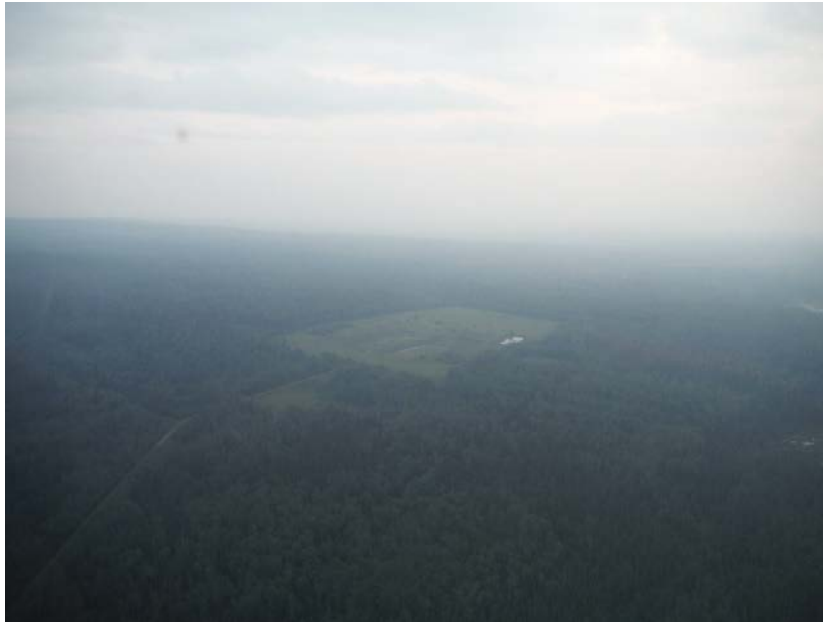
Photo 1 View northeast across the Plant Site and access road
