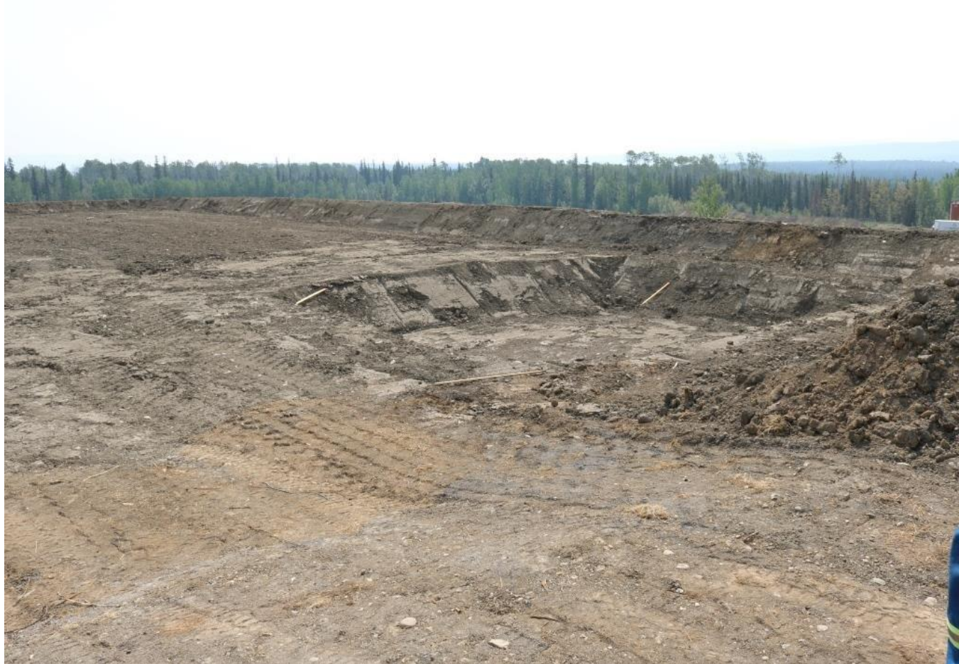
Figure 18 Prepped area for contaminated soil
