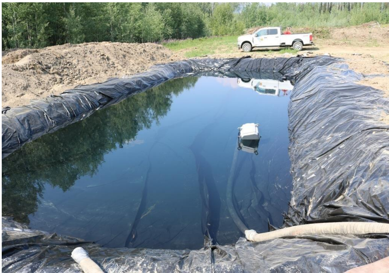
Figure 12 Lined cell with final product- clean (treated) water
