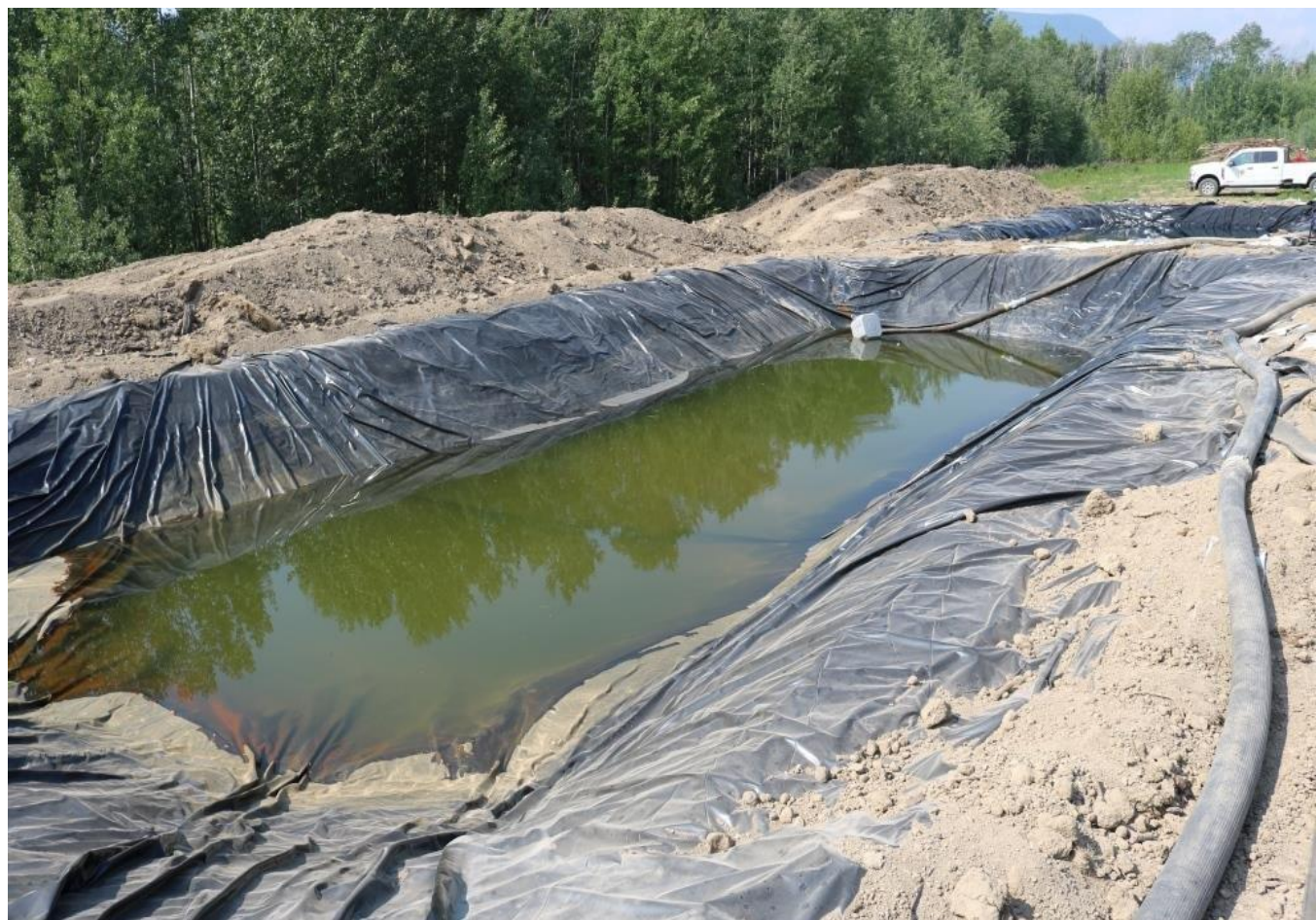
Figure 10 Water stored in lined cell to go through reverse osmosis
