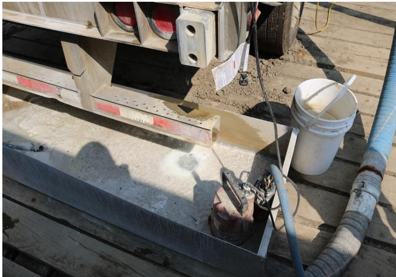
Figure 10 Water stored in lined cell to go through reverse osmosis
