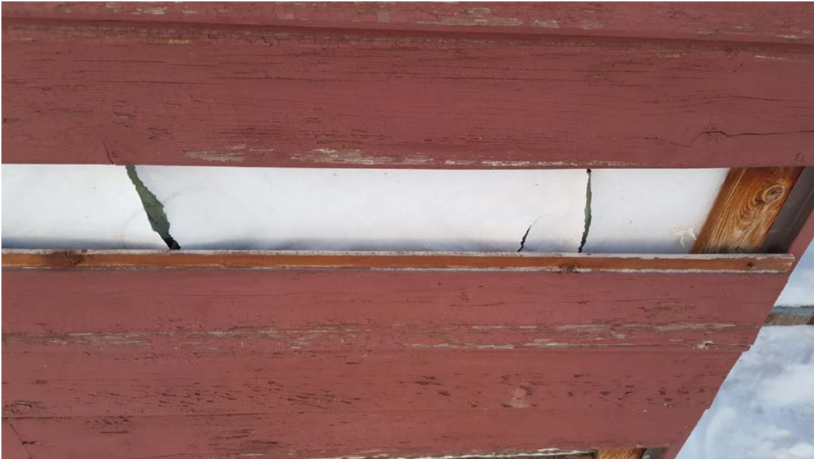
Photo 12: Exterior siding missing
