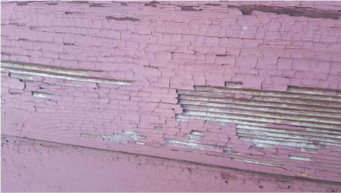
Photo 11: Exterior paint peeling
