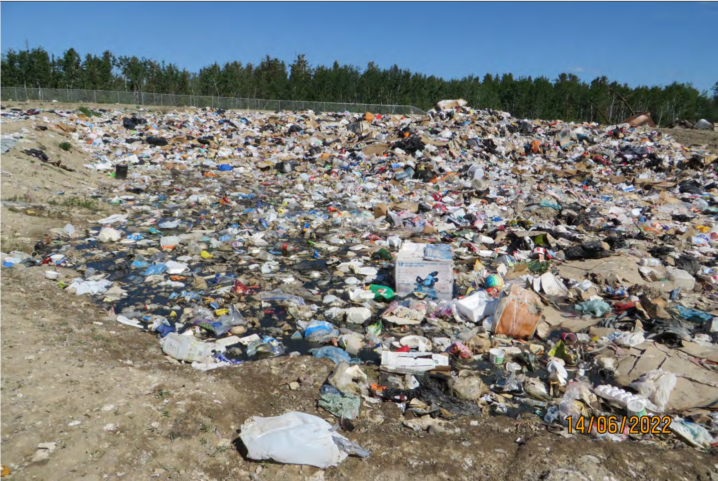
Figure 14 Landfill – Current domestic waste cell being used and leachate clearly visible
