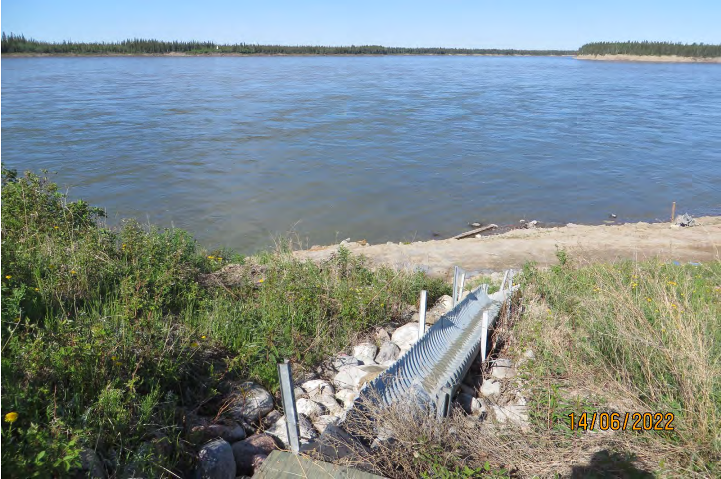
Figure 4 Water Treatment Plant (WTP) – Backwash discharge pipe
