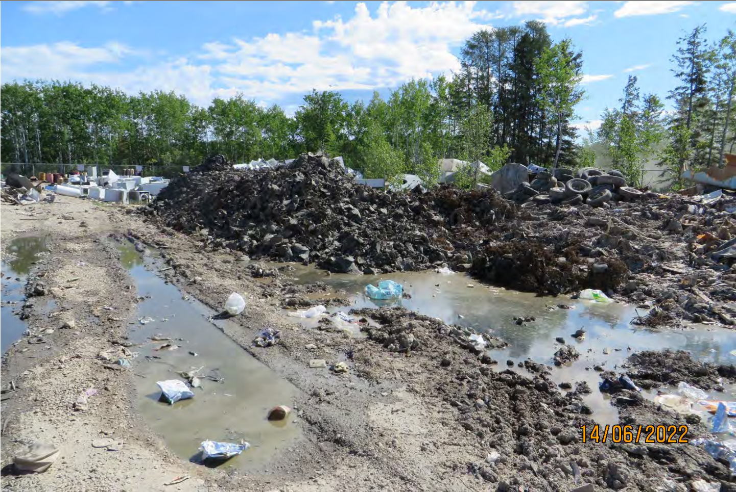
Figure 14 Landfill – Current domestic waste cell being used and leachate clearly visible
