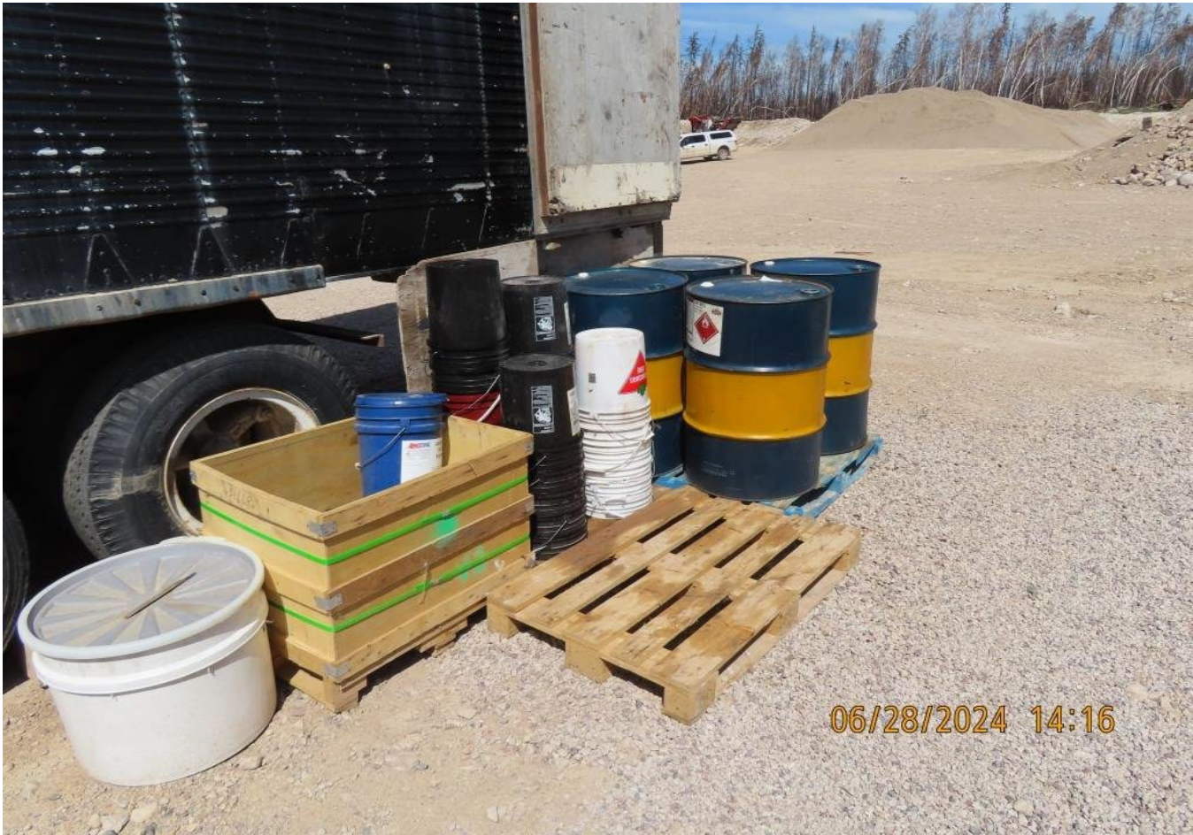
Figure 12 Fuel and chemical storage with spill kits.
