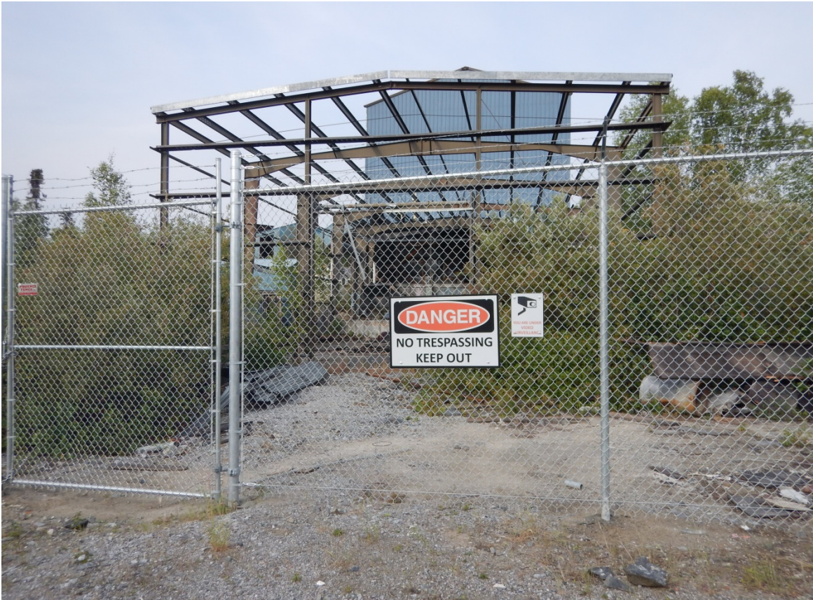
Figure 11 - Fence installation at Ptarmigan Mine
