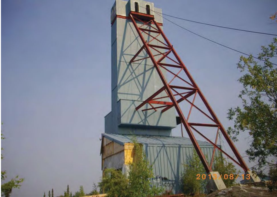
Figure 4 – Ptarmigan Mine headframe
