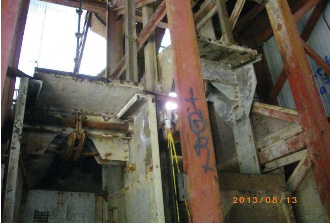
Figure 5 – Ptarmigan mineshaft elevators
