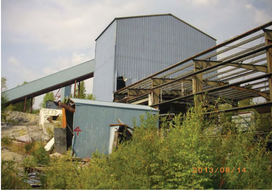
Figure 6 – Ptarmigan Mine mill building and gallery
