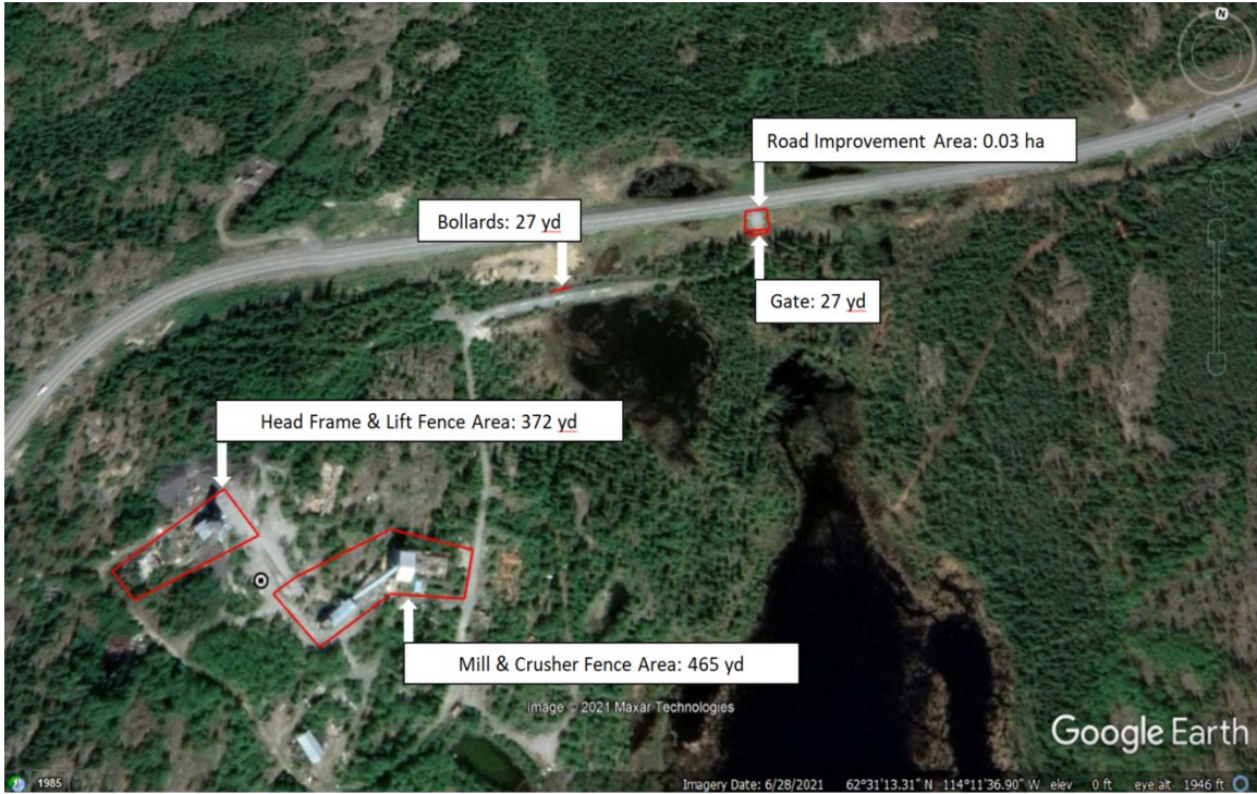
Figure 2 – The Ptarmigan Mine safety fence alignment and road improvements (red lines)
