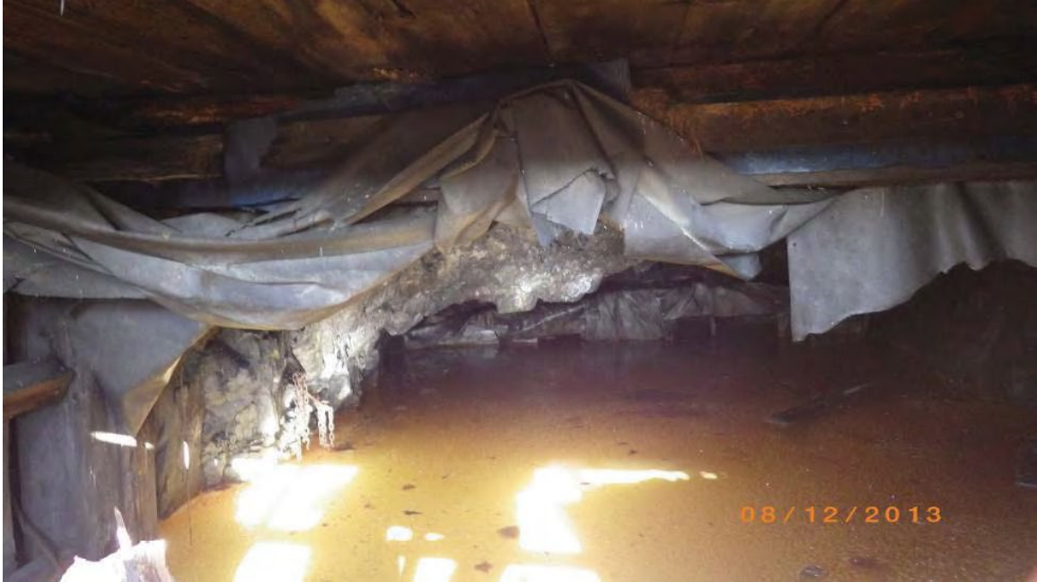
Figure 10 - Tom Mine flooded decline portal
