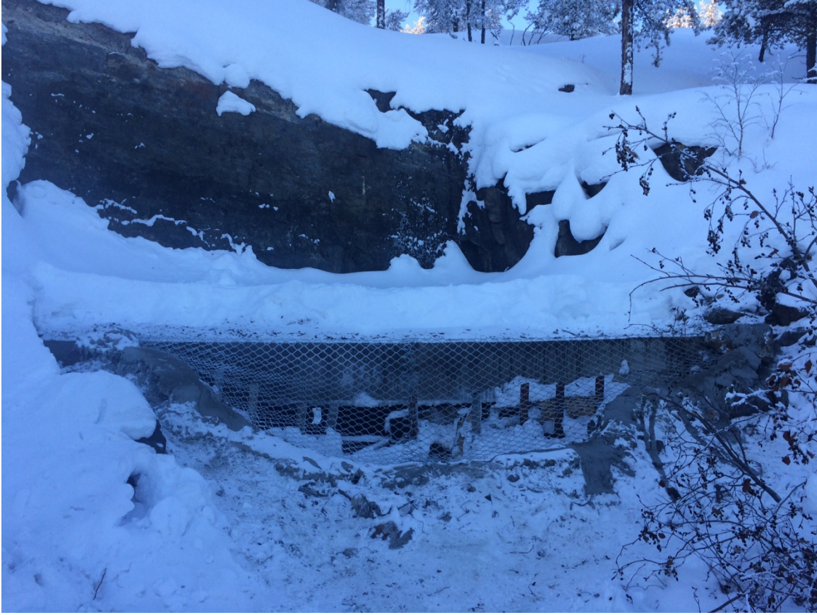
Figure 12 - Grouted wire mesh fence over mine opening at Tom Mine
