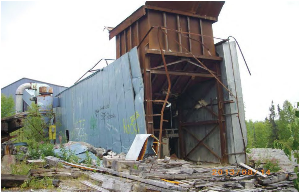
Figure 7 – Ptarmigan Mine crusher plant building
