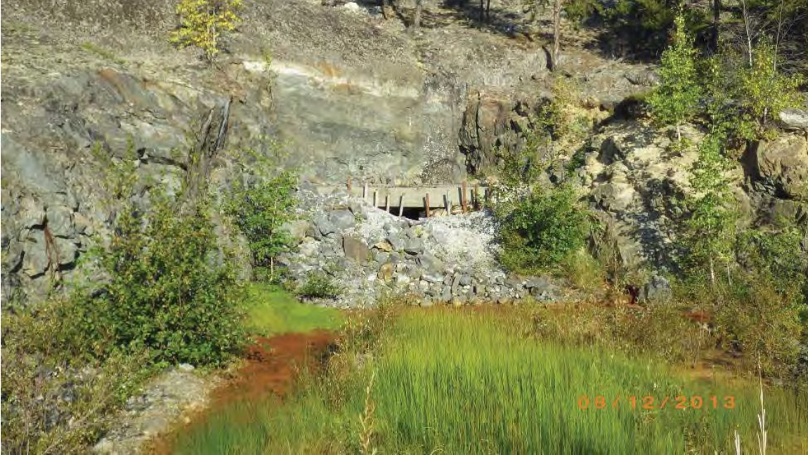
Figure 8 – Tom Mine decline portal
