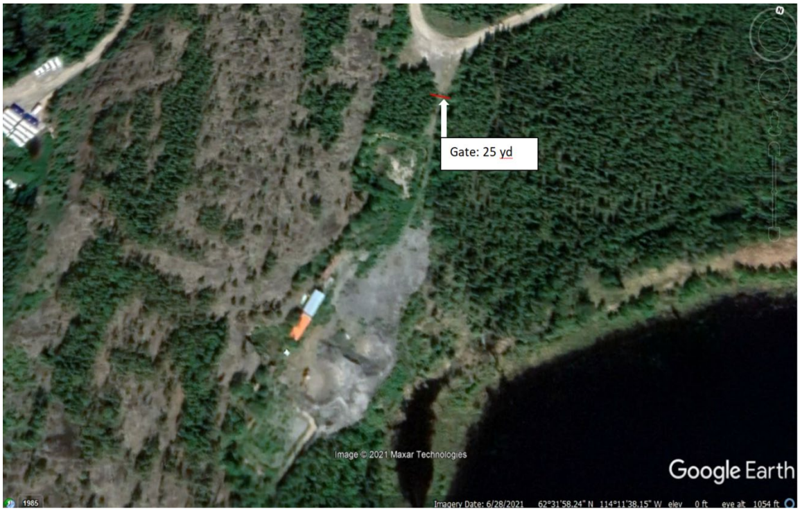
Figure 3 – Tom Mine safety fence and gate (red lines)
