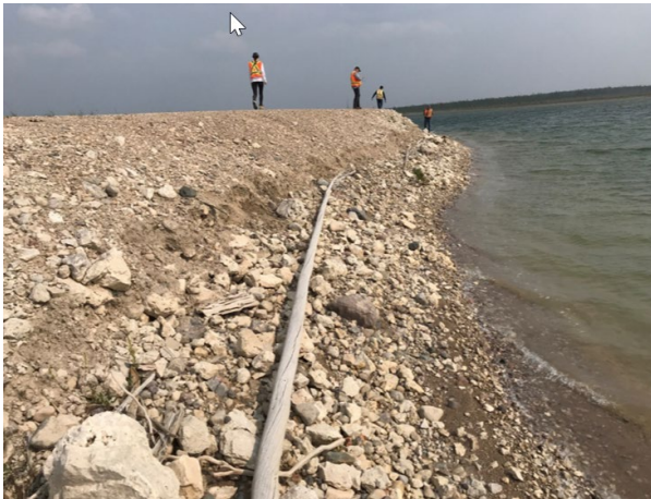
Photograph 1 – North Dyke – looking east, slumping and erosion on upstream slope
