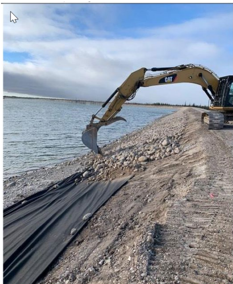
Photograph 3 – Placing riprap on North Dyke
