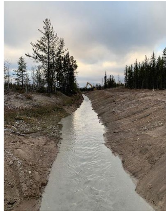
Photograph 5 – East Diversion Ditch grading
