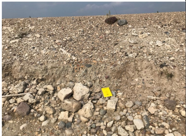
Photograph 2 – North Dyke – looking east, slumping and erosion on upstream slope
