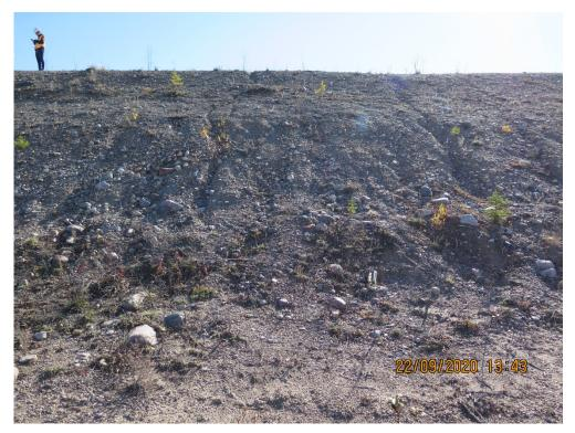
Photograph 16: North Dyke – Central Portion - Downstream Slope with Erosion Rills, Looking South, 22 September 2020
