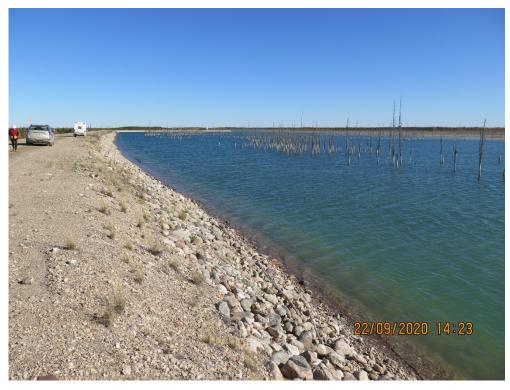
Photograph 17: North Dyke – Upstream Slope, Repaired with Riprap, Looking East, 22 September 2020
