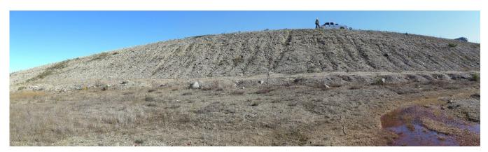
Photograph 11: West Dyke – North End - Downstream Slope with Erosion Rills, Looking East, 22 September 2020
