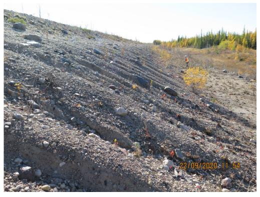
Photograph 9: West Dyke – Central Area - Downstream Slope with Erosion Rills, Looking South 22 September 2020
