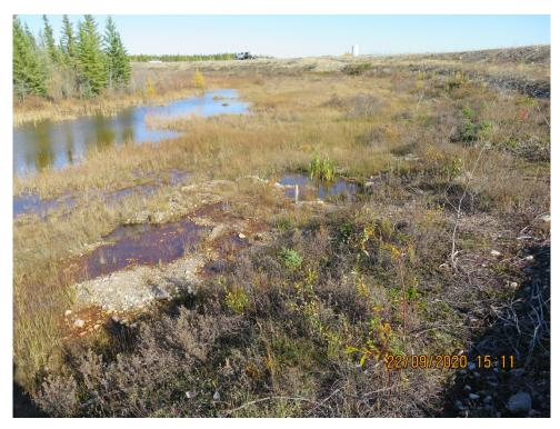
Photograph 20: North Dyke – Downstream Toe Area at Dogleg, Seep and Red Staining, Looking East, 22 September 2020
