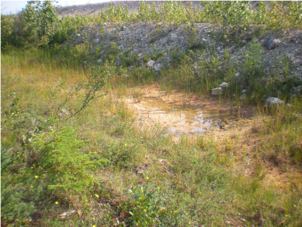
Photograph 5: West Dyke, South End. Ponded Water Downstream Of Toe, Looking North. 27 July 2017
