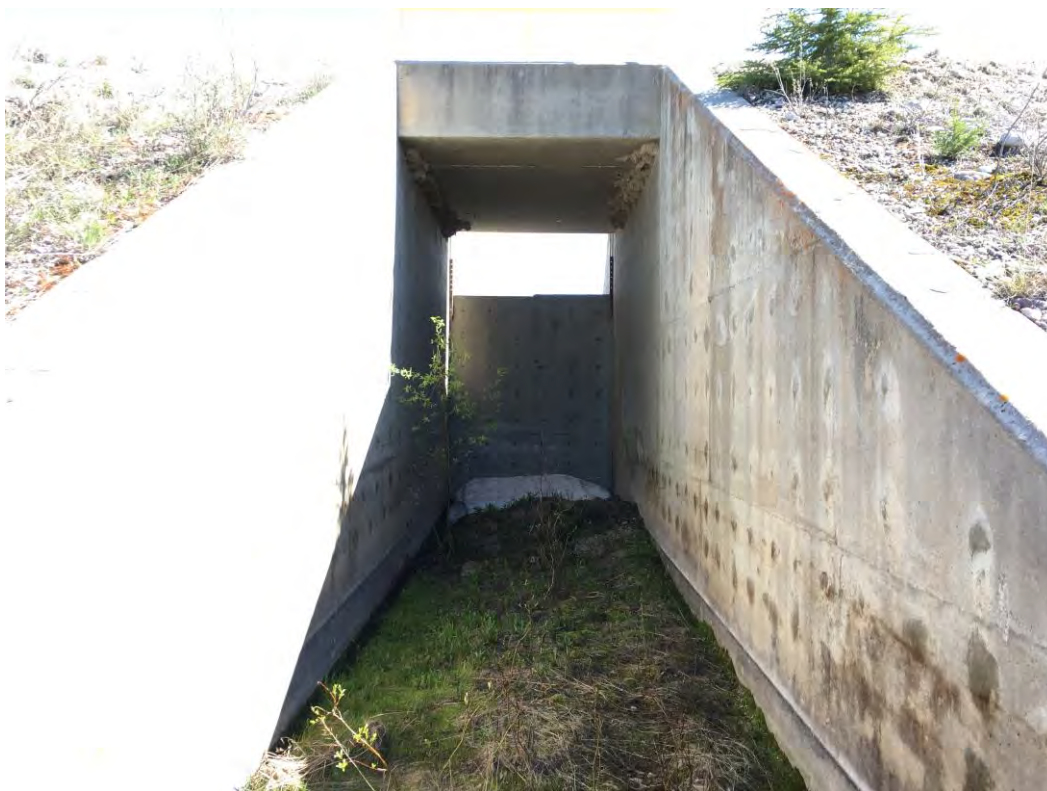
Downstream side of main pond spillway
