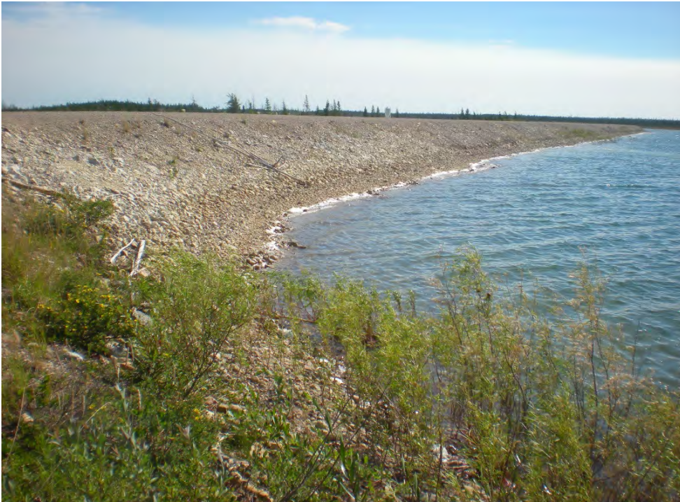
Photograph 10b: North Dyke Upstream Face, Gravel and Cobbles at Pond Waterline, at Dogleg Looking East. 27 July 2017
