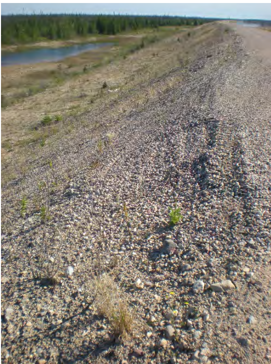
Photograph 8: North Dyke – Downstream Slope (left side of photo) with 2016 Patch on Erosion Feature in Place, Looking East. 27 July 2017
