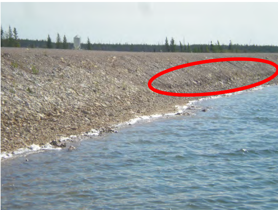
Photograph 10c: North Dyke Upstream Face, Gravel and Cobbles at Pond Waterline, at Dogleg Looking East. Detail Showing Possible Sloughing of Previous Repair. 27 July 2017
