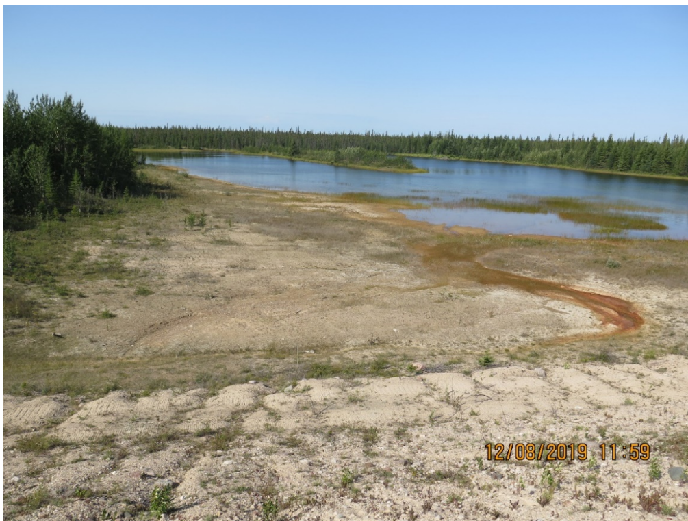
Photograph 6: West Dyke – Downstream Toe Area with Staining Along Drainage Near Former Seep Location, North End, Looking West, 12 August 2019
