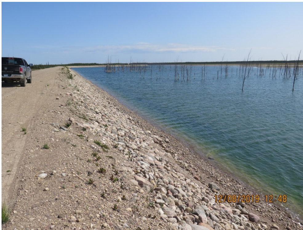
Photograph 11: North Dyke – Upstream Slope, Repaired with Riprap, Looking Northeast, 12 August 2019
