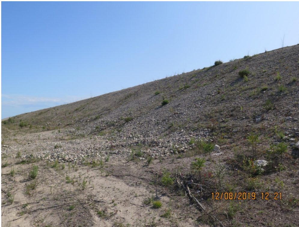
Photograph 9: North Dyke – Repaired Erosion Rills on Downstream Slope Near West End, Looking Southeast, 12 August 2019
