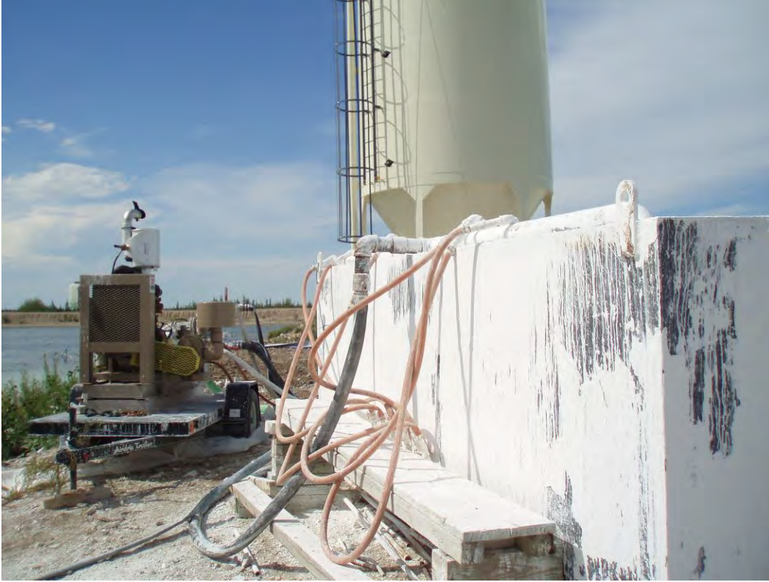
Lime Slurry Tank: New discharge header and air lines to the lances
