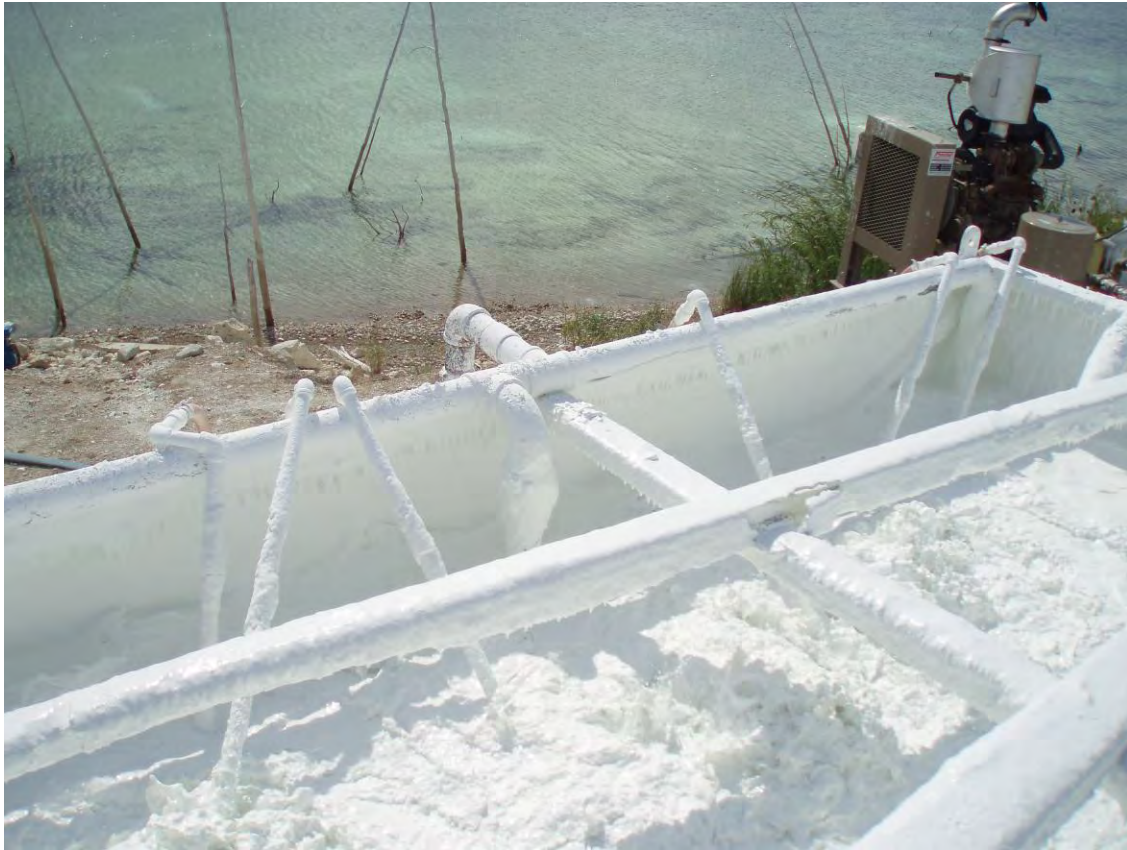
Lime Slurry Tank: New 2007 discharge header and air lances
