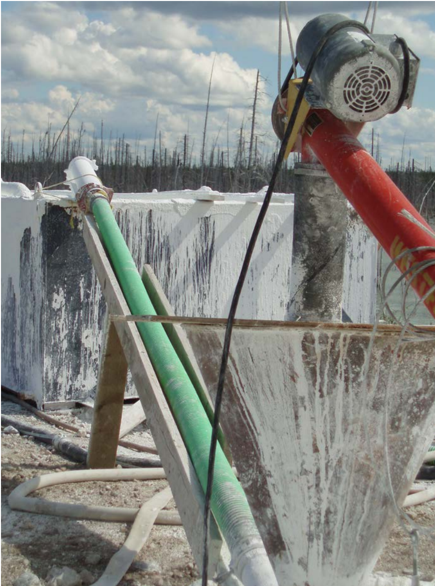
Lime Slurry Tank: Discharge Line from Jet Mixer and Suction Line to the Lime Pump
