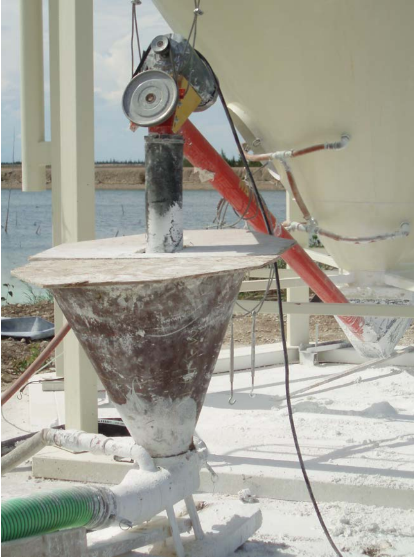
Lime Silo, Auger and Jet Mixer July 2007
