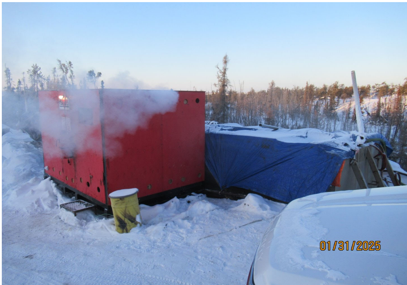
Figure 4 Coil stove in the red building is being used to heat the water in the settling tank.
