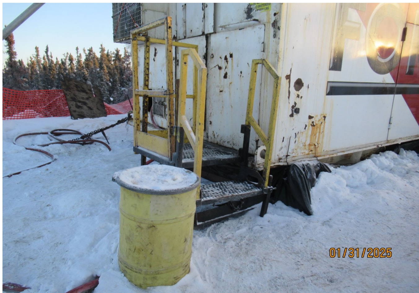
Figure 8 Spill kit located in a highly visible location at the second pump shack.
