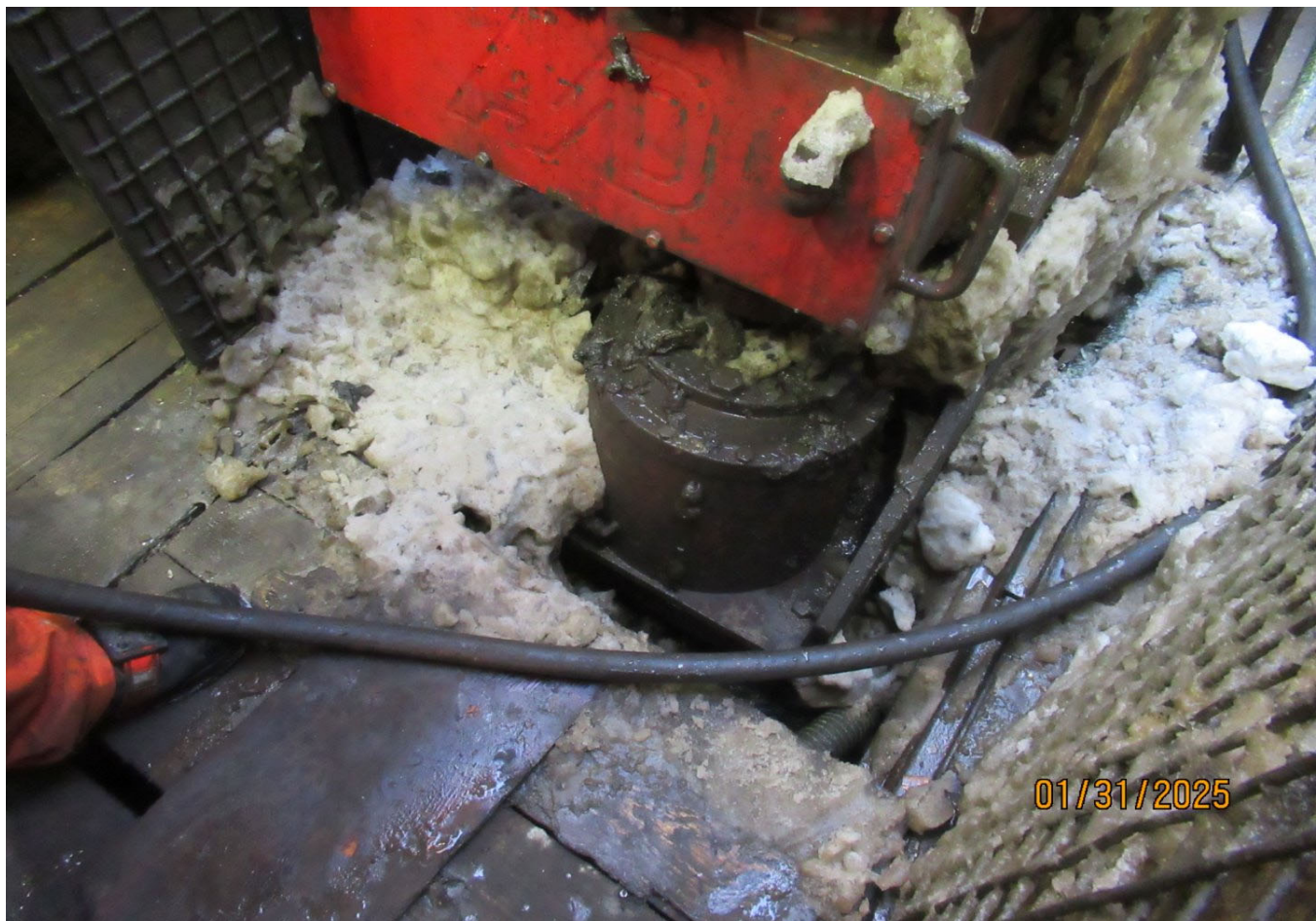
Figure 4 Coil stove in the red building is being used to heat the water in the settling tank.
