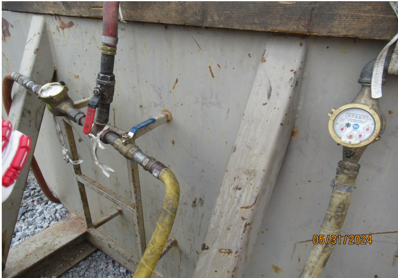
Figure 12 Water meters on the side of the settling tank.
