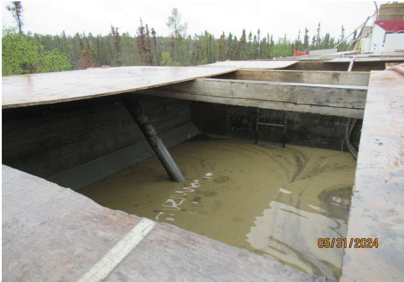
Figure 14 Cellar at the collar of the drill site for the collection of drill waste.
