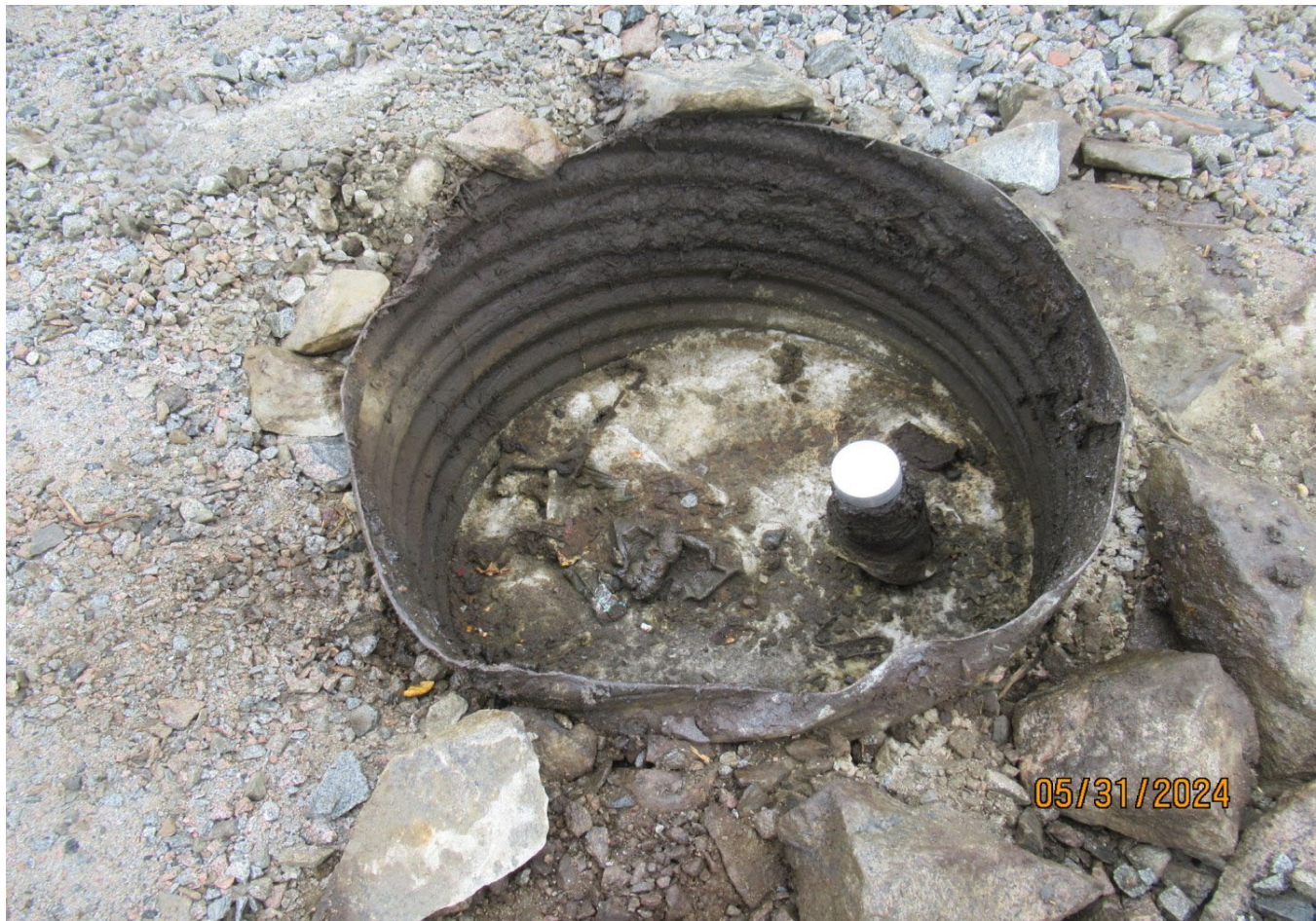
Figure 22 Cellar at the completed drill site. It will be removed once a final decision is made on the re-entry of this drill hole.
