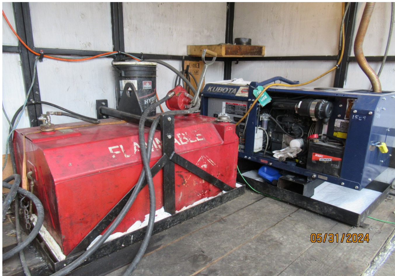
Figure 16 Secondary containment under other ancillary equipment in the land use area.
