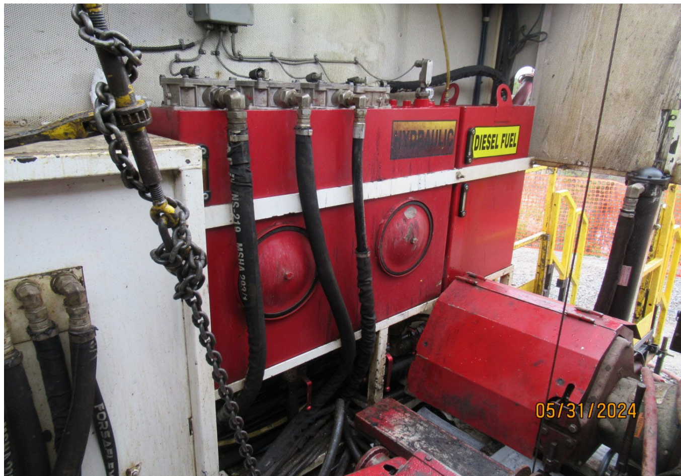
Figure 8 No obvious spills or concerns were noted with fuel handling at the generator or tidy tank inside the pump shack.
