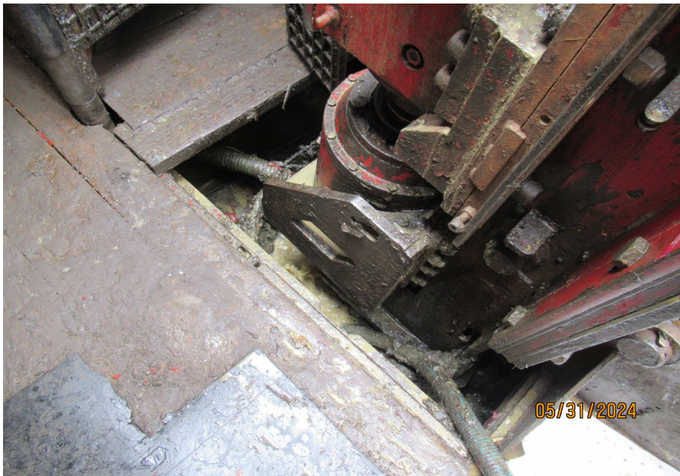
Figure 14 Cellar at the collar of the drill site for the collection of drill waste.
