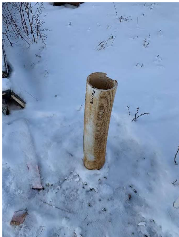
Photograph 2: PW-02 . No well cap. Hydrocarbon sheen observed during sampling and purging. Screen of the well extends above ground. Possible conduit to groundwater contamination. Needs inspection for possible decommission. Well sample collected. Photograph was taken on October 25, 2023.
