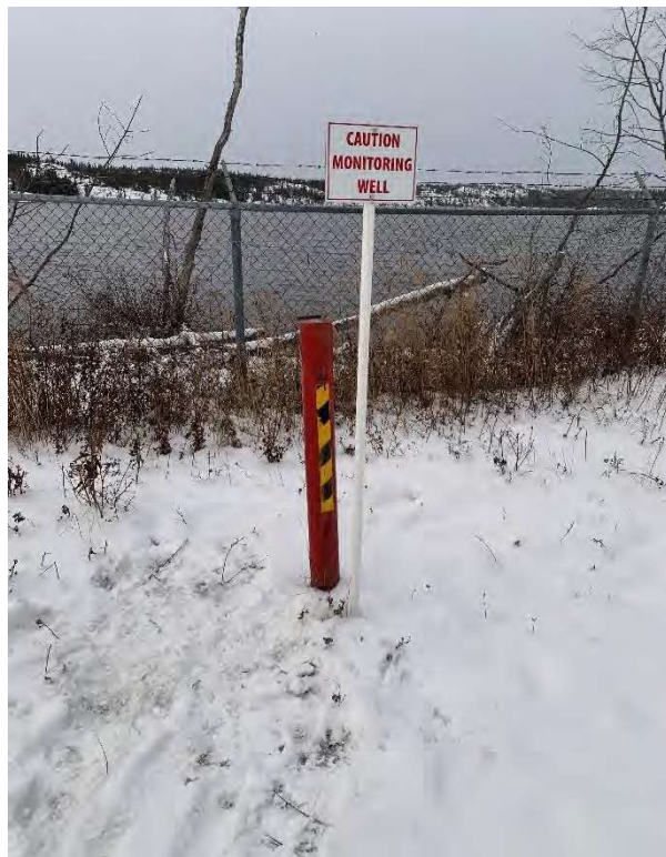
Photograph 7: JF01-04 . Appears to be in proper working condition. Silt observed at bottom of the well. Well sample collected. Photograph was taken October 25, 2023.
