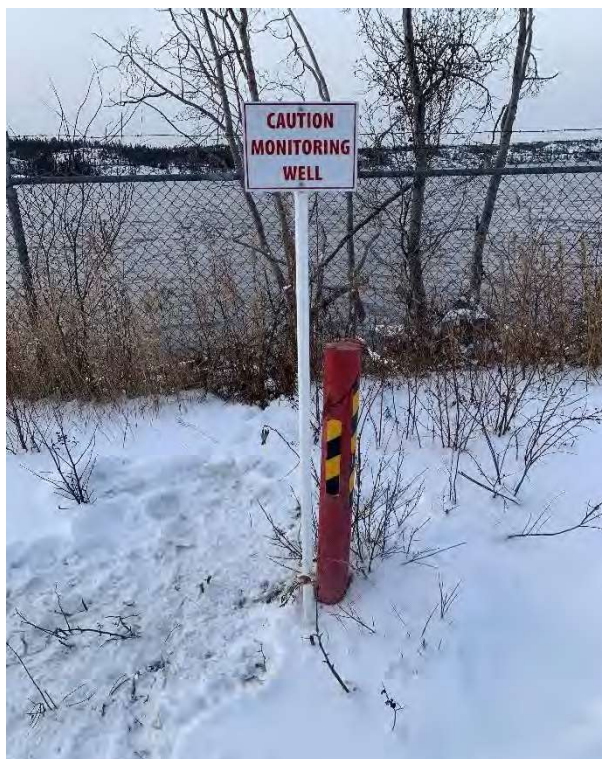
Photograph 9: JF01-06 . Appears to be in proper working condition. Silt observed at the bottom of the well. Well sample collected. Photograph was taken October 25, 2023.
