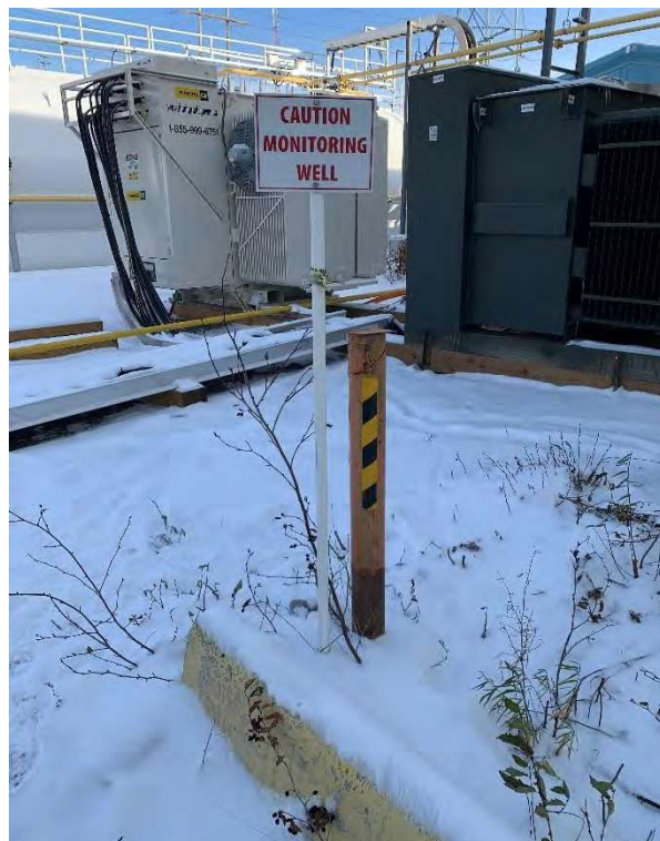
Photograph 14: MW-05 . Appears to be in proper working condition. Hydrocarbon sheen observed during purging and sampling. Well sample collected. Photograph taken on October 25, 2023.
