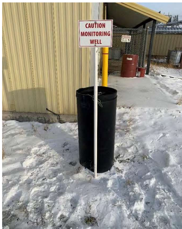
Photograph 3: PW-03 . No well cap. Debris observed in the well. Insufficient water for sample. Photograph was taken October 25, 2023.
