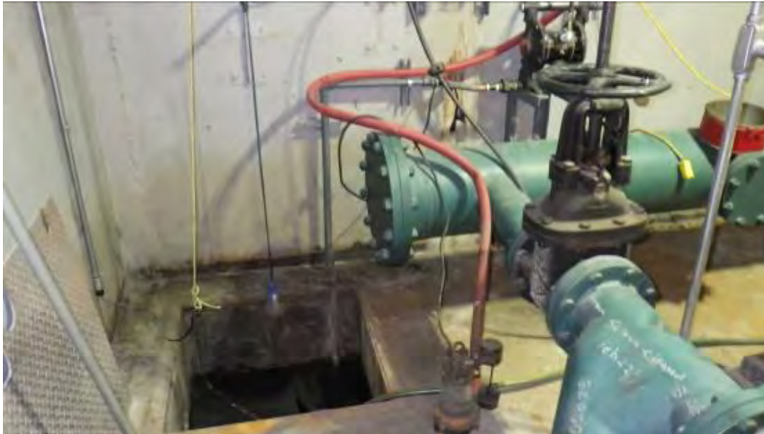
Photo 7: EMD Plant Sump
