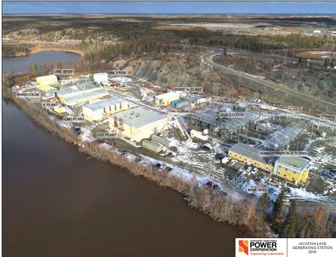
Figure 3: Jackfish Diesel Generating Facility
