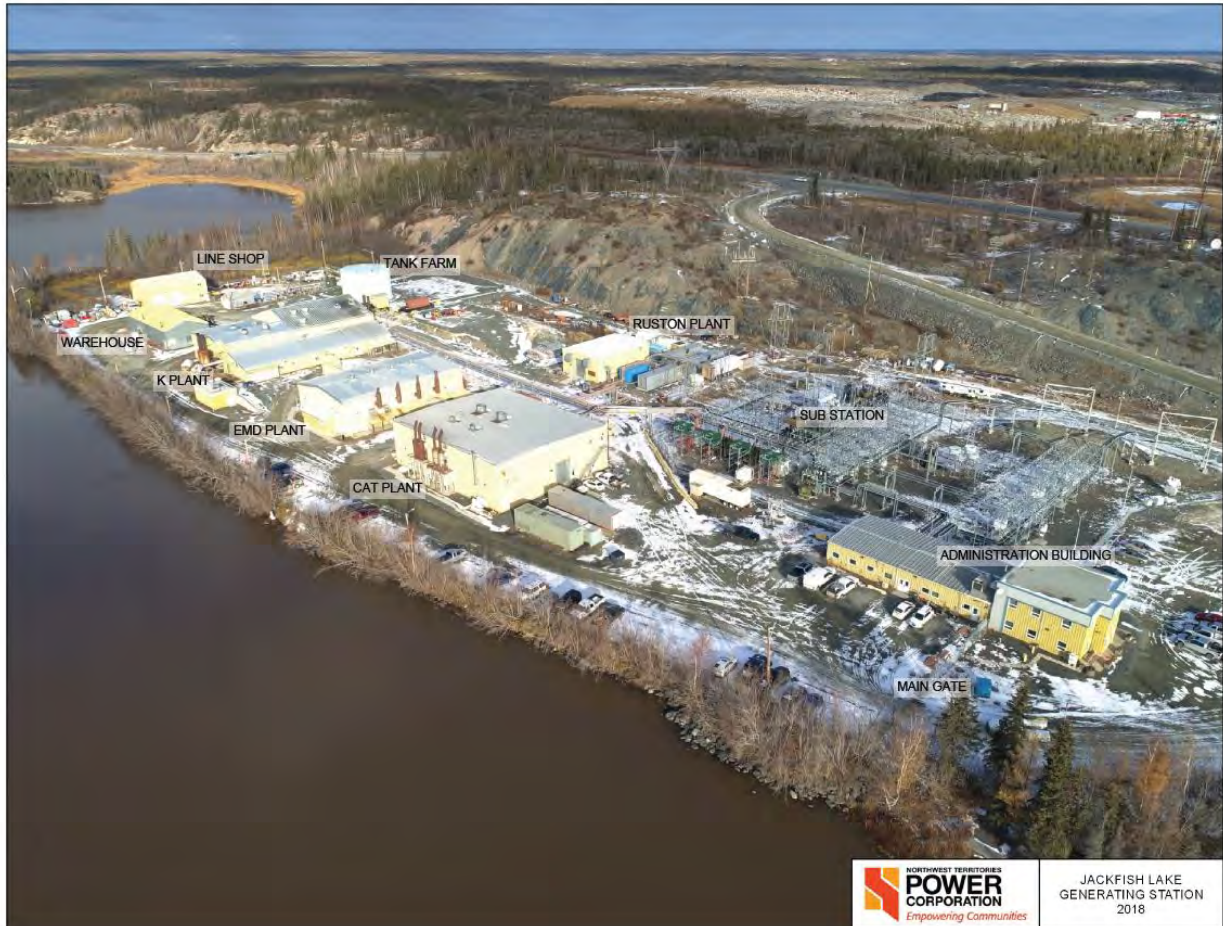
Figure 1: Jackfish Lake Generating Station
