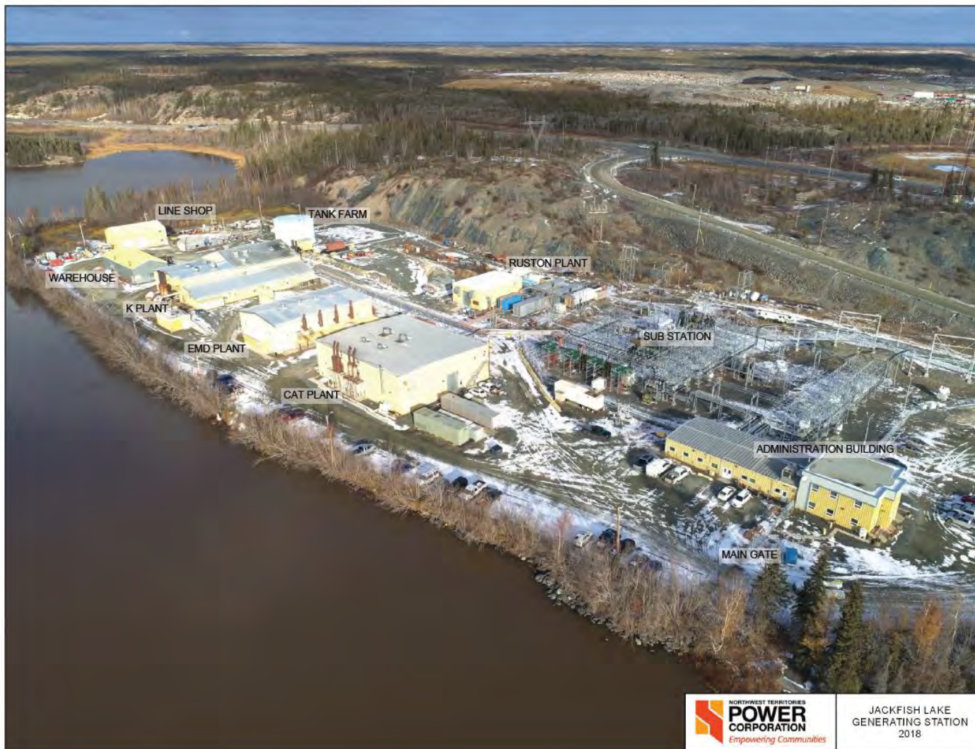
Figure 3: Jackfish Lake Generating Station
