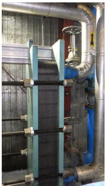
Photo 6: K-Plant Plate Heat Exchanger
