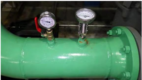
Photo 8: Raw Water Pressure and Temperature Gauges
