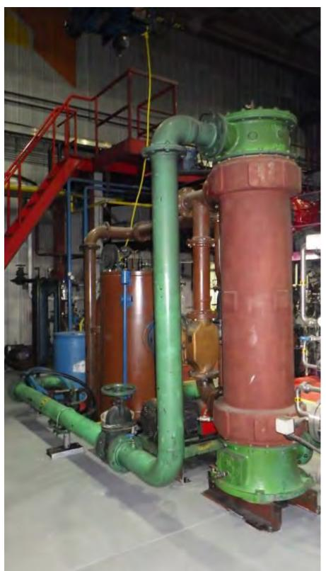
Photo 3: K-Plant Sheet and Tube Oil Heat Exchanger
