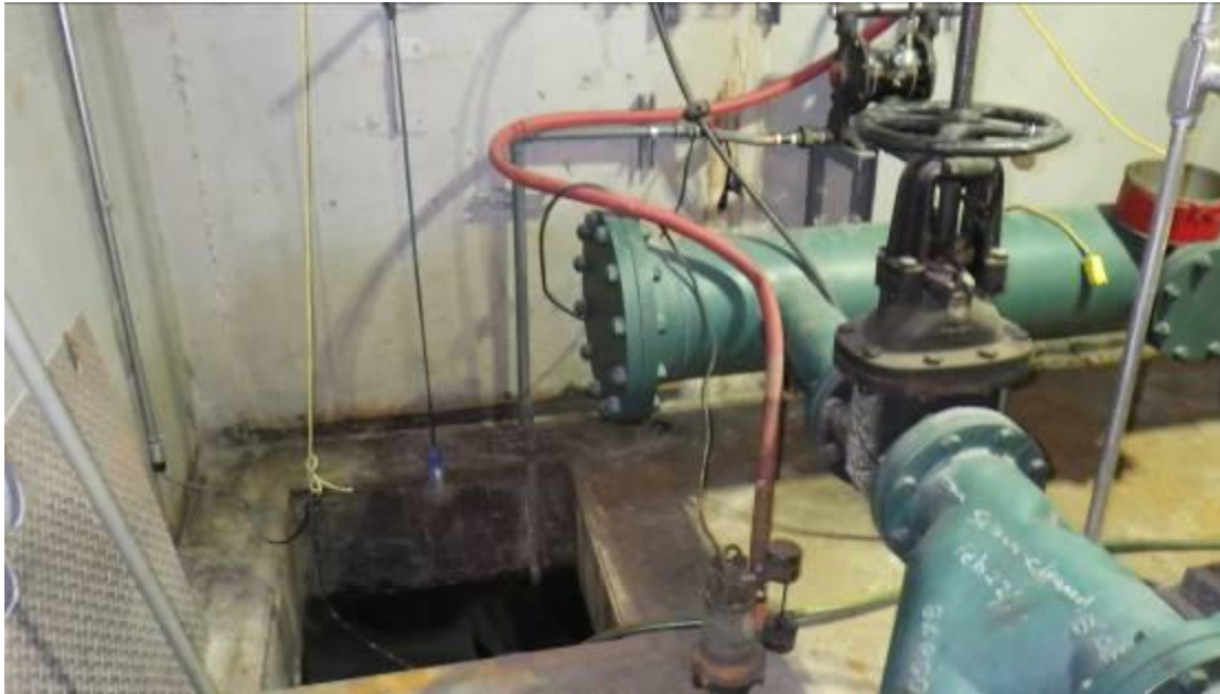
Photo 7: EMD Plant Sump
