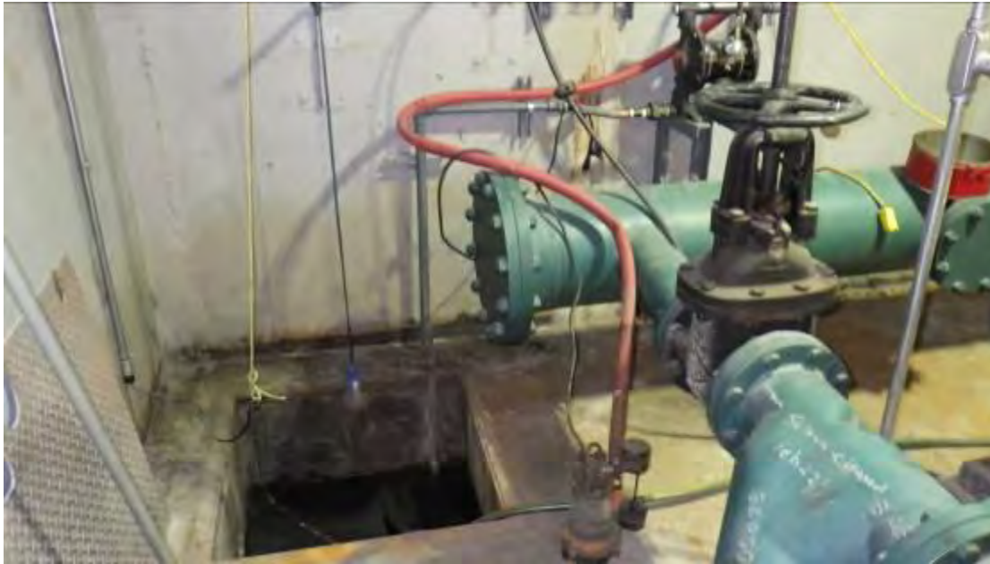
Photo 7: EMD Plant Sump
