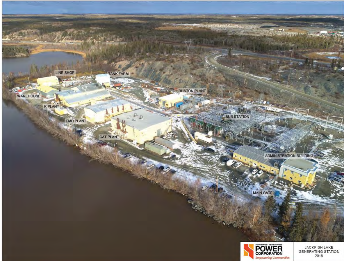
Figure 3: Jackfish Diesel Generating Facility
