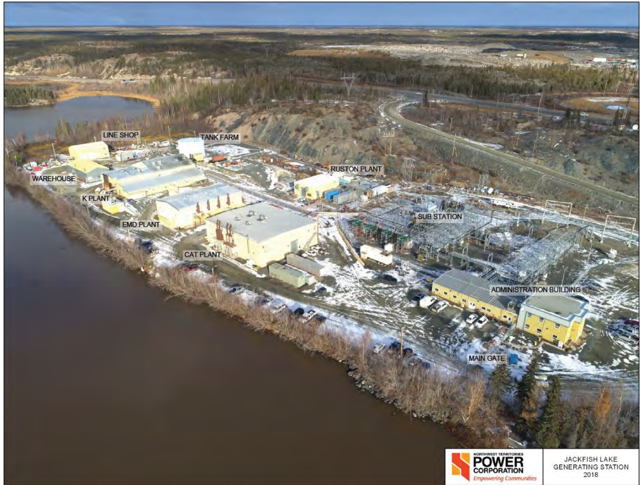
Figure 2-1: Jackfish Lake Generating Facility
