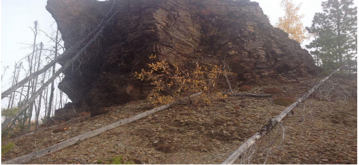
Figure 31: The fragmented shale rock knob the road passes thru at km 55.3.
