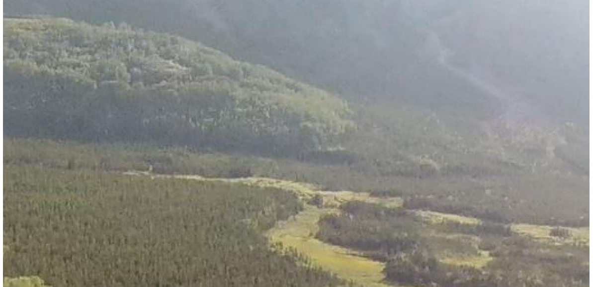
Figure 67. The noticeable elevated knob/ridge should provide suitable subgrade borrow. The proposed ASR alignment is located at the lower base of the slope.
