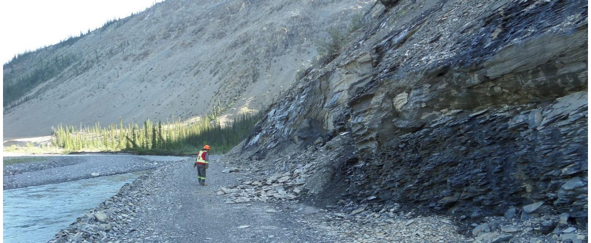
Figure 4: The rockfall hazard at 4.01 km may generate a large quantity of waste rock that could be used to supply subgrade borrow needs elsewhere nearby.
