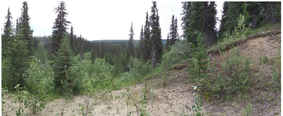
Figure 17: View of the existing cut for the past winter road across the end of the esker at 42.6 km.
