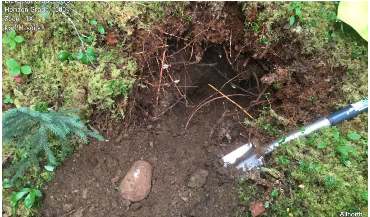
Figure 66. A shovel test of material near BP 110 indicates excellent material for overland subgrade material.
