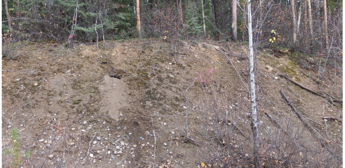
Figure 51: Existing cut slope exposing the BP86A sand material. Large timber growing on the site indicates the area is likely permafrost free.
