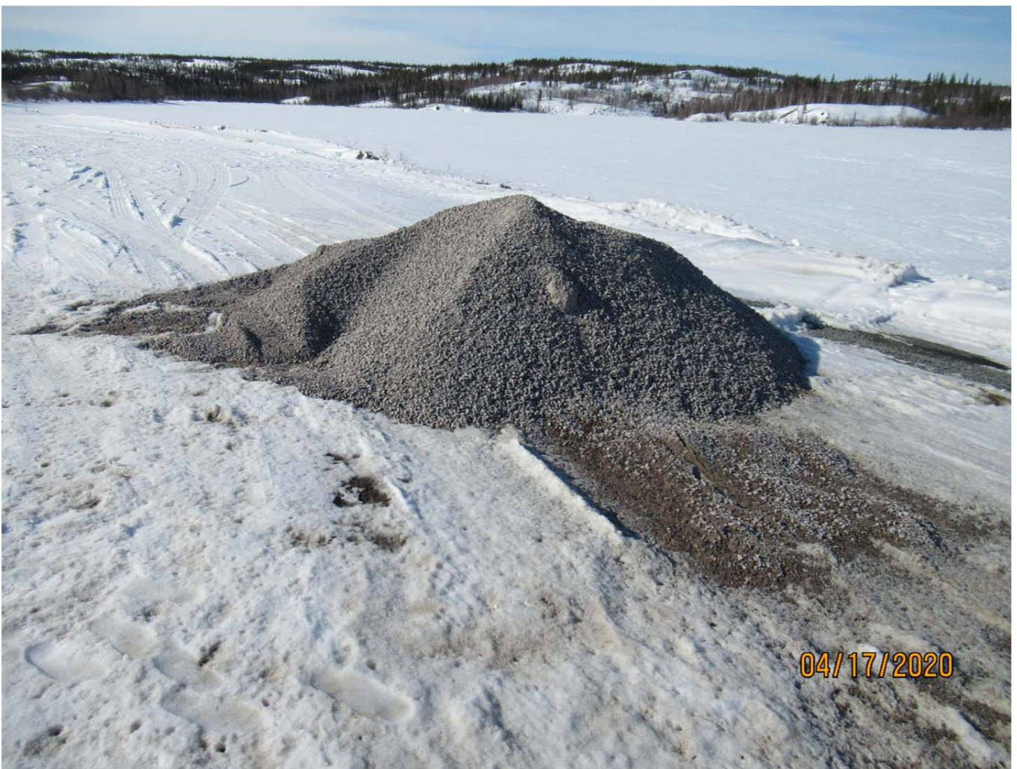
Photo #4 - MV2019X0008 - GNWT-ITI - Prosperous Lake Territorial Park A stockpile of 20 mm blend remains on site.
