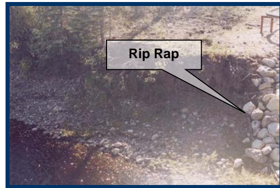
Riprap helps to stabilize stream banks.
