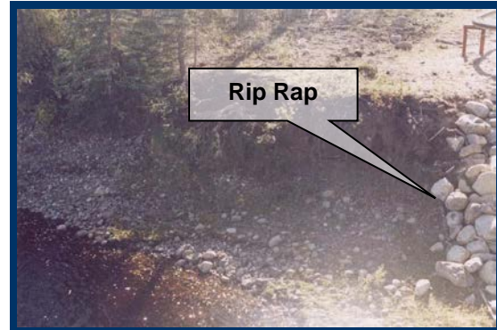
Riprap helps to stabilize stream banks.
