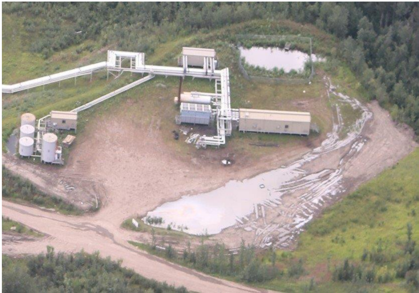
Figure 8 F-25/F-25A- note sump overflowing
