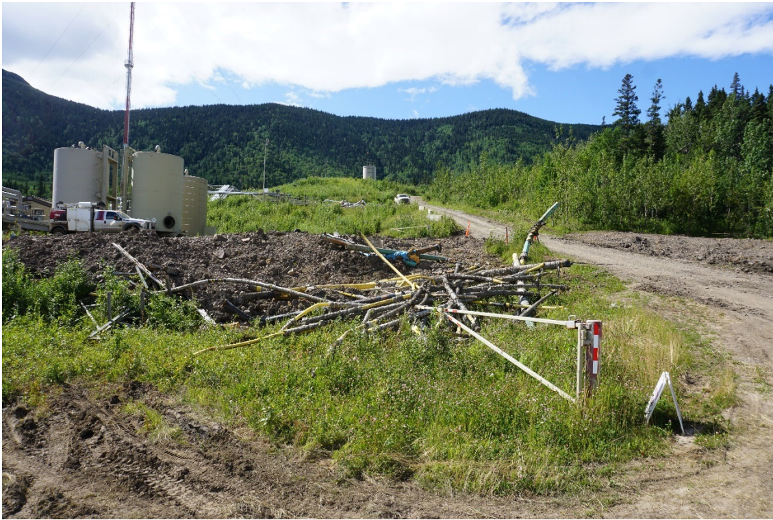
Photo #11: Waterline was removed from the ground and staged at the F-25 site.
