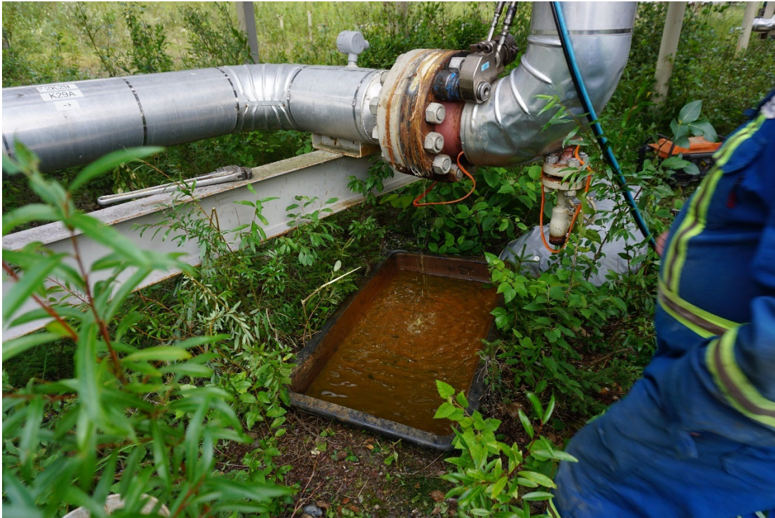
Photo #4: Drip trays were present underneath disconnected lines to prevent impacts to the underlying soils.
