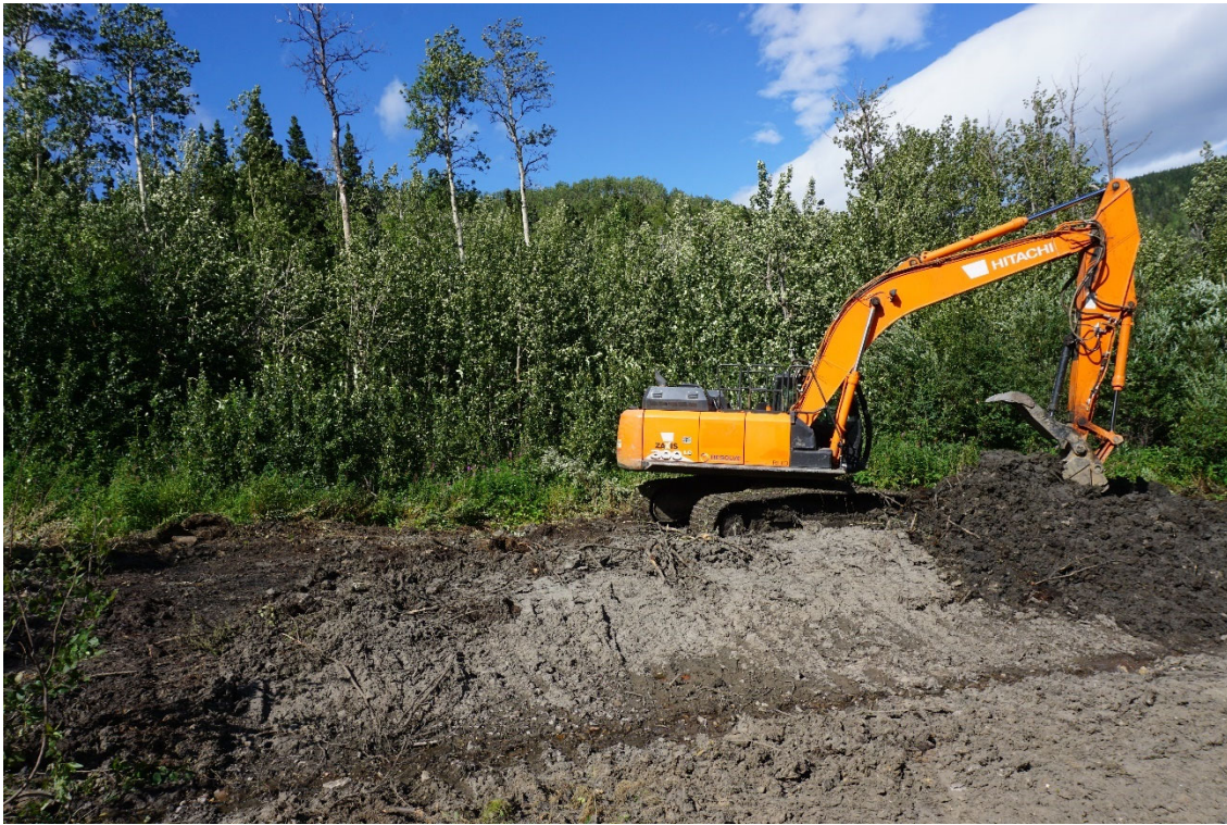
Photo #13: The areas under the waterline extraction points were re-contoured.
