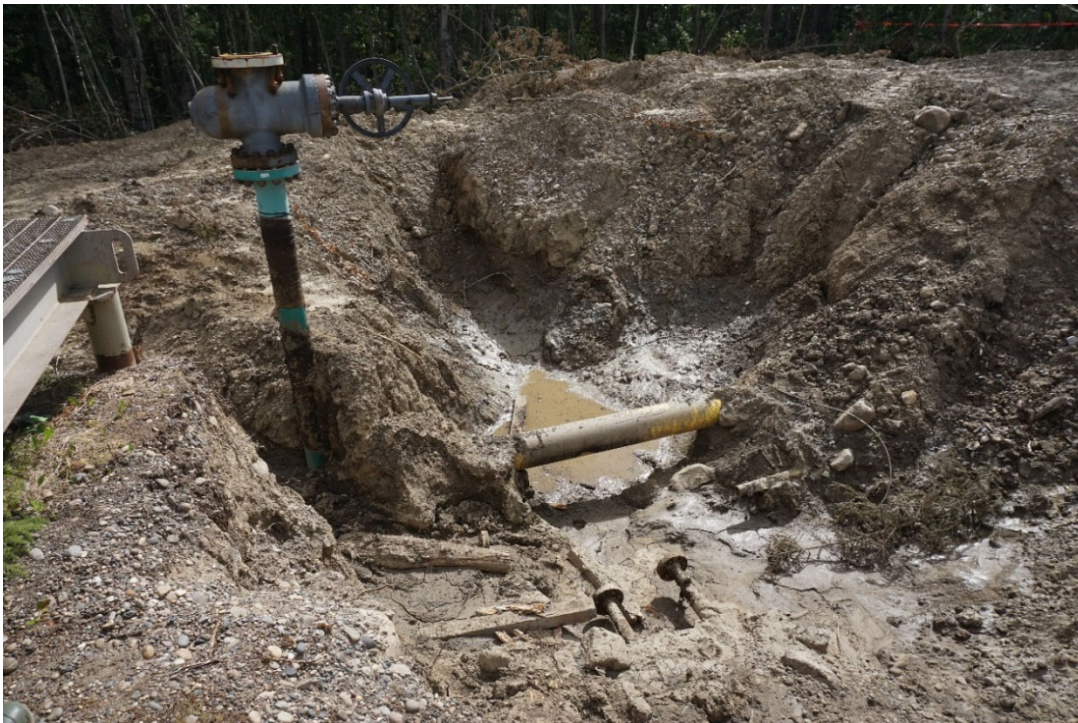
Photo #8: Waterlines at the junction that leads to the O-80 Injection well. And Pipelines from the Liard West field that lead to the South Pointed Mountain pig receiver. This hole will be refilled and mounded to prevent the ponding of water.
