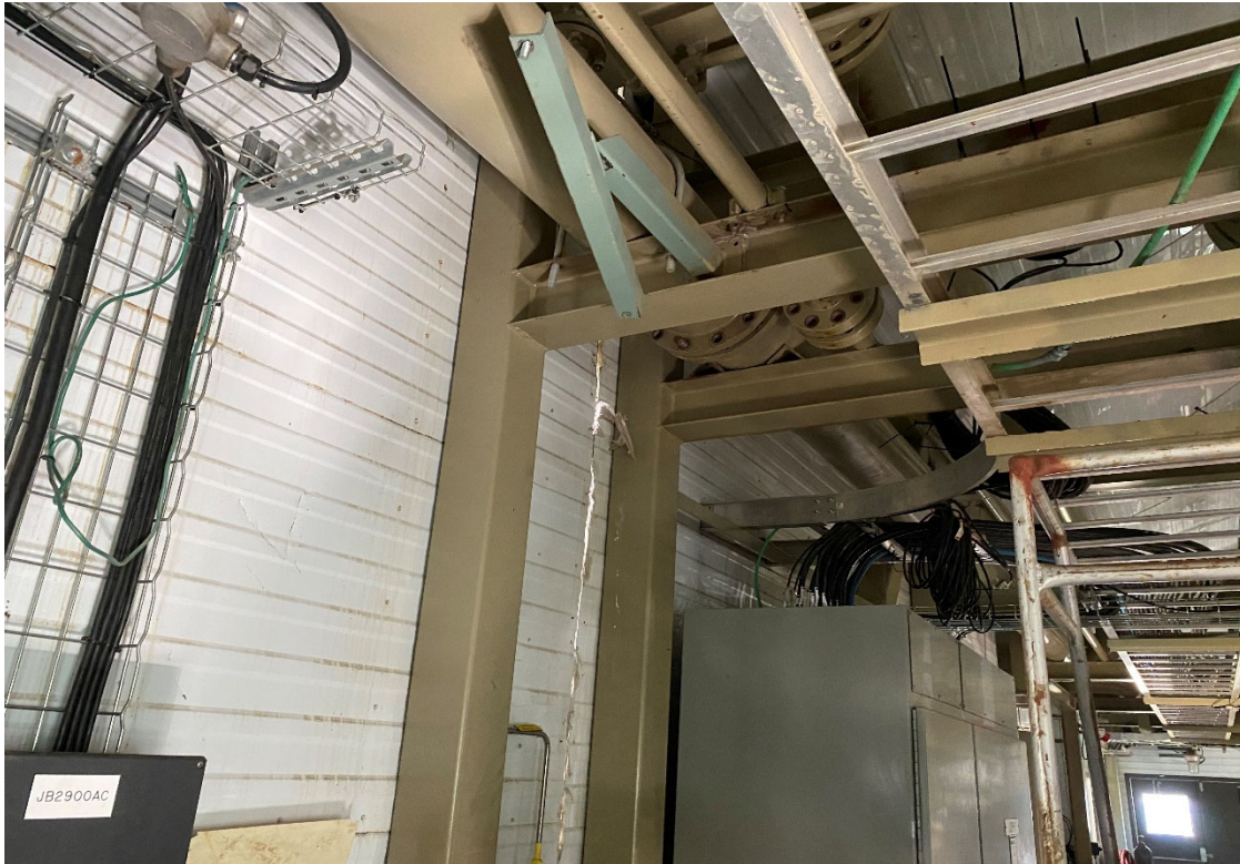
Photo #6: Electrical lines are disconnected and wrapped neatly inside the buildings.
