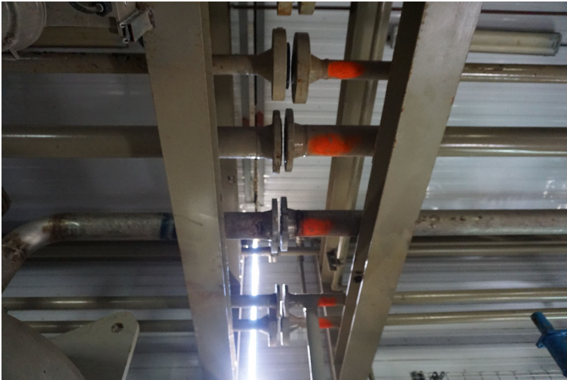
Photo #1: Pipelines inside buildings have been disconnected along with the walls and floor of the building.
