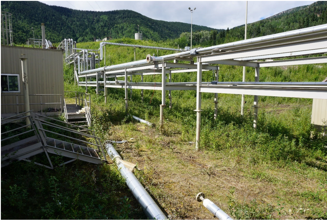
Photo #5: Above ground lines at the F-25 site have been disconnected from the separator buildings.
