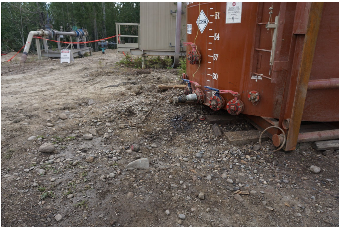
Photo #18: Vertical tank containing water and hydrocarbons from pigging operations was overtopped and hydrocarbons have impacted the underlying soils. This concern was discussed on site and contaminated soils will be excavated, containerized, and removed for proper offsite disposal prior to the end of operations.
