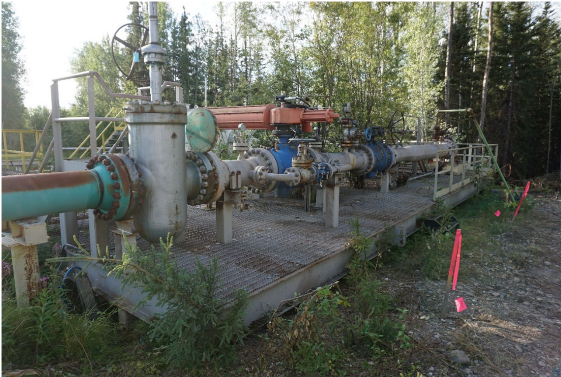
Photo #9: View of the South Pointed Mountain pig receiver. The pipeline from the Liard West Field ties into the South Pointed Mountain transboundary pipeline at this location.
