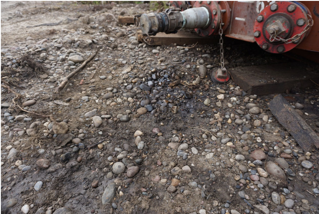
Photo #19: Drip trays must be utilized under all fluid transfer points to reduce the likelihood of hydrocarbon impacts to the underlying soils.
