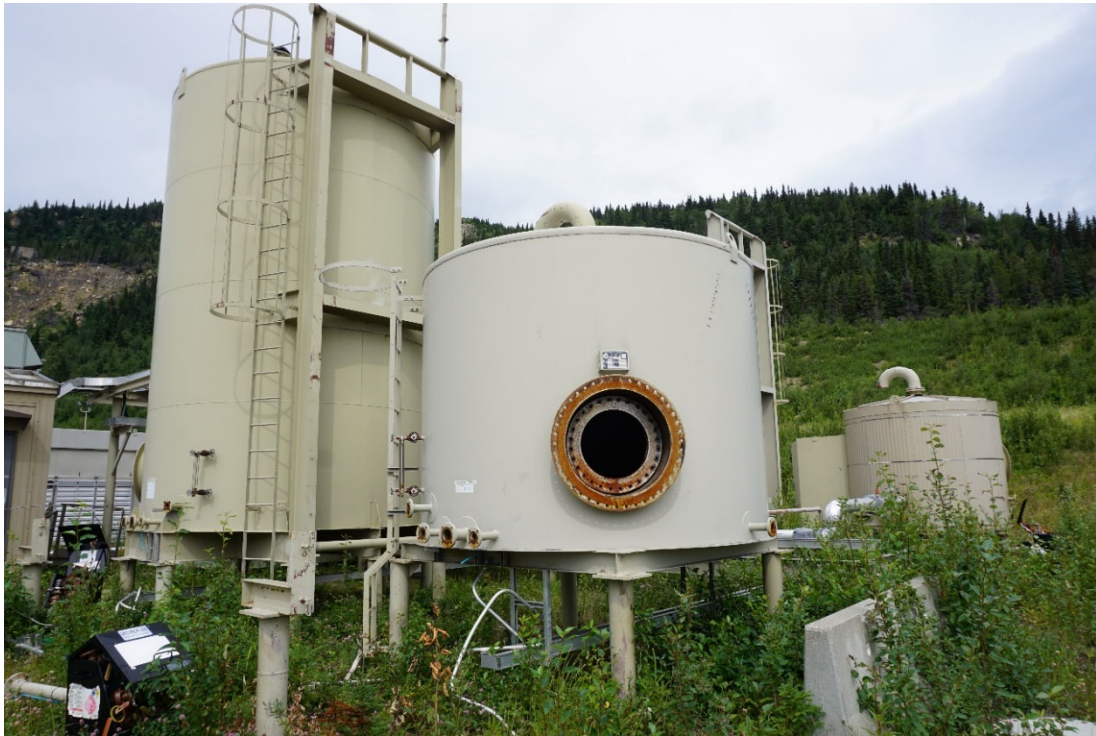
Photo #17: Vertical tanks containing Methanol, Diesel, etc have been emptied with a vac truck and access hatches opened to ensure all fluids have been removed.
