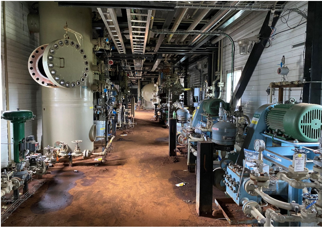
Photo #7: View of the inside of a purged and plugged building that has been disconnected from the outside above ground pipelines.
