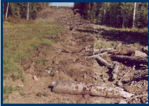
Rollback of wood slash over the trench line helps to stabilize the soil.
