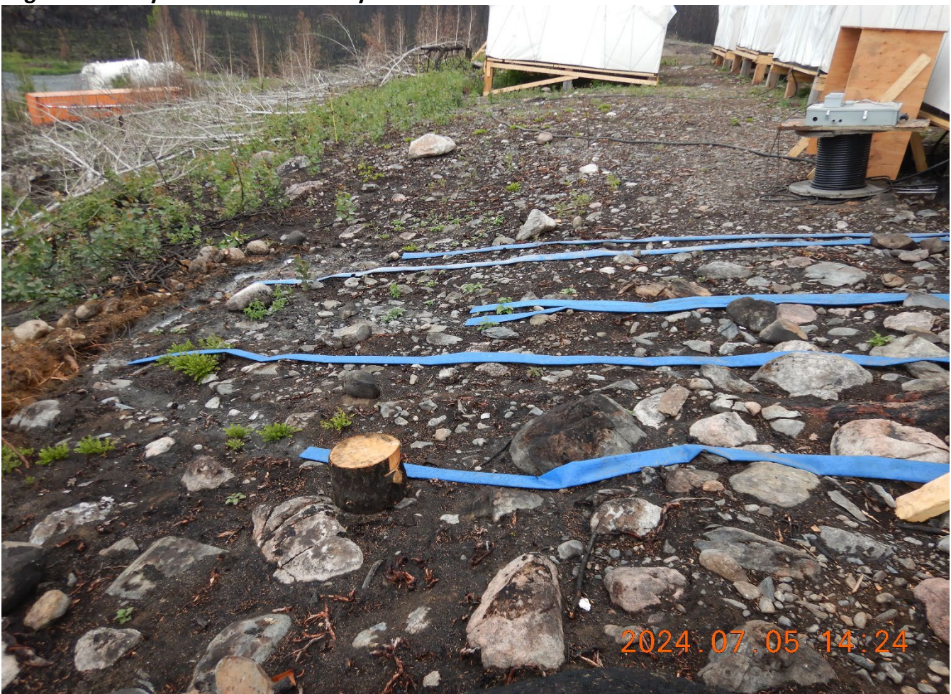
Figure 4 – Greywater lines from dry and kitchen.
