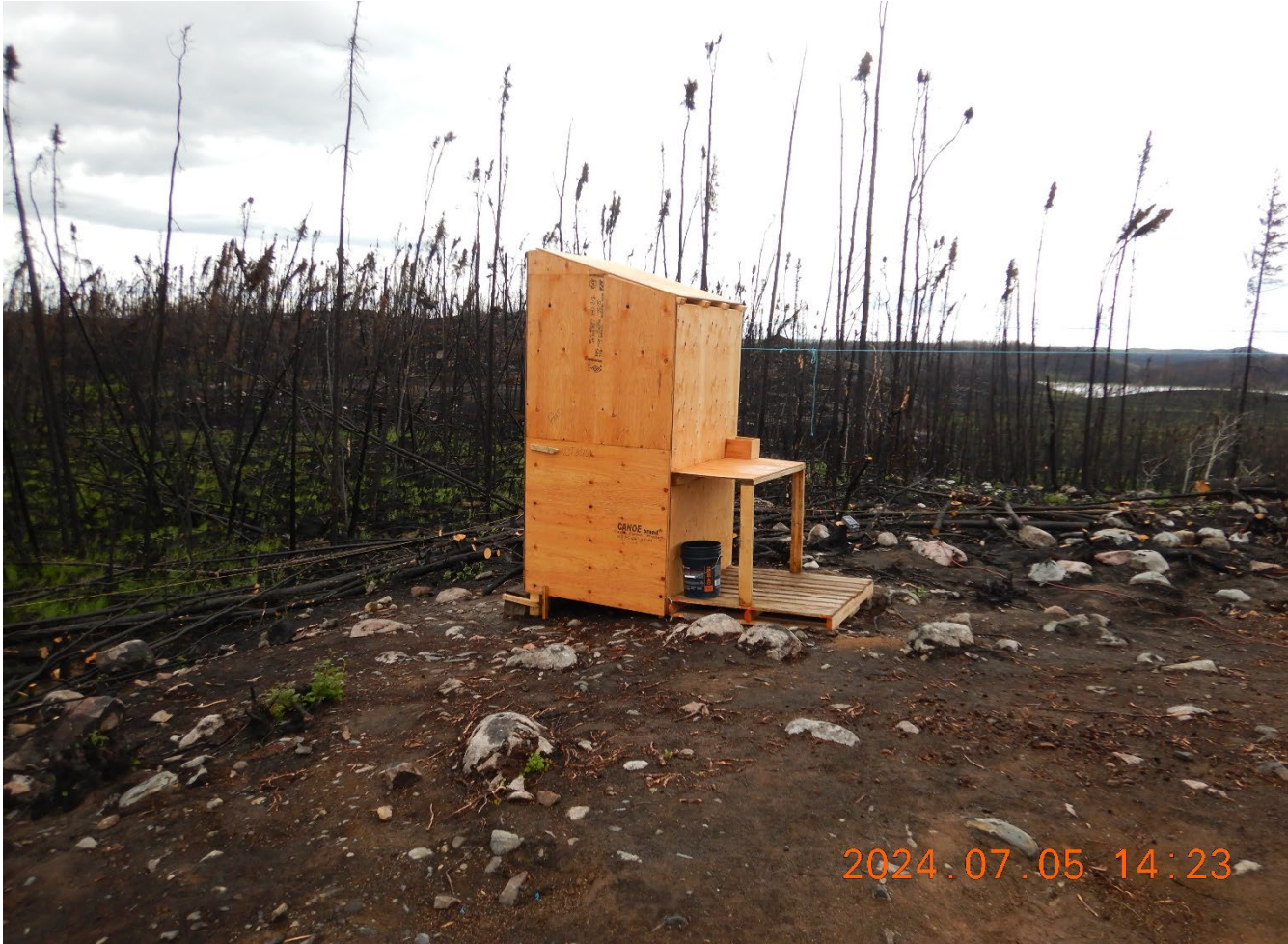
Figure 3 – Pit Privy for sewage disposal.
