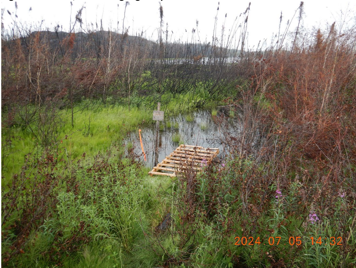
Figure 9 – SNP-9, Clearer signage required.
