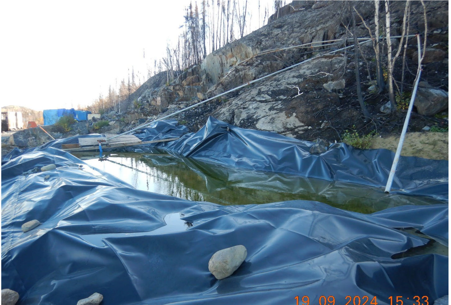
Figure 3 – Mine water settling pond.
