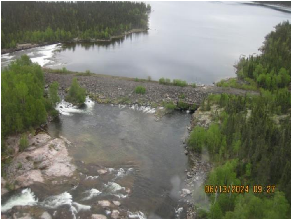
Photo 20. Shows the Nonacho Dam, Spillway & Control Structure with Ro-torque Operators (3). It is a rockfill dam designed to accommodate leakage. About 300mm of settlement of the crest occurred shortly after 1968 construction where leakage is high at the right abutment, and has remained stable since. Inspection reports over the years, based on visual assessments, have stated no change in condition. Pins have now been installed for survey and to verify the stability of the structure.
