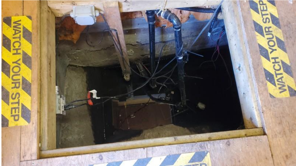
Photo 14. Shows the Well, right side, above Switchyard & Powerhouse. Stagnant water. No flow in drainpipe at the right side of the Powerhouse, where flow is measured.
