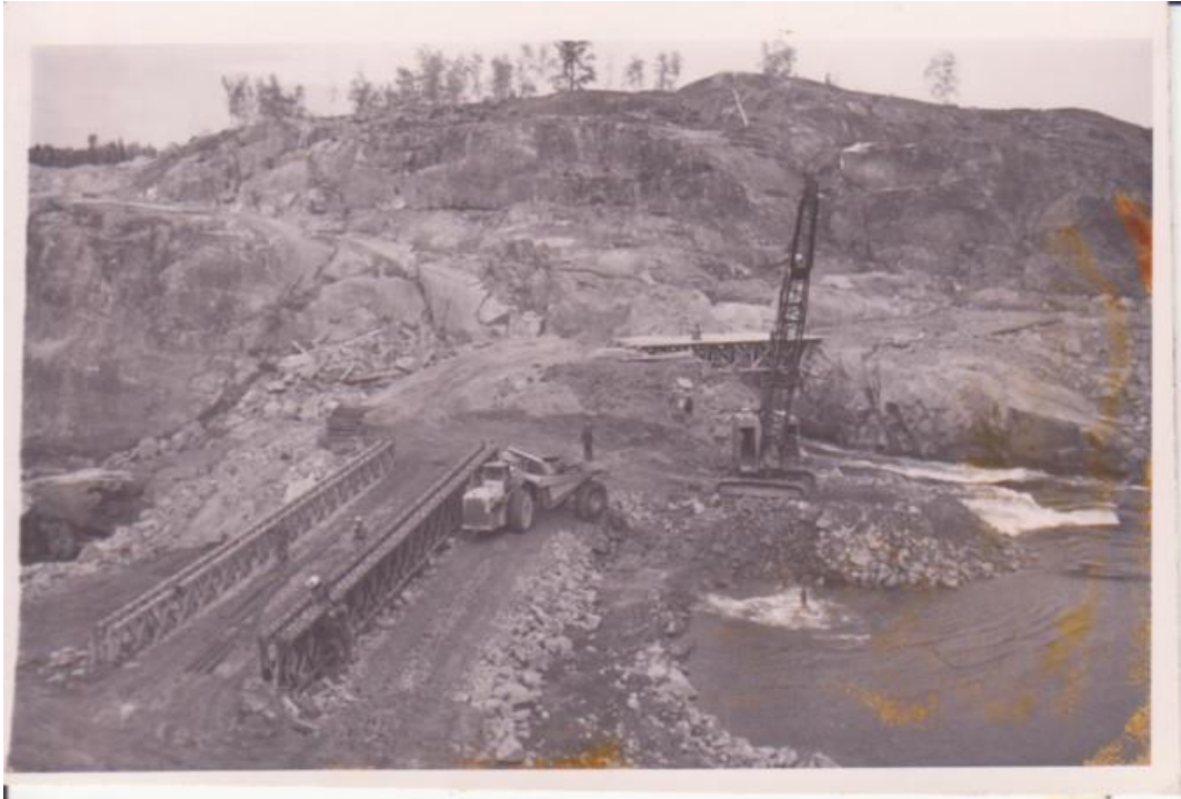
Photo 26. Shows the Main Dam Cofferd Dam and flows to Diversion Tunnel during construction.
