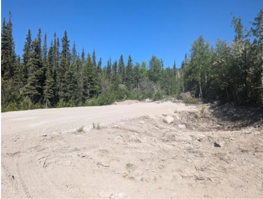
Photo 29. Shows repair to the far end of North Dyke near the Quarry. Crest raised to design grade tied to high ground.
