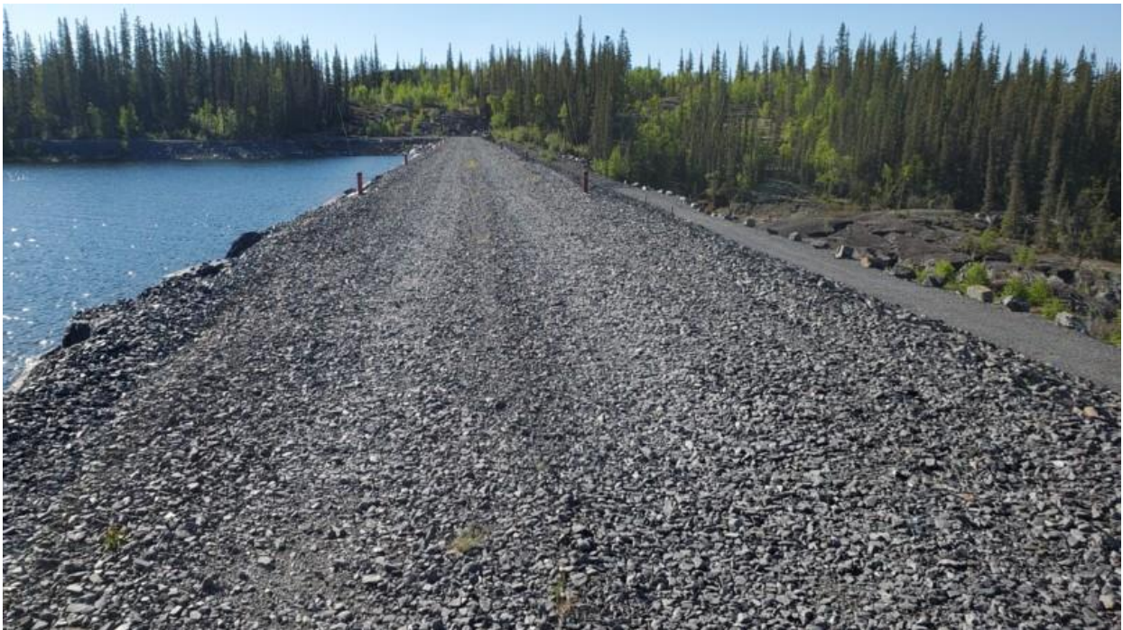
Photo 6. View of crest looking towards the left abutment. No sign of instability.
