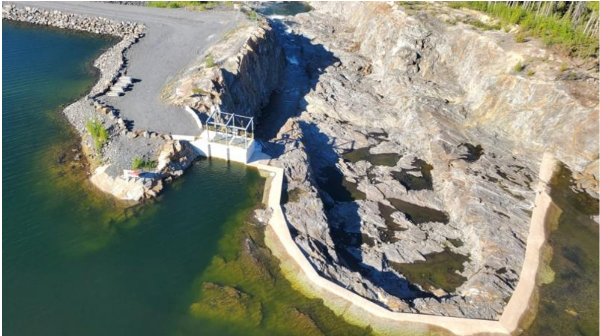
Photo 7. Shows the horseshoe Spillway, Channel and Low Level Outlet.
