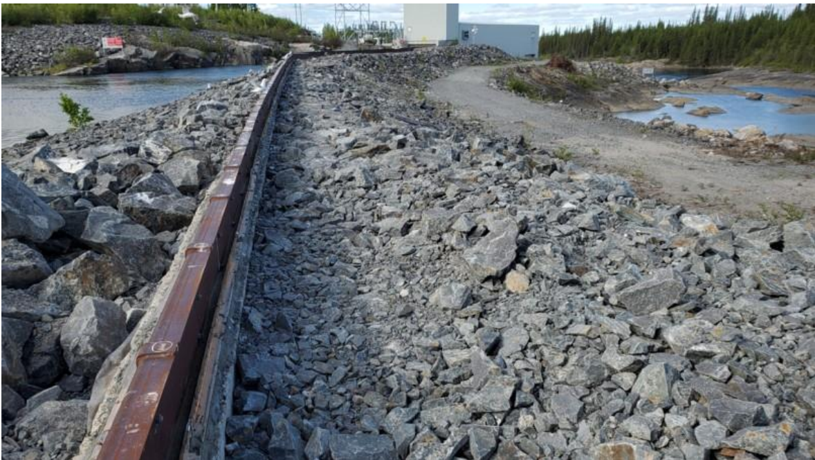
Photo 27 Shows the steel membrane, on top of Cut Off Wall. The wall provides free board protection against potential overtopping by wave action in the event of the design flood.
