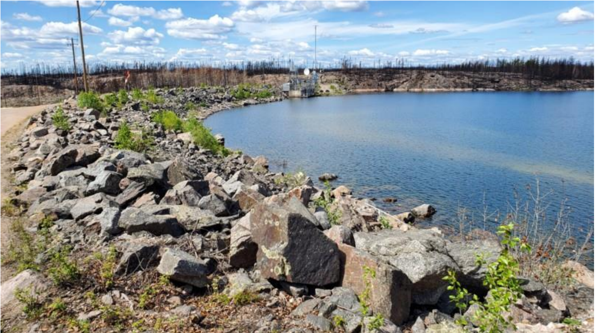
Photo 12. View of Taltson Dam seen from the left abutment. The riprap erosion protection is satisfactory except at the intake where improvement is recommended, as shown in Photo 13.
