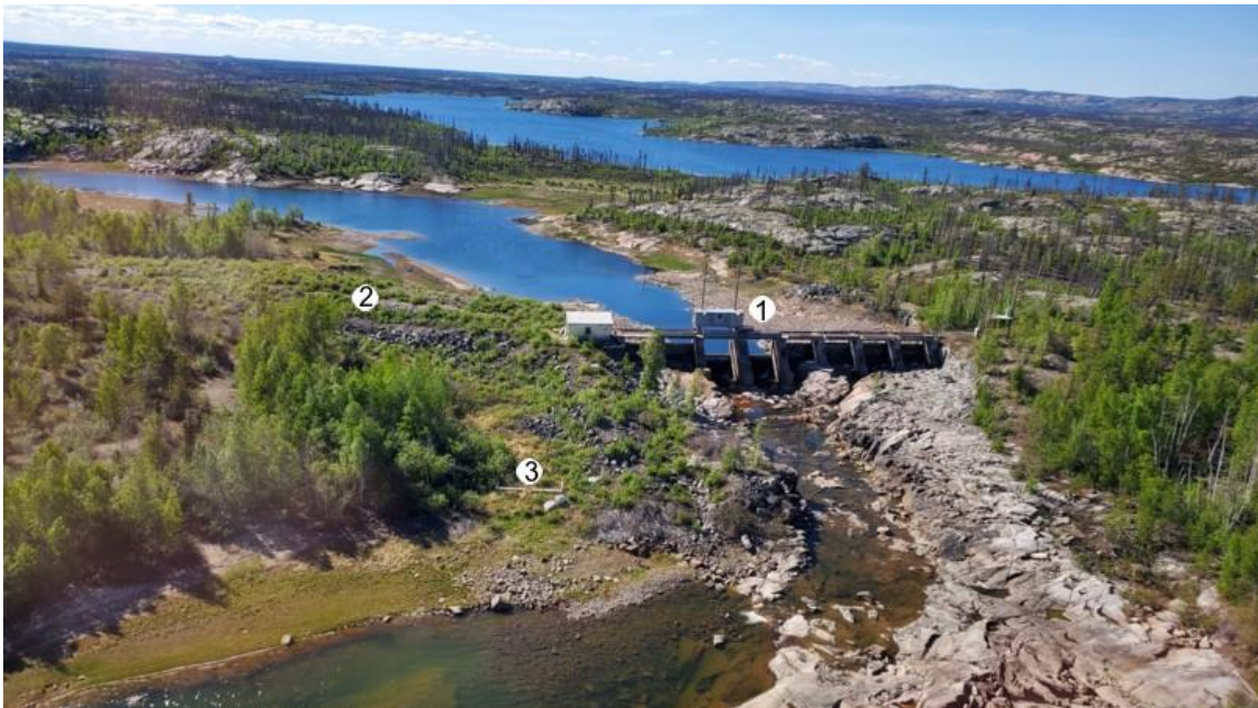
Photo 21. Shows (1). 5B Spillway; (2.) 5B Dyke & (3) Weir.
