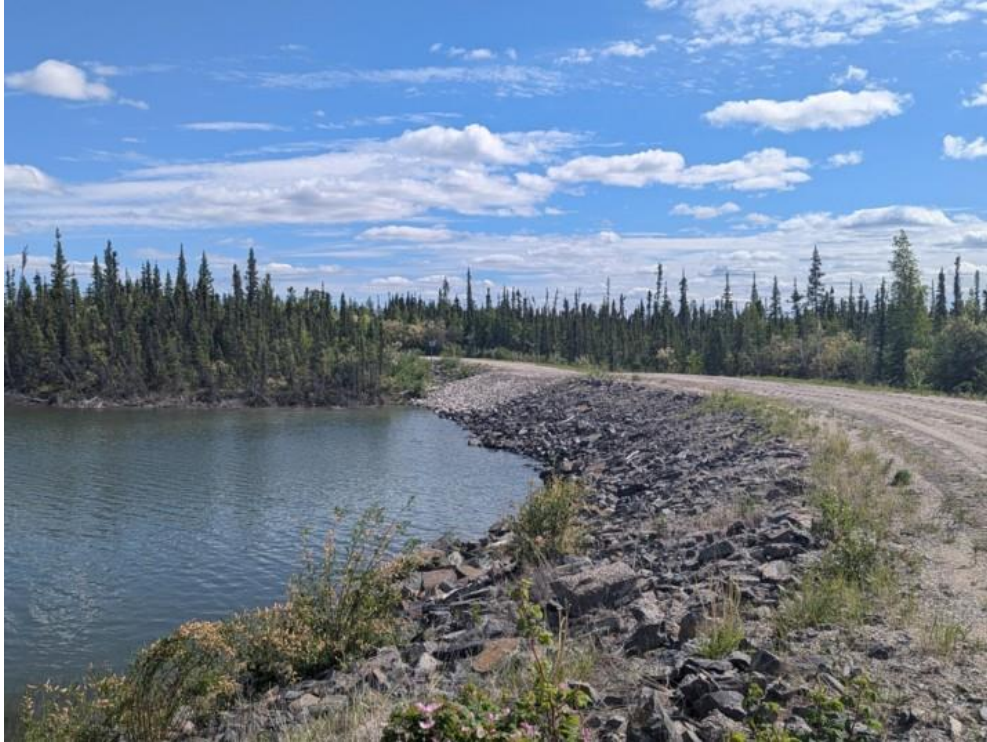
Photo 31. Shows the riprap repair to the left abutment of Dyke 3.
