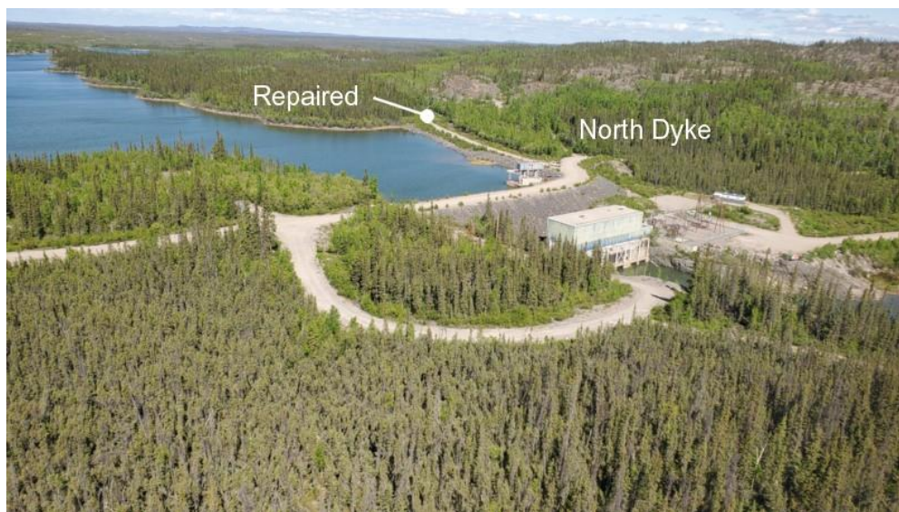
Photo 29. Shows location of 2024 repair to the North Dyke to prevent overtopping and wash-out of the main access road in event of the design flood.
