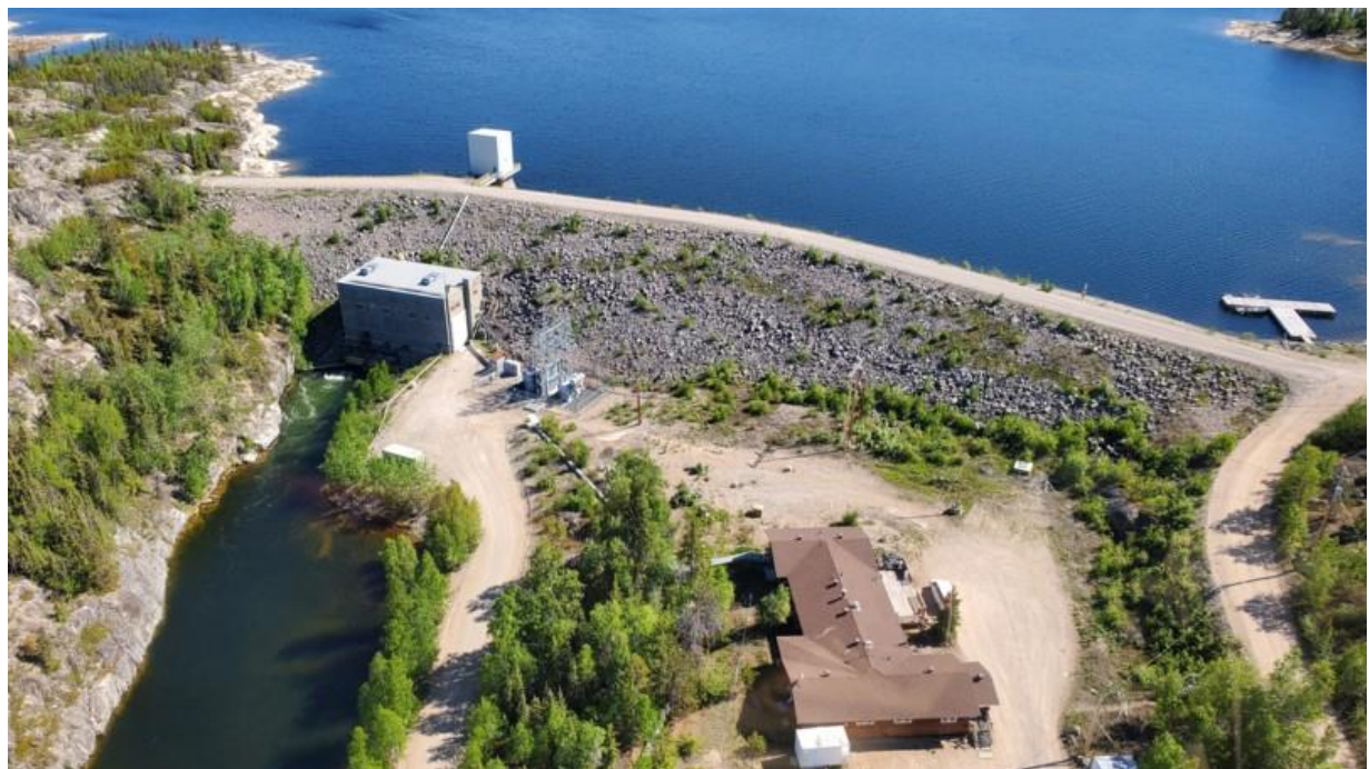
Photo 18. View of Rapids Dam and downstream area. Stable. Minor leakage, monitored.
