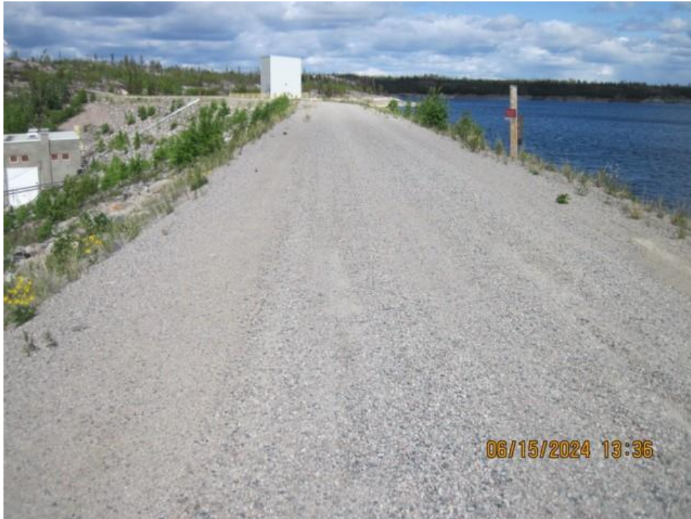
Photo 19. Rapids Dam. View of crest. Some minor cracking evident.
