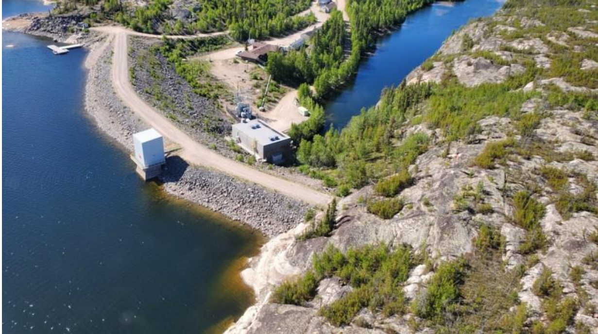
Photo 21. Upstream view of Rapids Dam. Variable riprap. No beaching. Satisfactory.
