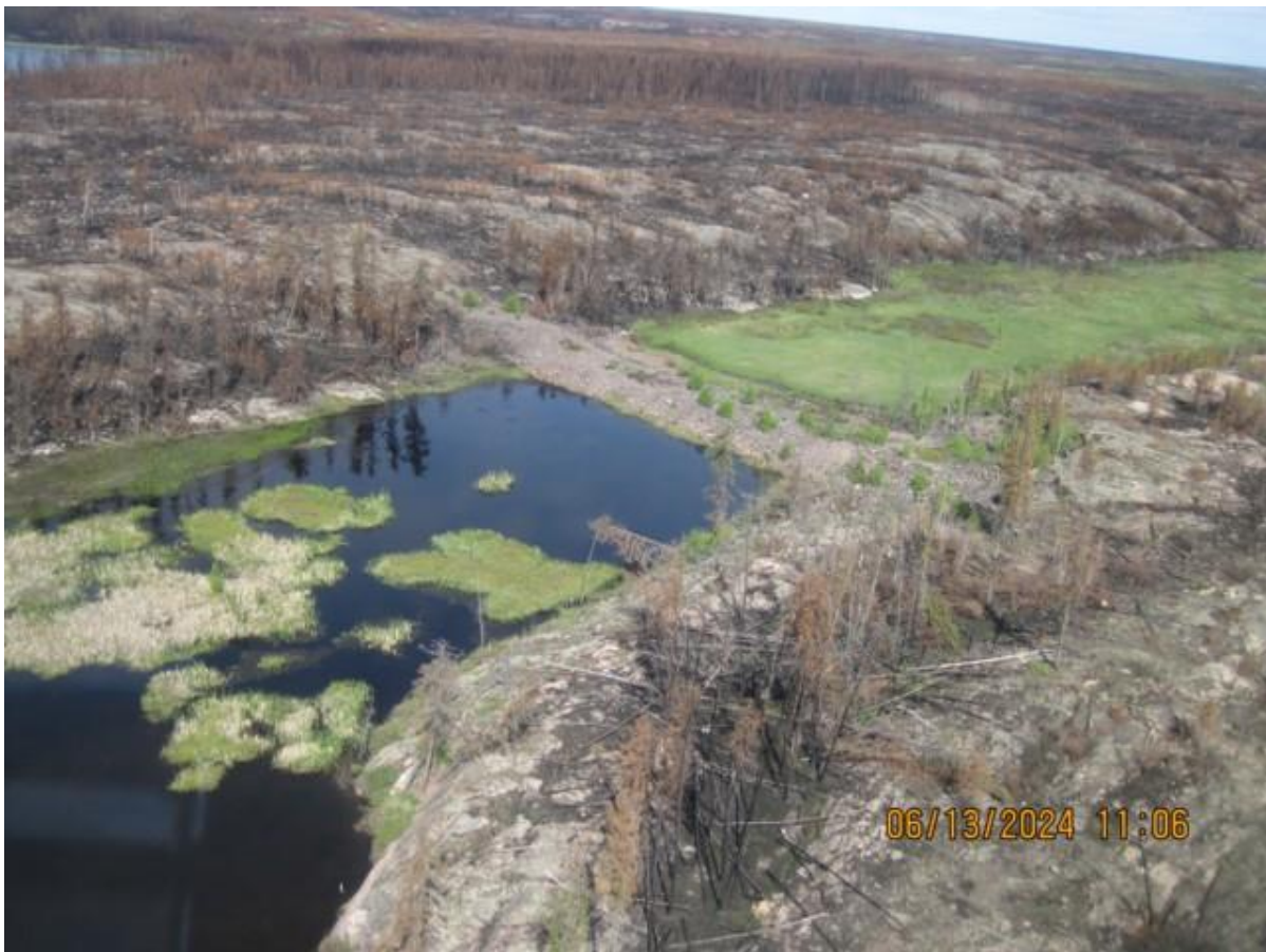
Photo 16. View of the Taltson North Valley Dam.
