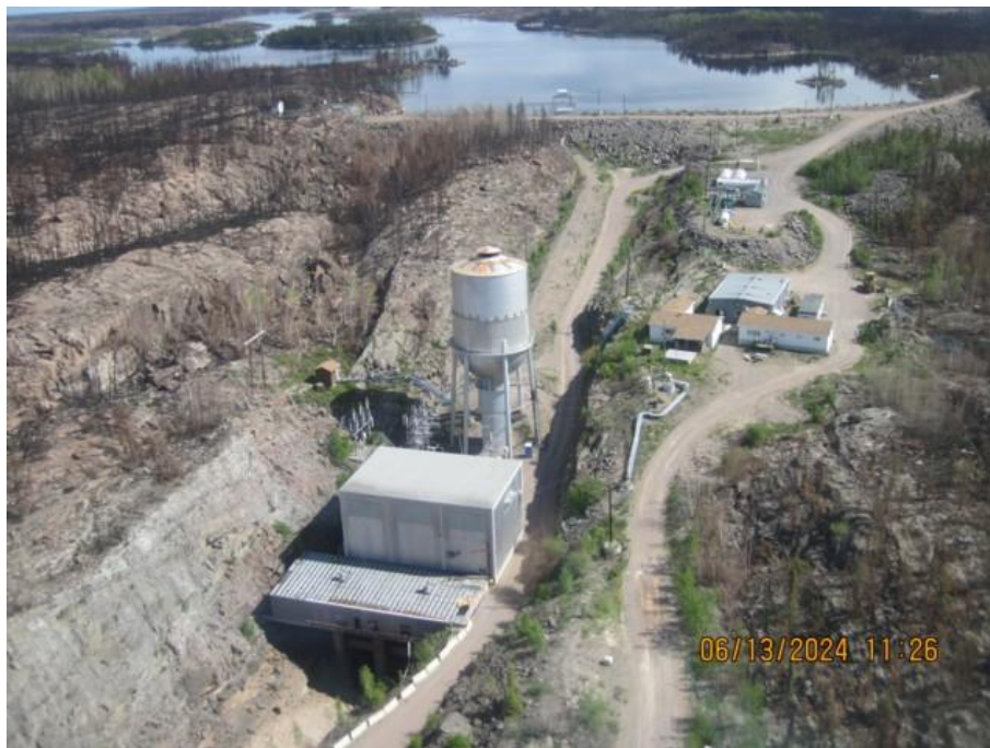
Photo 9. View of the Taltson Power Site showing the Twin Gorges Dam.
