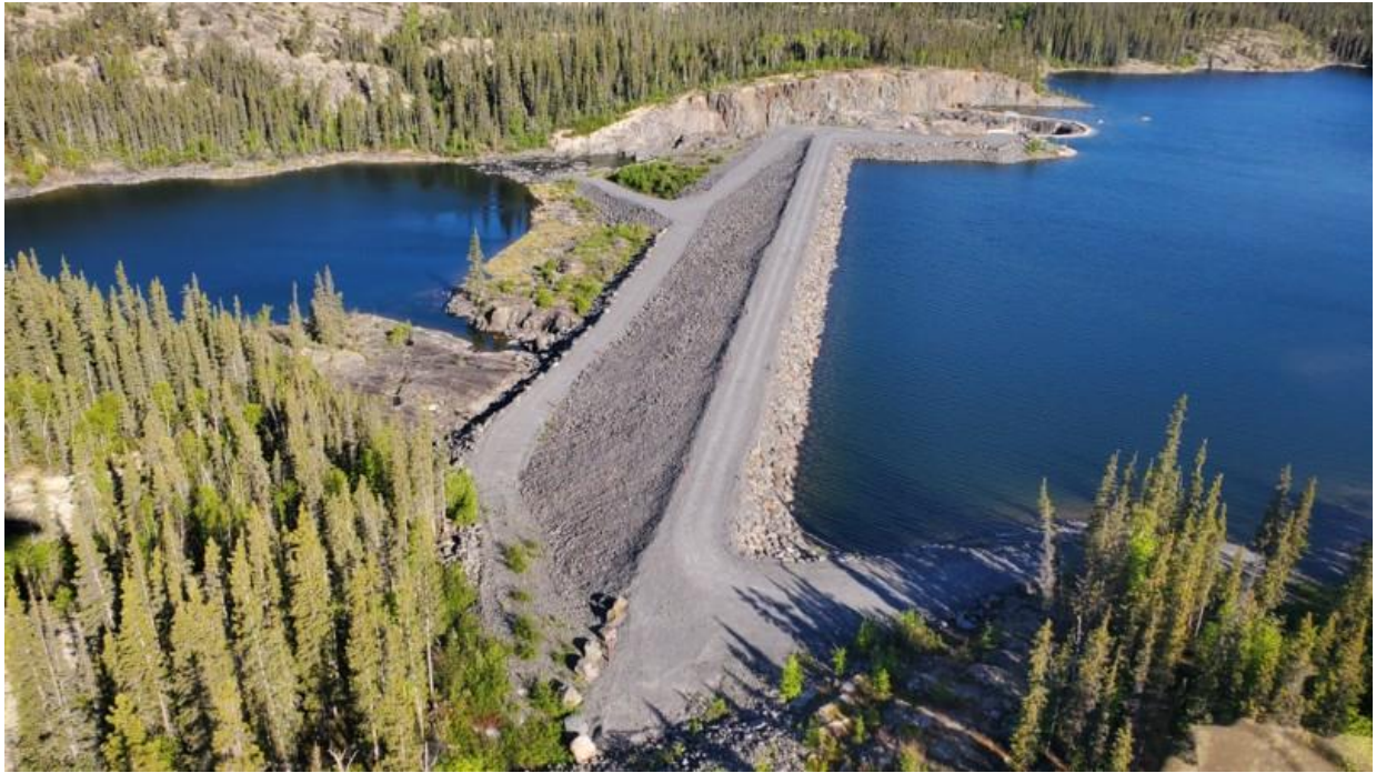
Photo 5. View of Bluefish Dam & Spillway from left side showing the spillway in the distance.
