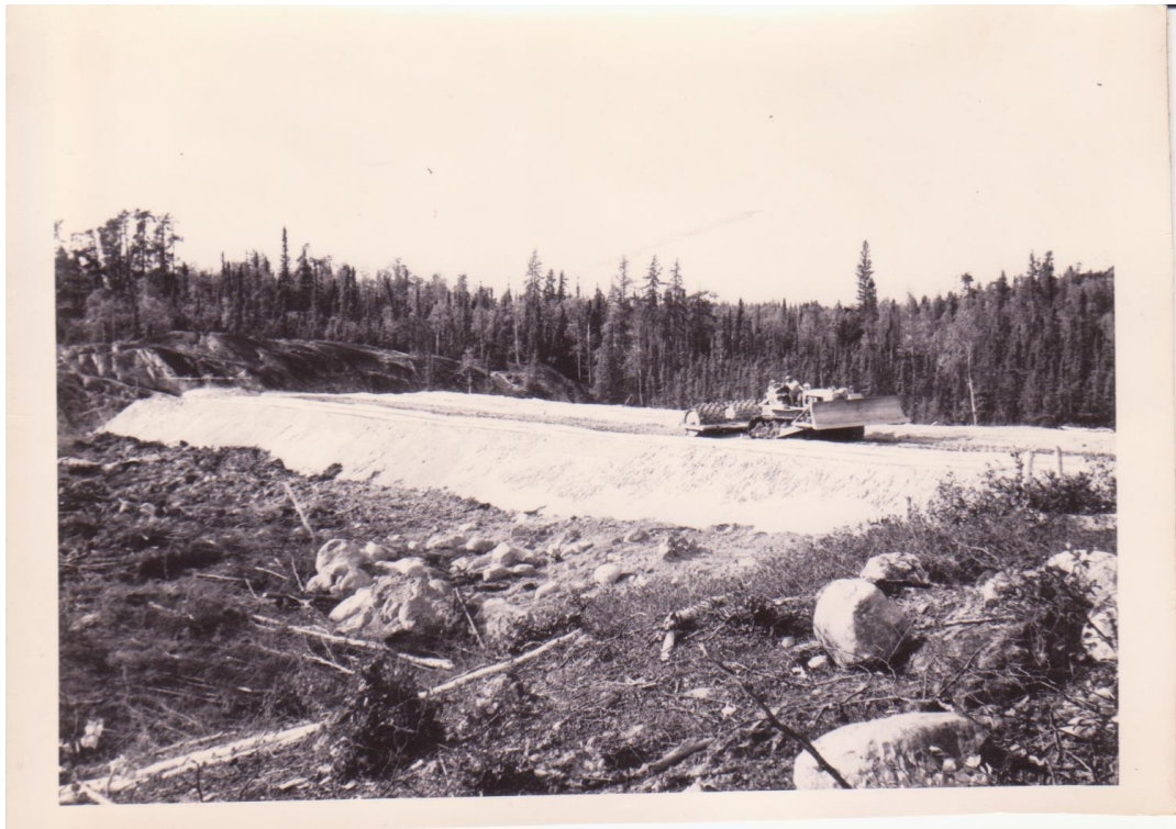
Photo 27. Side Dam construction. Compaction using sheep's foot compactor.
