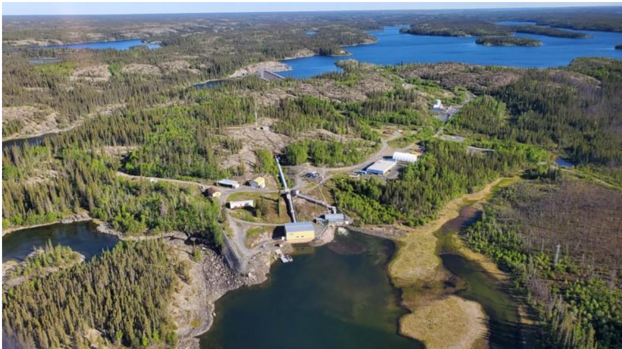
Photo 4. General view of the Bluefish Development The location of the new Rockfill Dam and Spillway constructed in 2012 can be seen near the top, middle of the photo. (see Photo 5)
