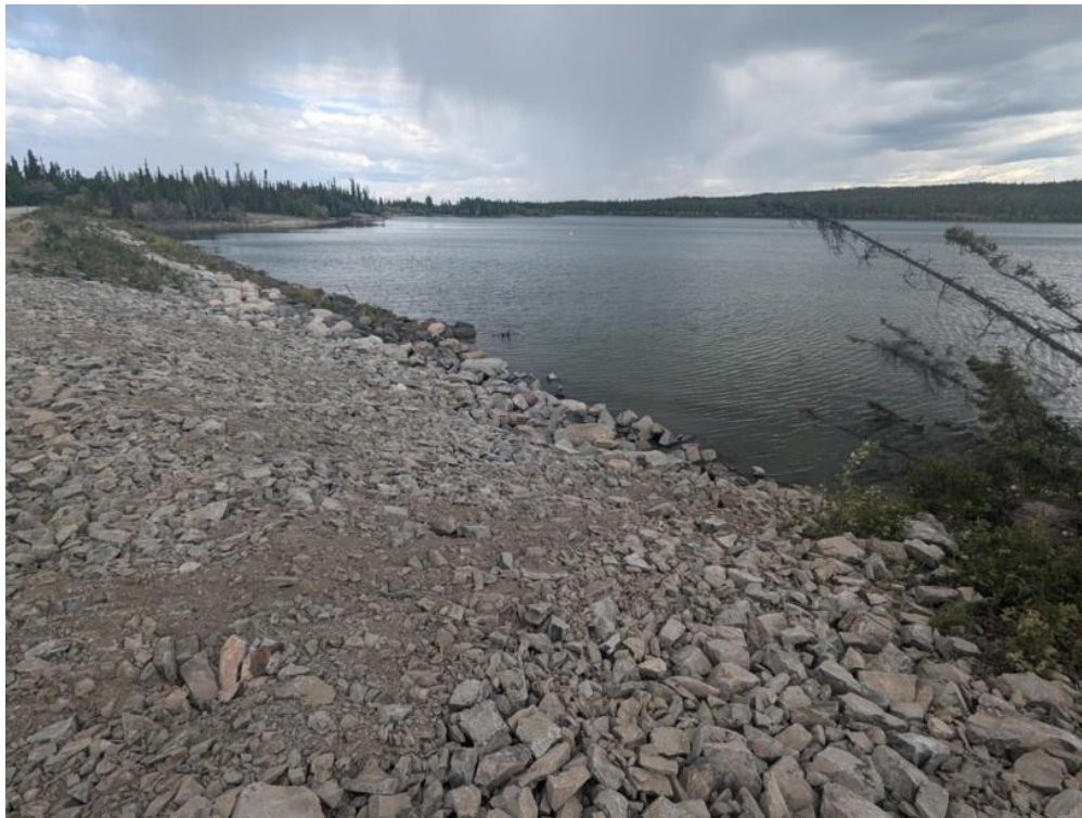
Photo 30. View of riprap repair at left abutment of Dyke 2.
