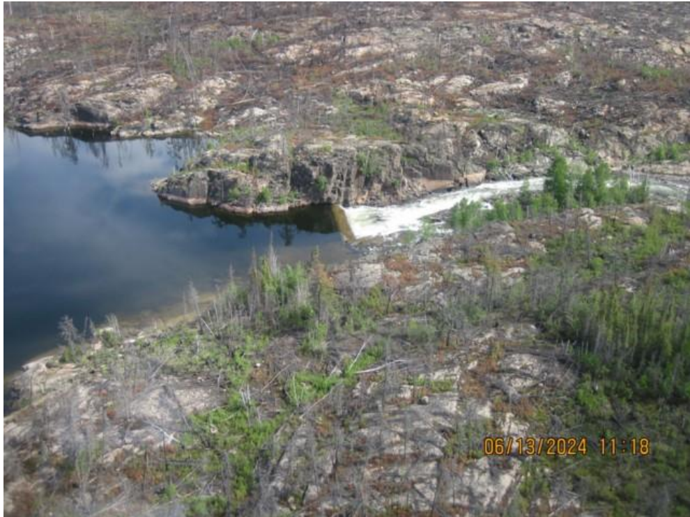
Photo 19. Spill channel at location 3 showing a concrete sill.
