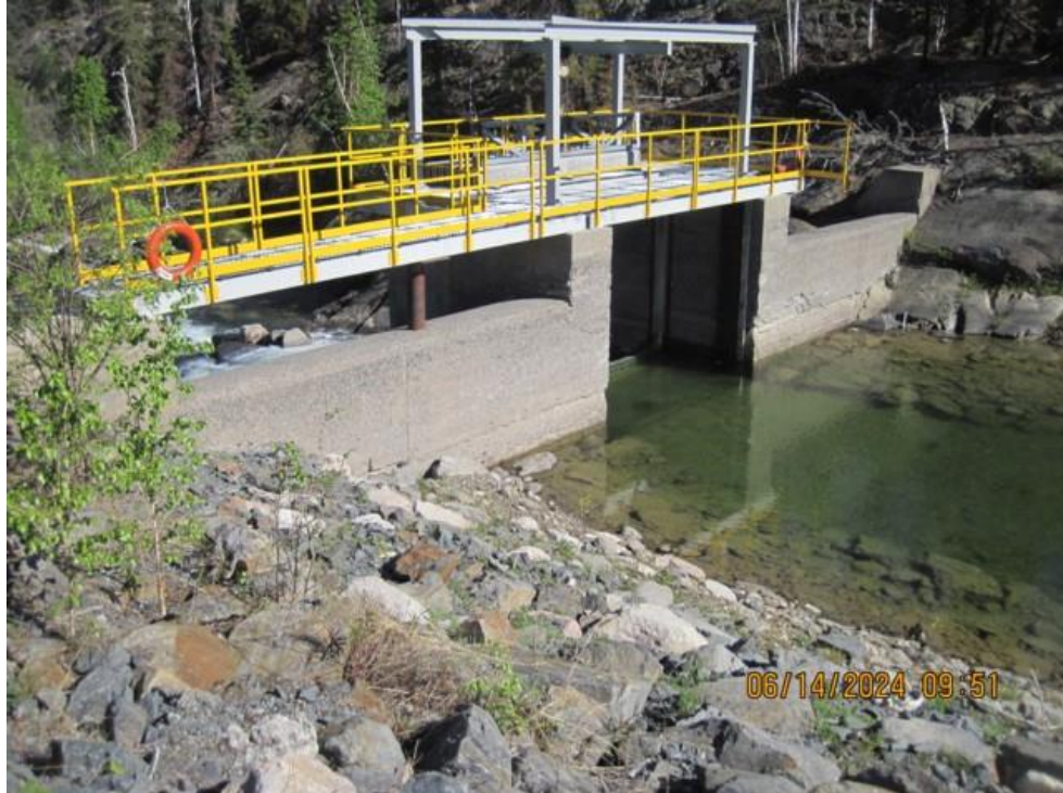
Photo 2. View of the upstream face of the Dam at low water level. The concrete and steel work is in good condition. There is some surface erosion of the concrete above the water level that was repaired this year, 2024. The Dam is structurally sound.
