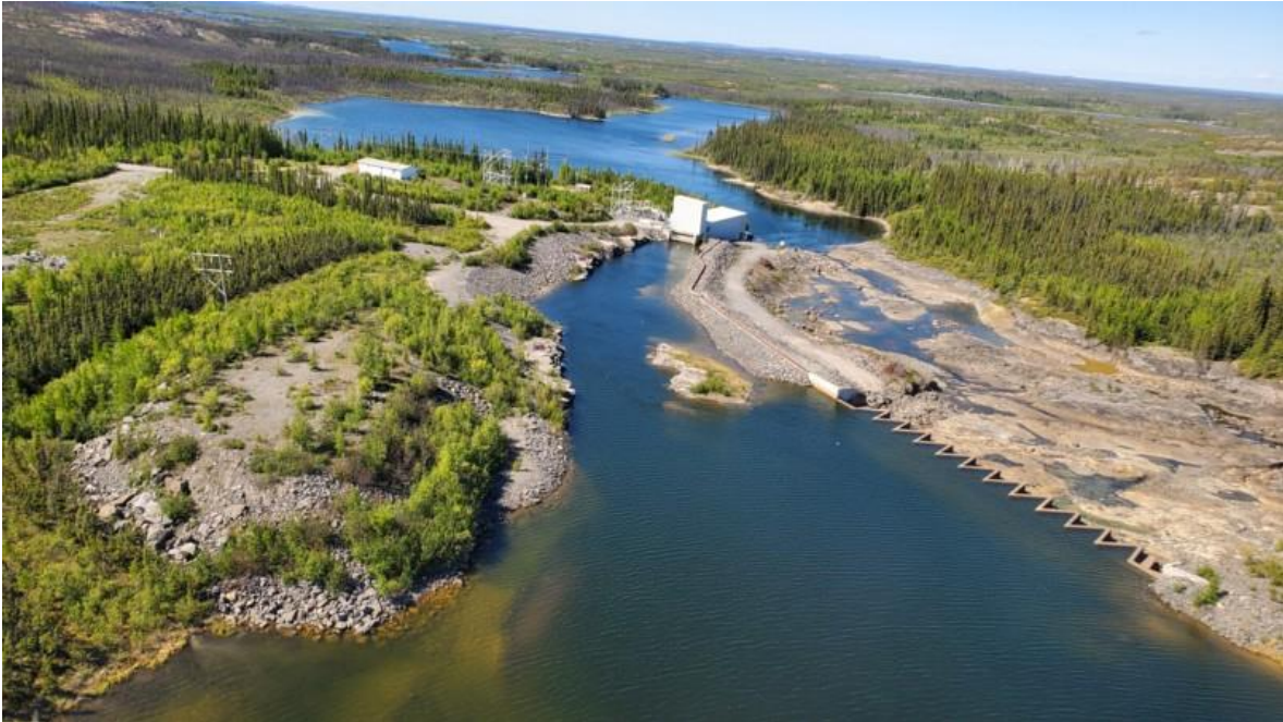
Photo 26. Shows the Cascades Development, ie: Powerhouse, Rockfill Dyke with Cutoff Wall, Spillway & Earthfill Dyke. The top of the Dyke Cutoff Wall was raised in 2023 to El 185m by installation of a 0.5m high steel membrane.
