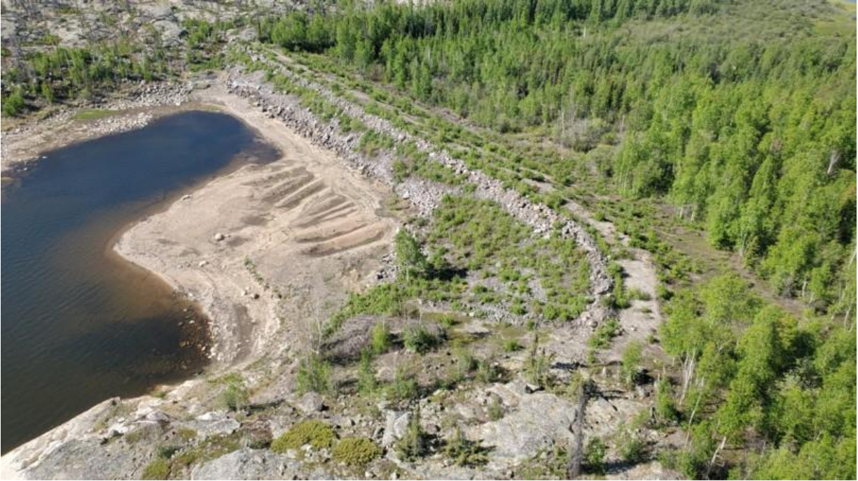
Photo 22. Aerial view of Dam 4.
