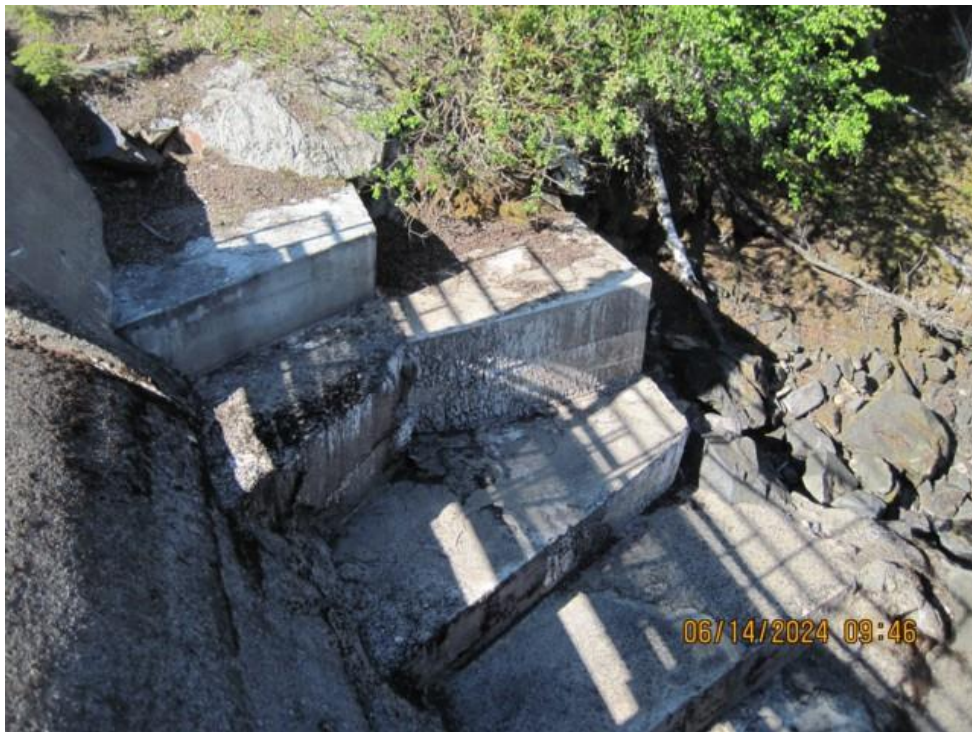
Photo 3. Shows view of the benched concrete repairs done in 2007. In good condition.
