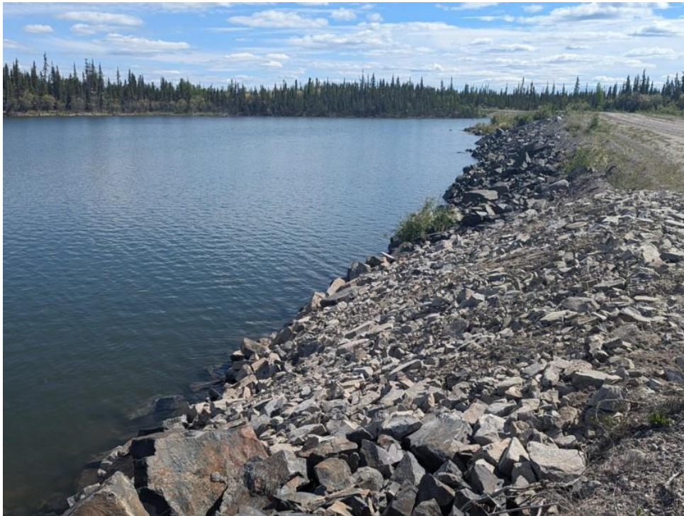
Photo 32. Shows enhancement to riprap at Forks Main Dam.
