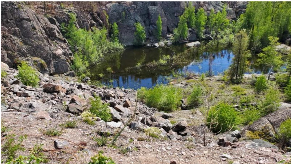
Photo 15. View of the Dam at the South Gorge. The level of the pond at the downstream toe is recorded by a camera and calibrated rod (gage). No indication of leakage flow in the pool.
