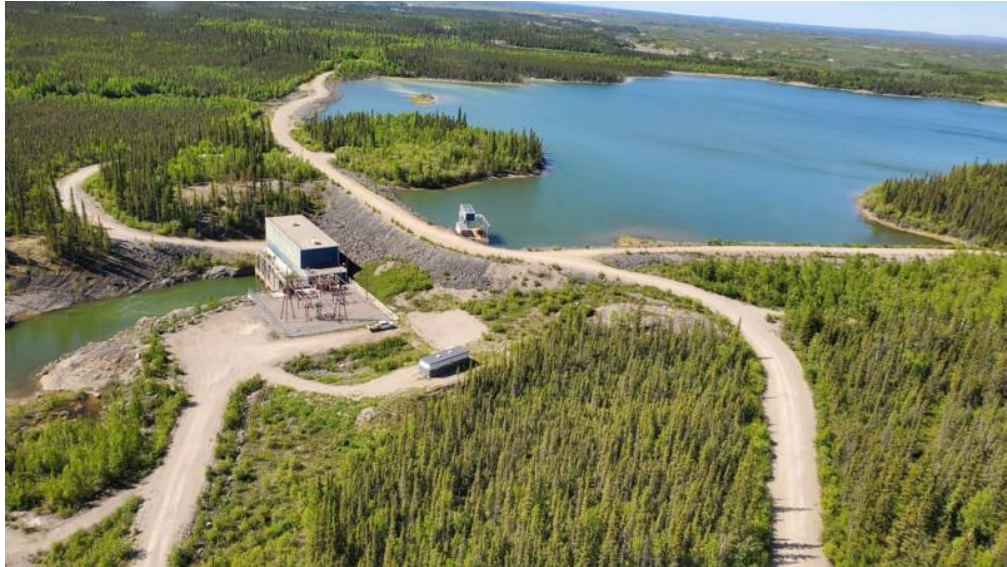
Photo 28. Strutt Lake Dam. North Arm Dyke on the right of the photo.
