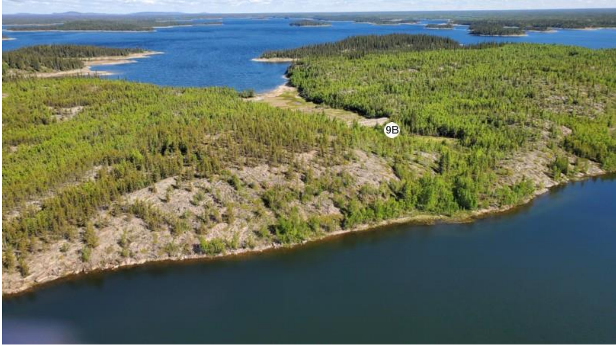
Photo 23. View of Freeboard Dyke 9B.
