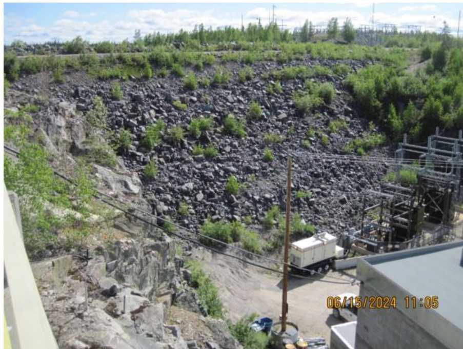
Photo 25 Shows the downstream face of the Main Dam. Stable. No visible leakage.
