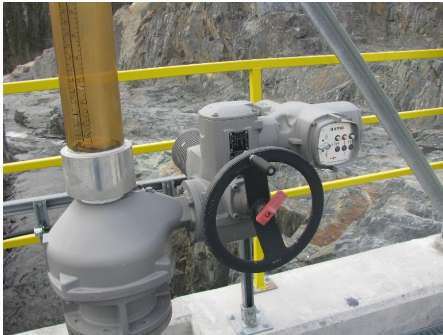
Figure 3-1: Bluefish IFR Gate Manual Control
