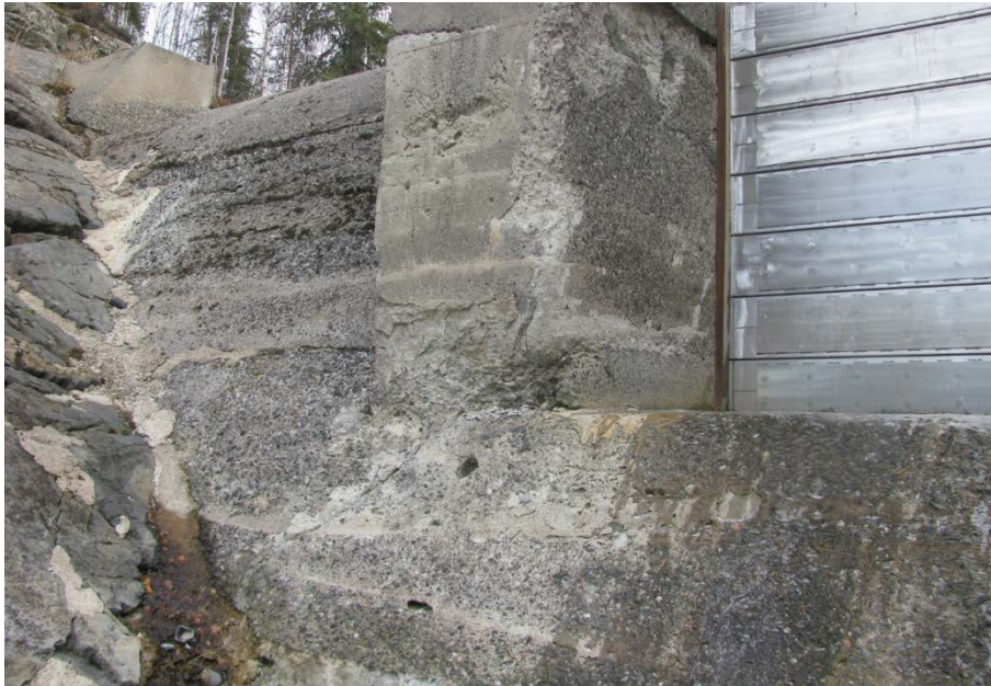
Figure 6-8: Downstream side of piers and side face shows signs of freeze-thaw damage. Eroded concrete zone should be patched to reinstate concrete cover
