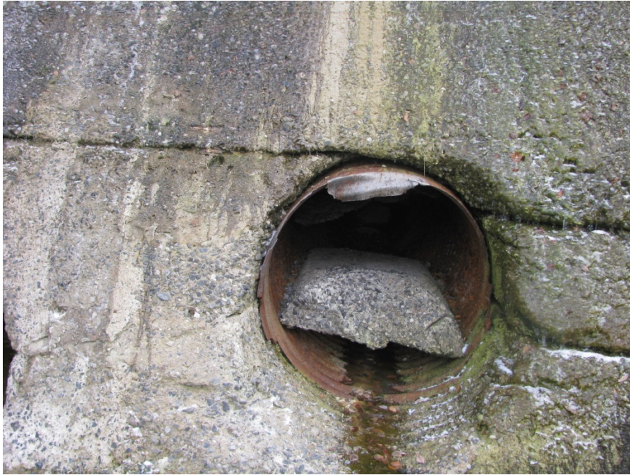
Figure 6-11: Abandoned low level conduit appears to be in fair condition
