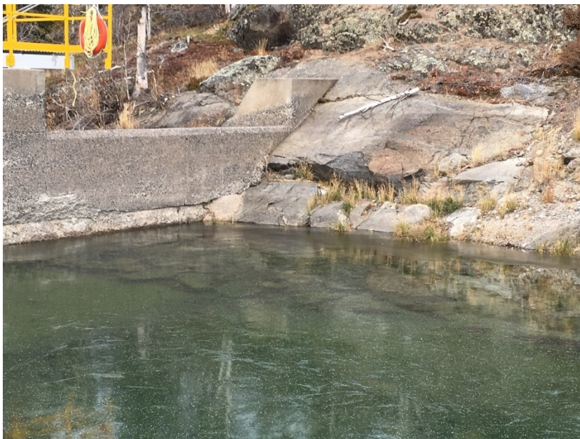
Figure 6-16: Joints/fractures parallel to the direction of water flow present an opportunity for seepage to pass beneath the concrete during higher water elevations.
