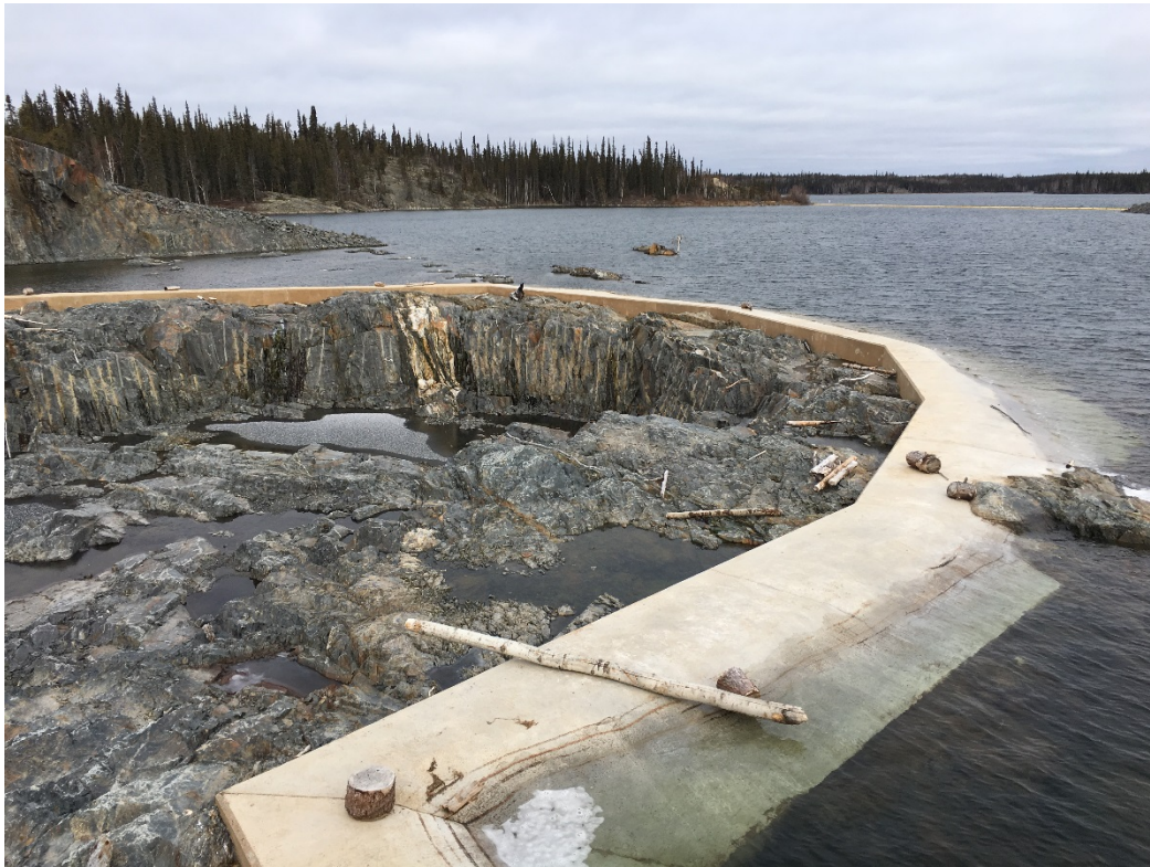
Figure 5-7: Condition of upstream spillway vertical rock face.
