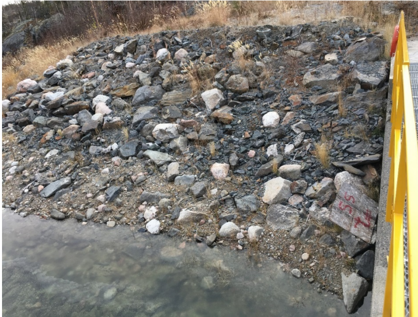
Figure 6-15: Upstream left abutment conditions – exposed fine grained soils within water flow areas could be eroded at higher water elevations.
