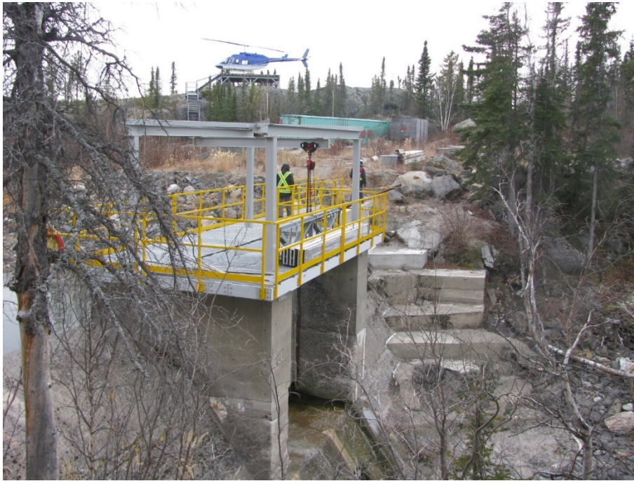
Figure 6-9: Stepped concrete added to downstream side of dam. Concrete appears to be in good conditions
