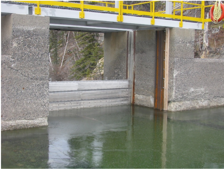
Figure 6-3: Freezing damage/spawling at waterline
