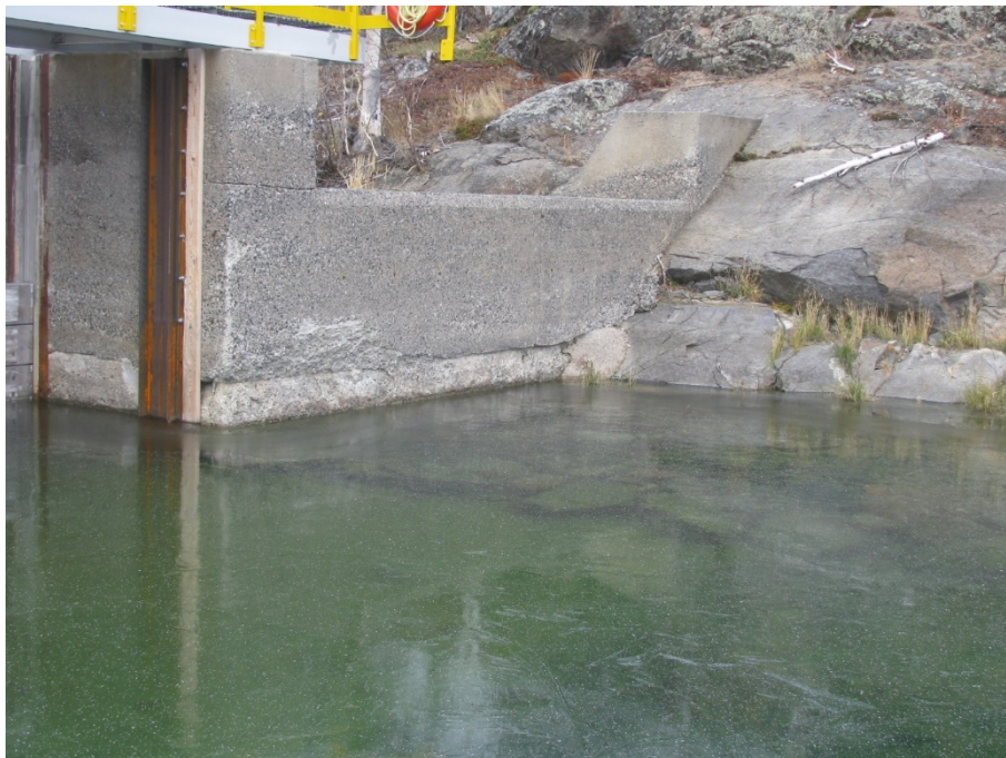
Figure 6-4: Abutment/overflow section appears to be in good condition. Interface between rock and concrete appears to be tight.
