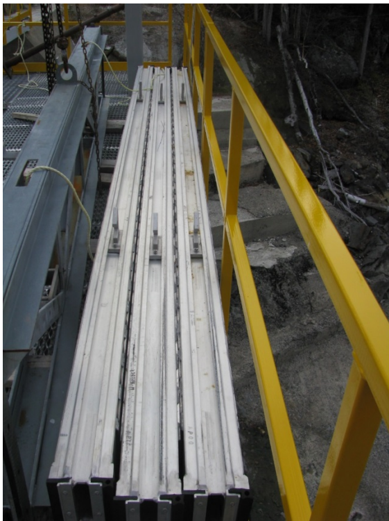
Figure 6-12: Metal stoplogs on operational platform appear to be in good condition.
