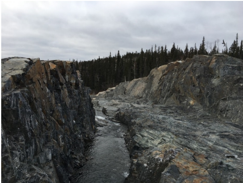
Figure 5-10: Low Level Outlet channel left wall and main spillway channel right wall and rock base
