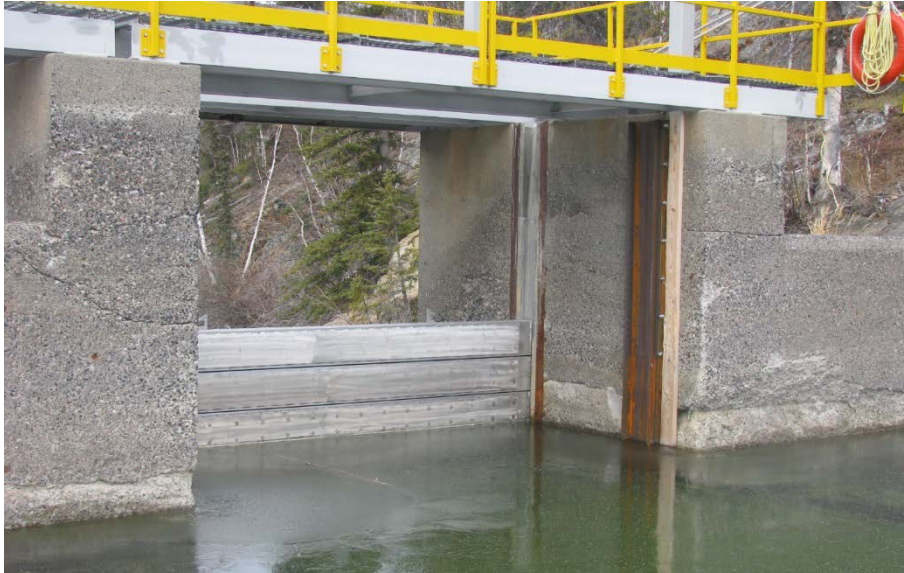
Figure 6-7: Crack visible on upstream side of both piers near rollway crest on both piers. Cracks to be epoxy injected
