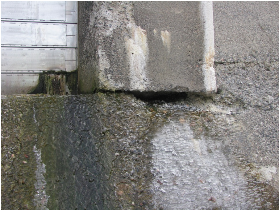
Figure 6-10: Downstream pier base has eroded and some leakage is evident. Toe of pier should be repaired
