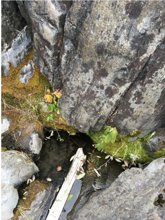
Figure 5-5: Observed seepage from base of dam at former river channel location.
