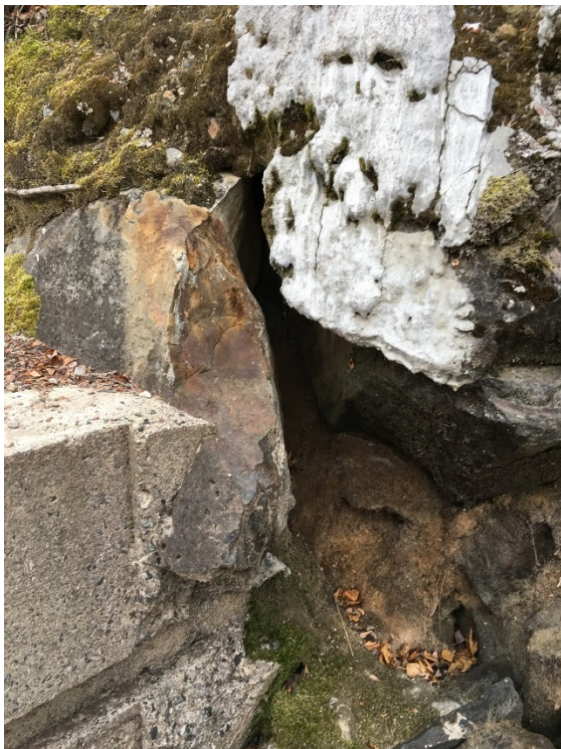
Figure 6-14: Example of voids in blast rock/rubble of the left abutment.
