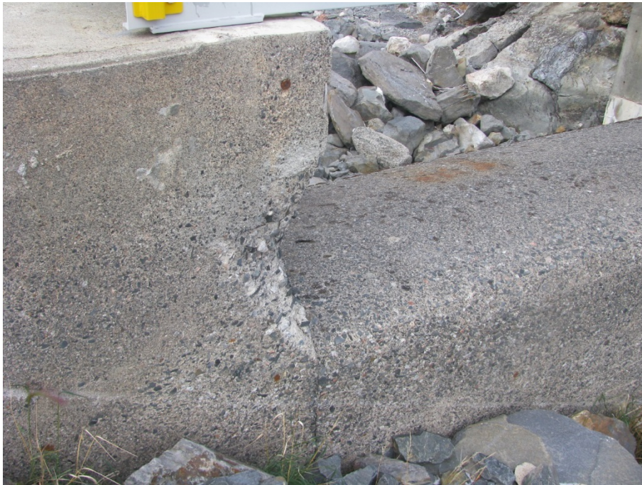
Figure 6-5: Eroded concrete at abutment upstream corner at rollway. Concrete should be rebuilt to protect from further damage.
