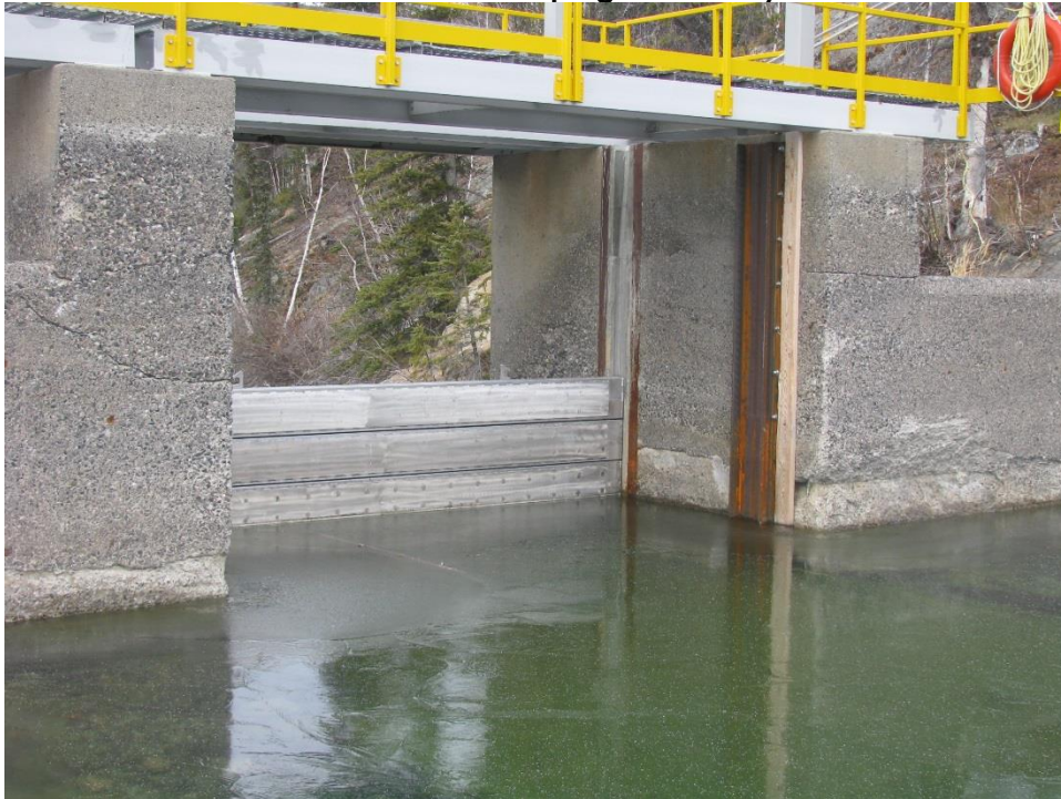
Bluefish Dam – Stoplogs sluiceway
