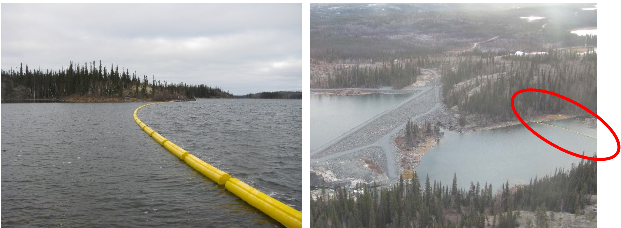
Figure 9-1: Safety booms upstream and downstream of Bluefish dam.
