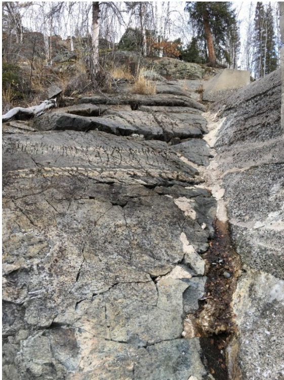
Figure 6-13: Minor seepage observed along the rock/concrete contact of the right abutment
