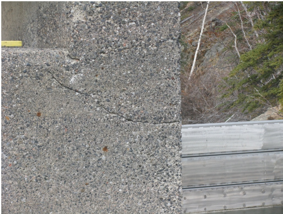
Figure 6-6: Large cracks (2 cracks) at pier to rollway interface. Cracks should be epoxy injected
