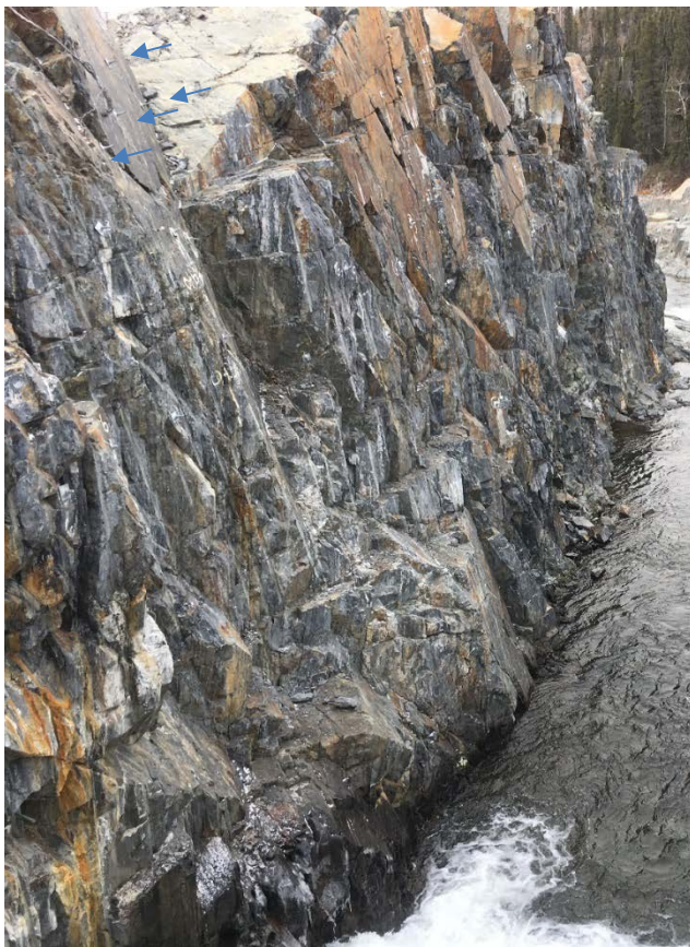
Figure 5-11: Low Level Outlet channel left wall with some anchor locations shown securing areas of the upper rock wall
