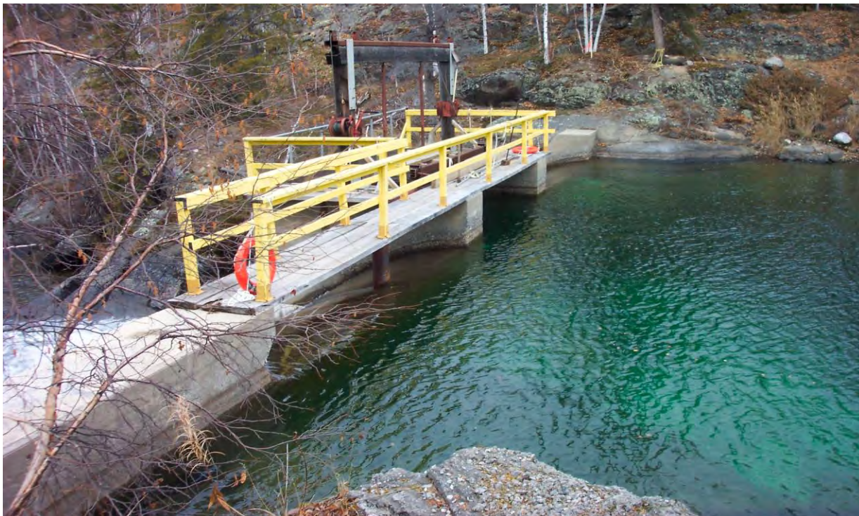
Figure 11: Duncan Lake Spillway Dam
