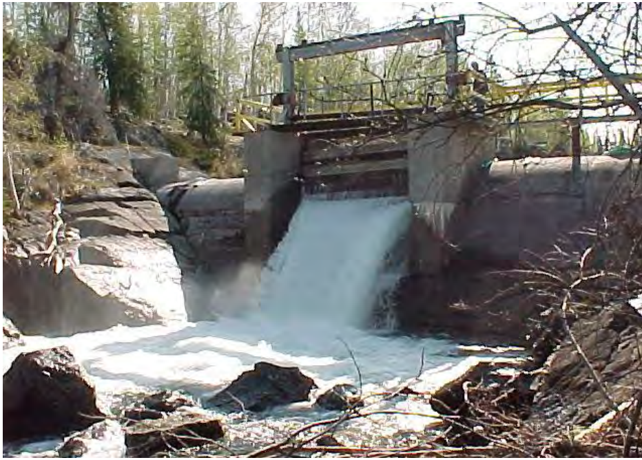
Figure 6: Duncan Lake Control Structure
