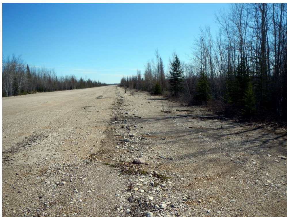
Photo 2: Existing Haul Road at Pine Point
