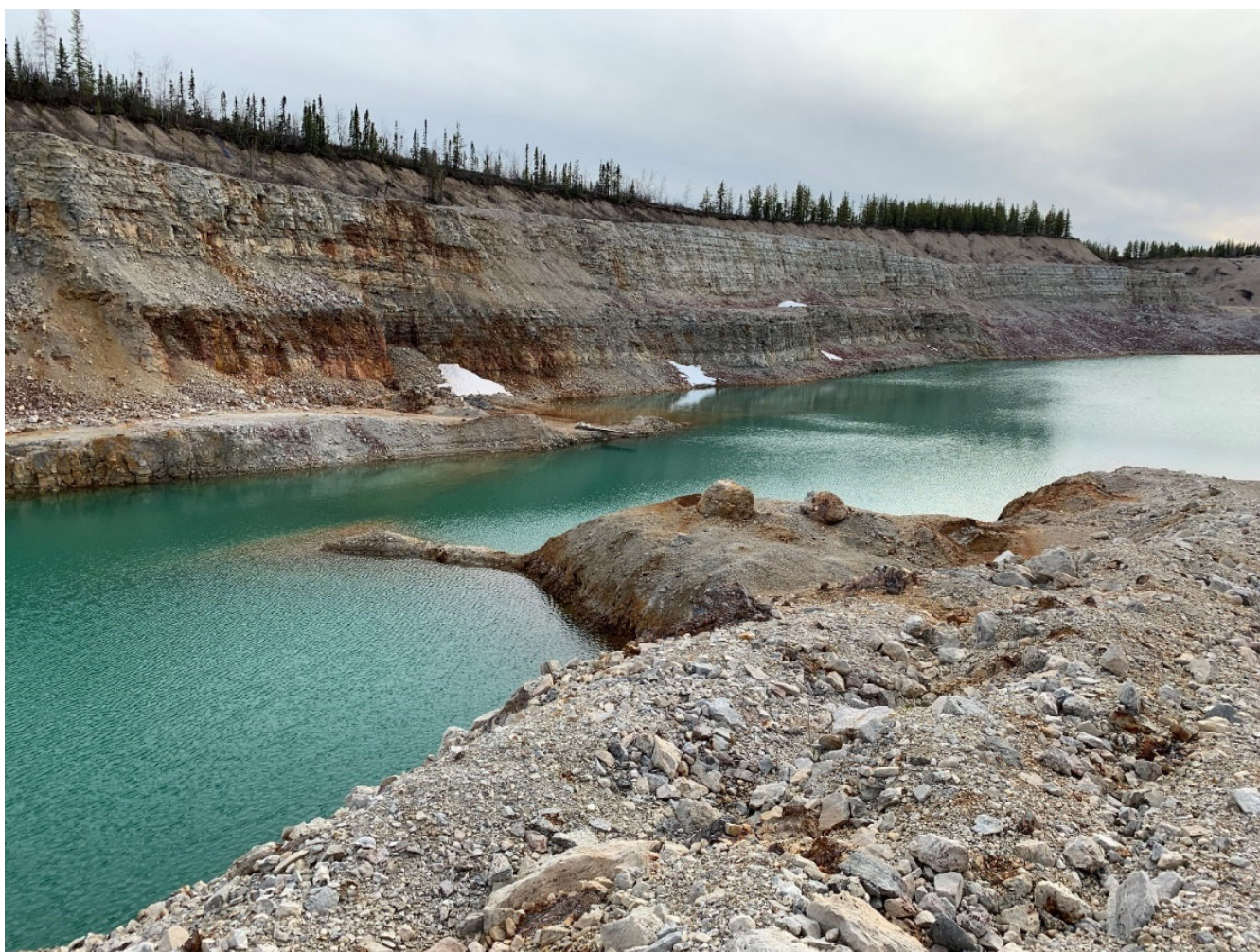
Photo 3: Abandoned Open Pit near the Pine Point Townsite
