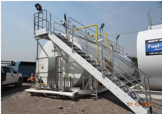
Figure 10 90,000L Diesel fuel tank located in the storage and distribution area.
