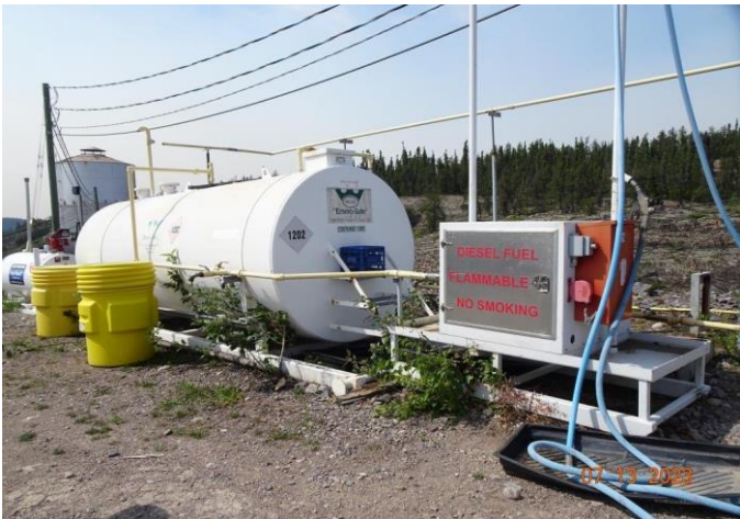
Figure 9 13,600L Diesel fuel tank located in the storage and distribution area.
