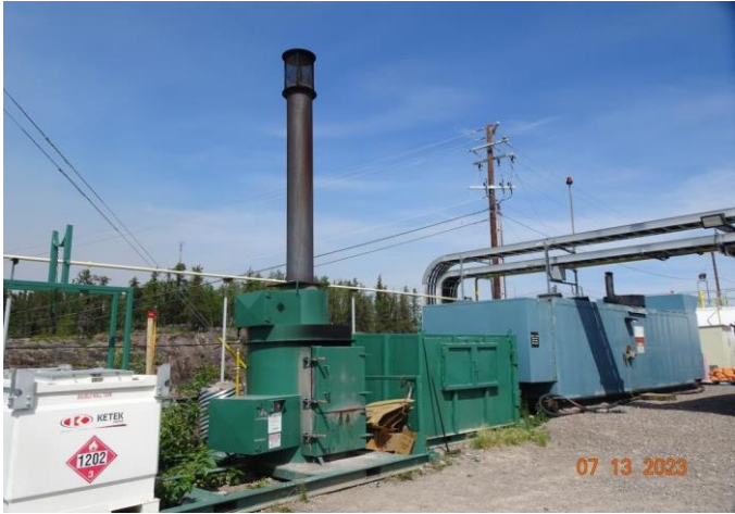
Figure 16 Incinerator and existing generator located in the storage and distribution area.
