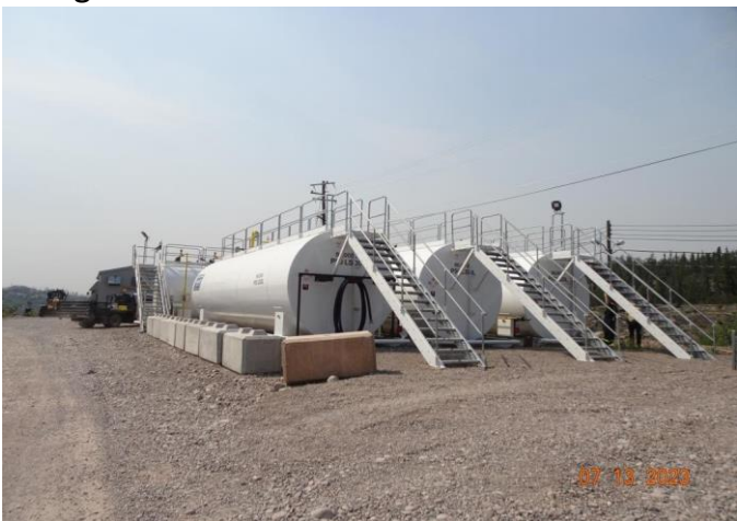
Figure 11 3 x 90,000L Diesel fuel tanks located in the storage and distribution area.
