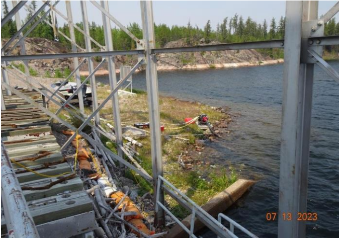
Figure 13 Emergency water pump and 25L jerry can without secondary containment located at the head gate.
