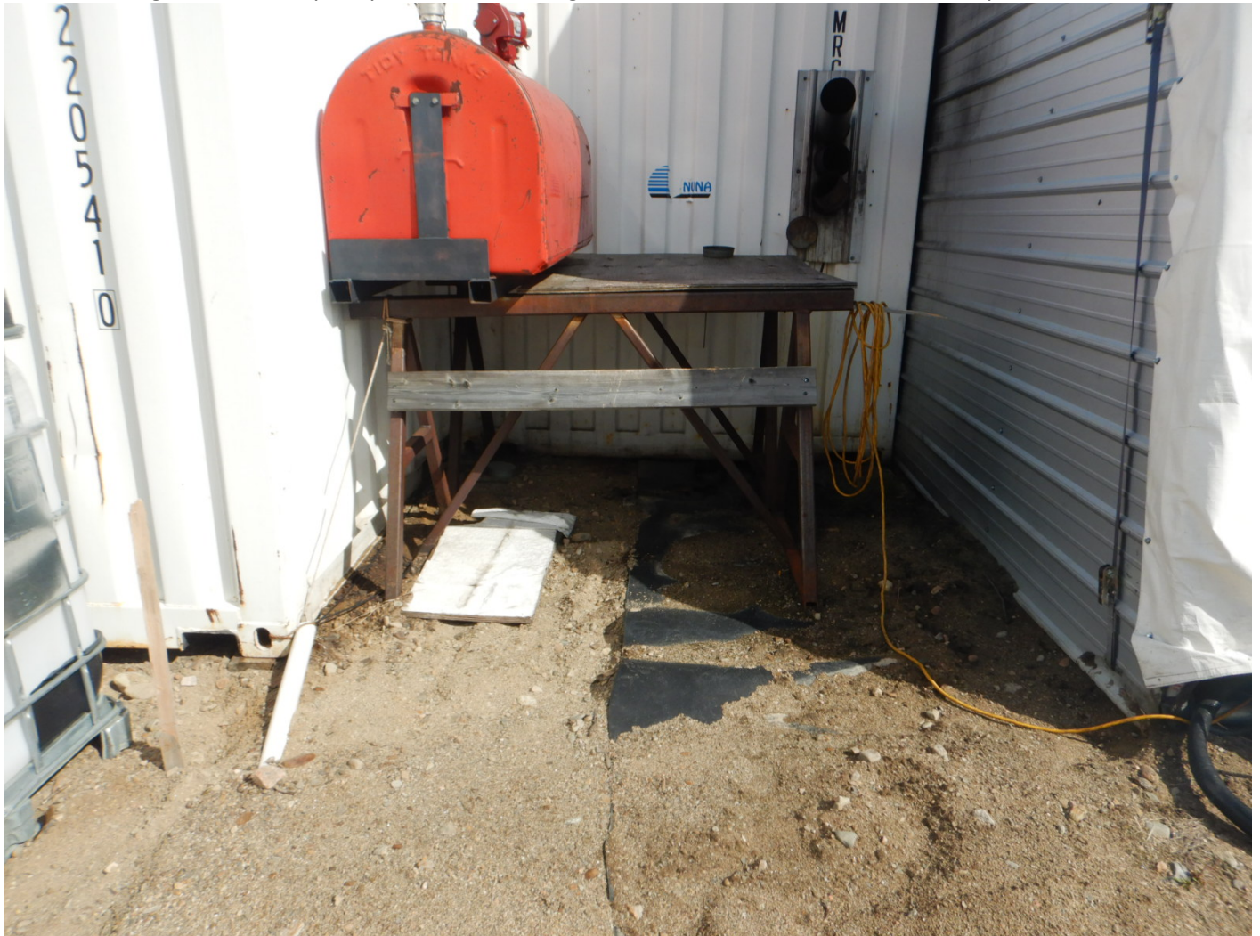
Photo 7 - Margaret Lake Camp – Hydrocarbon staining below raised tank has been cleaned-up.
