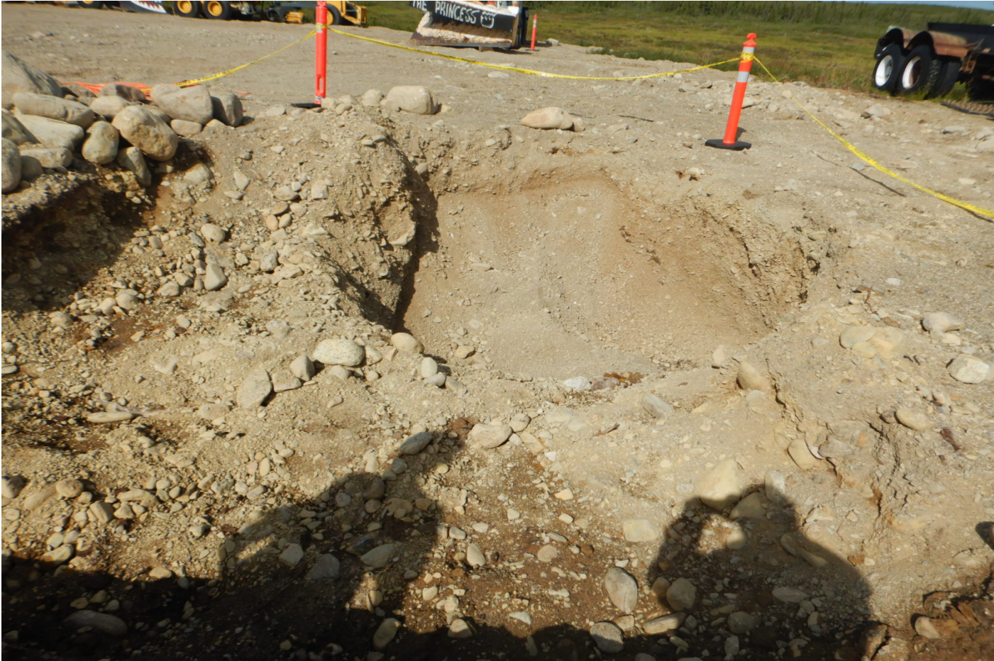
Photo 2 – Margaret Lake Camp – Previously identified spill area excavation.
