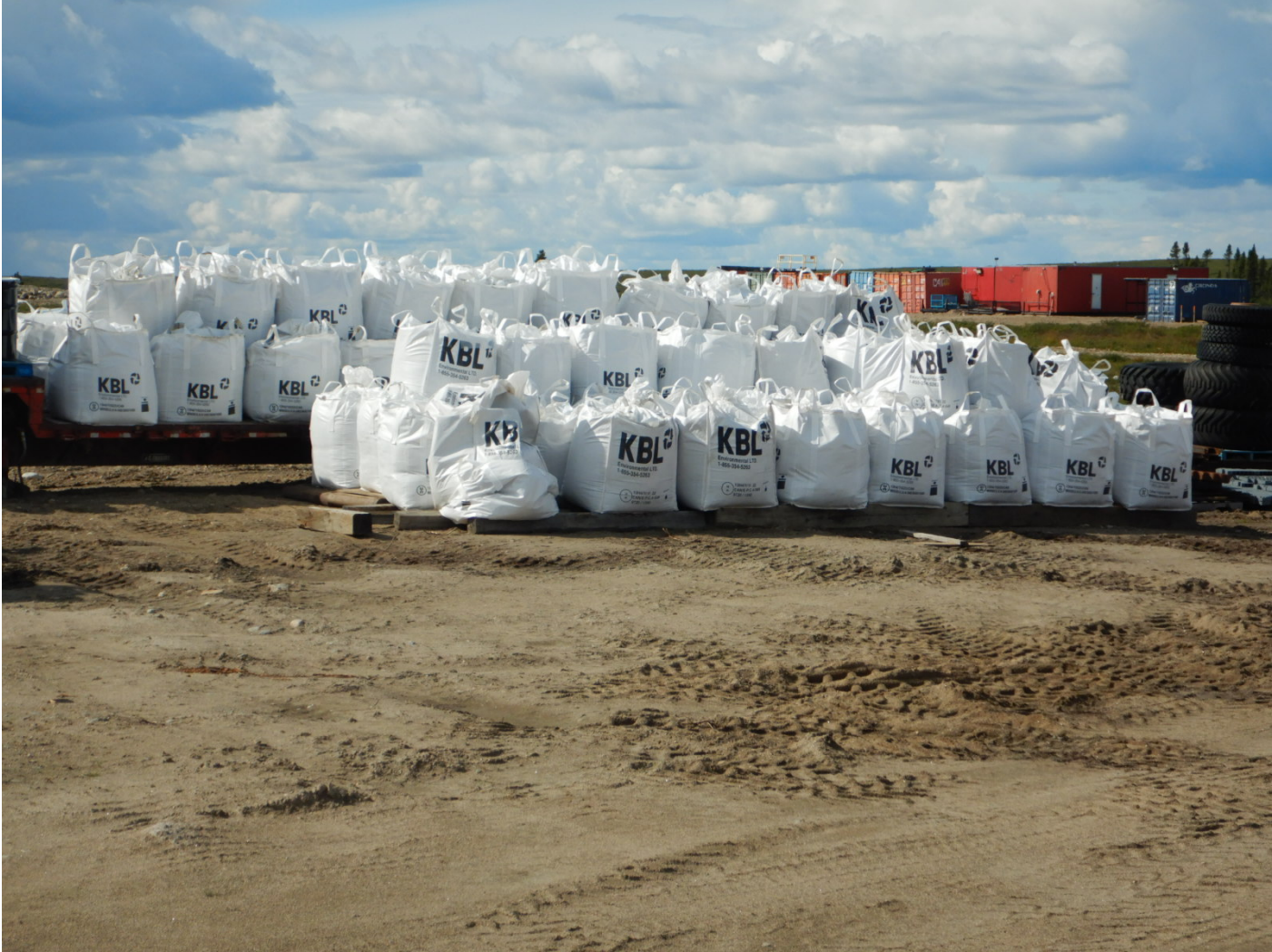
Photo 13 - Margaret Lake Camp – Mega bags of hydrocarbon contaminated soil from cleanup.
