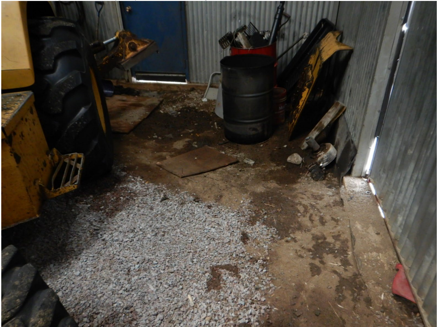
Photo 15 - Margaret Lake Camp – Hydrocarbon staining inside the maintenance shop.
