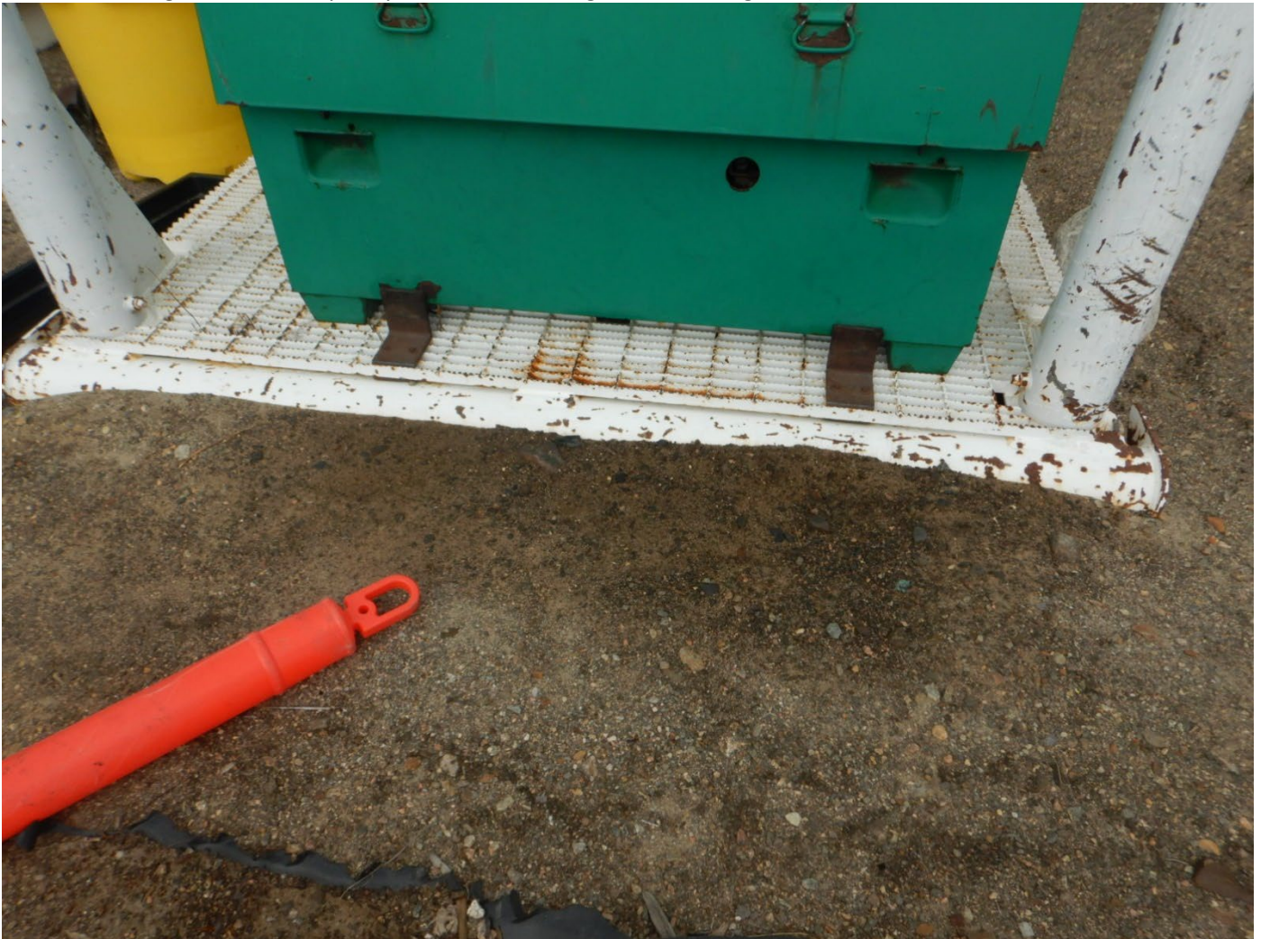
Photo 13 - Margaret Lake Camp – Hydrocarbon staining near refueling area (2).
