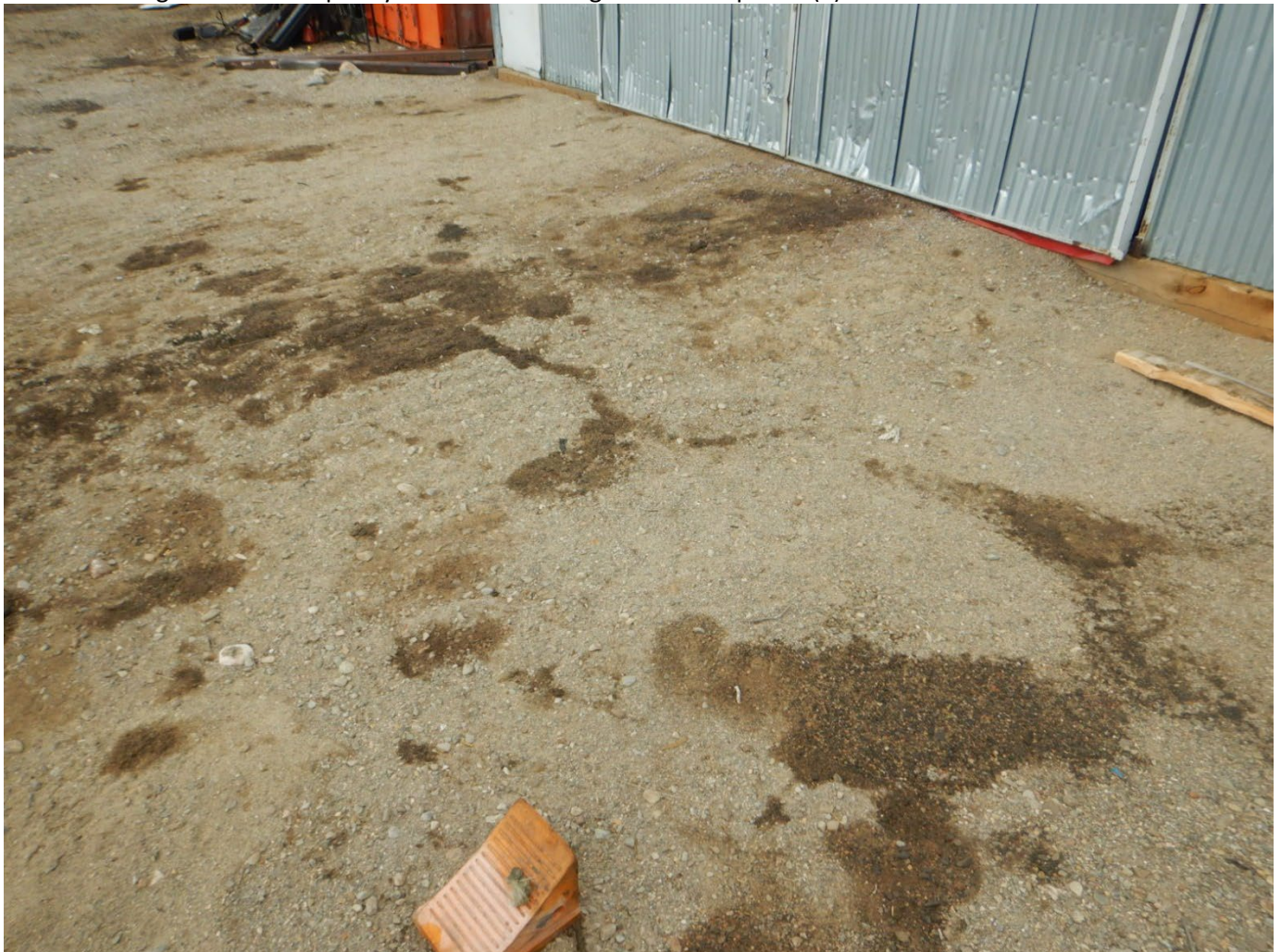
Photo 8 - Margaret Lake Camp – Hydrocarbon staining outside shop area (1).
