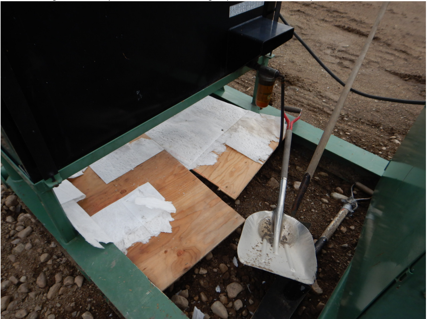
Photo 6 – Margaret Lake Camp – Incinerator Area - Leakage repaired and absorbents placed.
