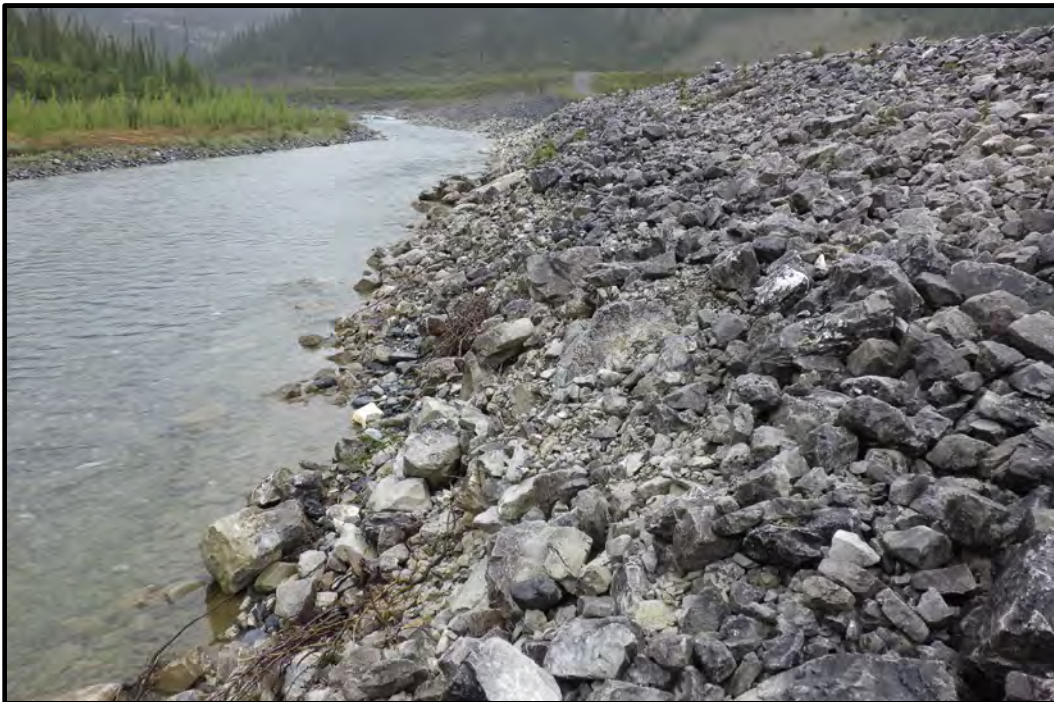
Photo A8: Flood Protection Berm, toe of creek side slope looking upstream from near Monitoring Site NHC-03. Riprap erosion and oversteepening shown along slope. (photo taken August 20, 2024)
