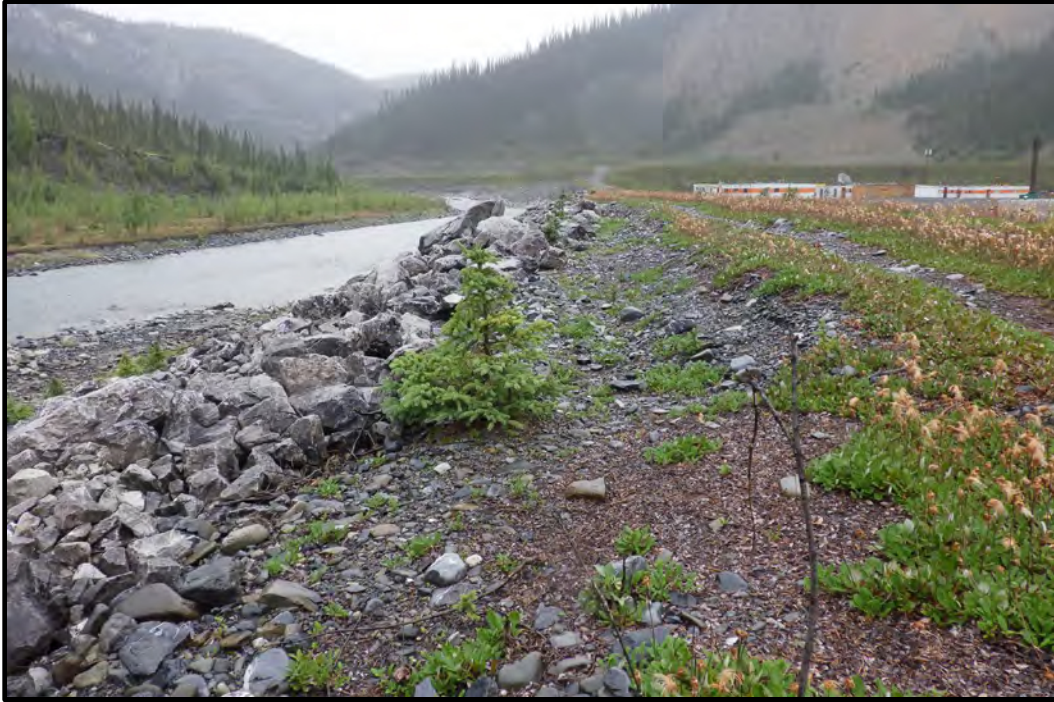
Photo A7: Flood Protection Berm, crest of creek side slope looking upstream from near Monitoring Site NHC-01. Riprap settlement shown along crest of berm. (photo taken August 20, 2024)
