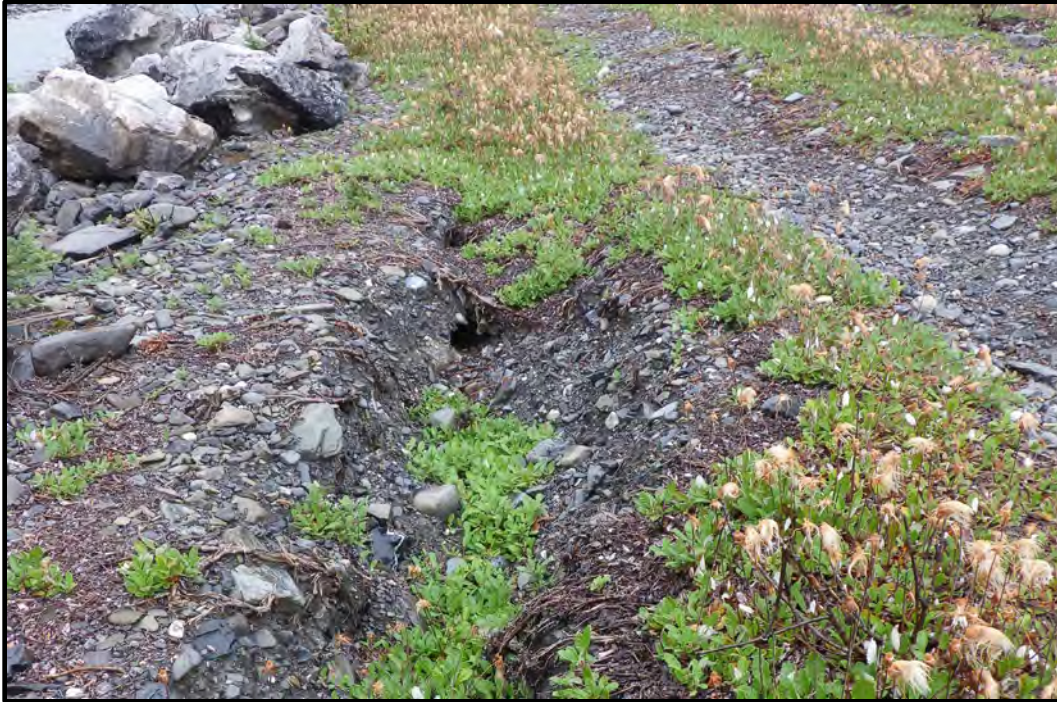
Photo A11: Flood Protection Berm, crest of creek side slope looking upstream from between Monitoring Sites NHC-03 and NHC-04. Old animal burrow and tension crack shown. (photo taken August 20, 2024)
