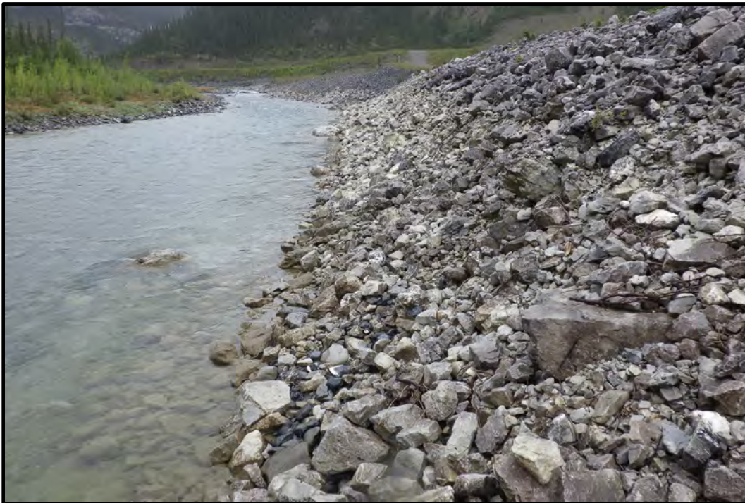
Photo A12: Flood Protection Berm, toe of creek side slope looking upstream from near Monitoring Site NHC-04. Riprap erosion and oversteepening shown along slope. (photo taken August 20, 2024)
