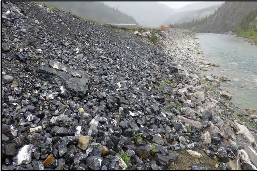
Photo A19: Flood Protection Berm, toe of creek side slope looking downstream from location of 2009 riprap repairs (NHC 2009, Repair Site “C”). (photo taken August 20, 2024)
