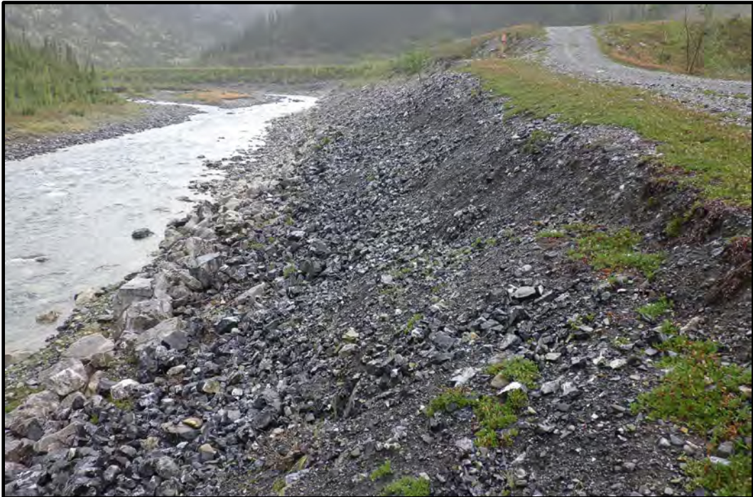
Photo A16: Flood Protection Berm, crest of creek side slope looking upstream from location of 2009 riprap repairs (NHC 2009, Repair Site "C"). (photo taken August 20, 2024)
