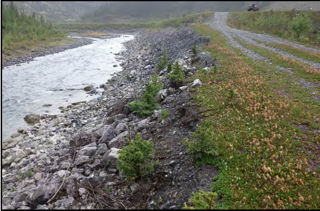
Photo A15: Flood Protection Berm, crest of creek side slope looking upstream from near Monitoring Site NHC-05. Riprap settlement shown along crest of berm. (photo taken August 20, 2024)
