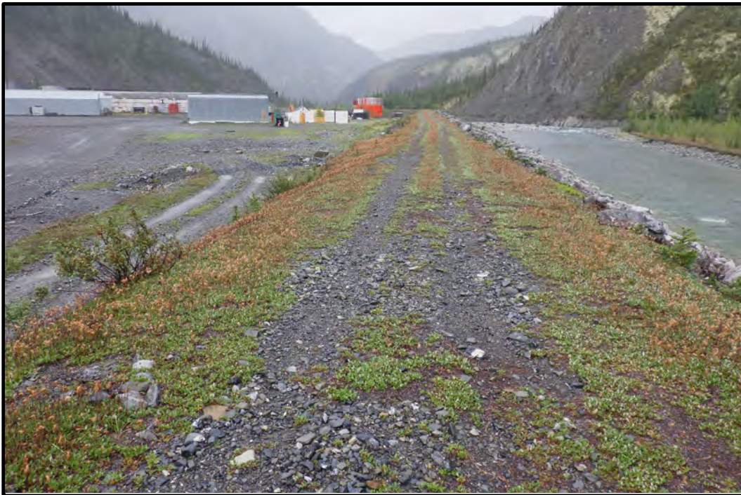
Photo A20: Flood Protection Berm Top of berm looking downstream from connection with Water Storage Pond. (photo taken August 20, 2024)
