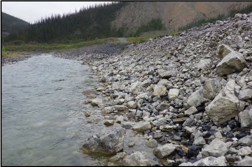
Photo A14: Flood Protection Berm, toe of creek side slope looking upstream from between Monitoring Sites NHC-04 and NHC-05. Riprap erosion and oversteepening shown. (photo taken August 20, 2024)
