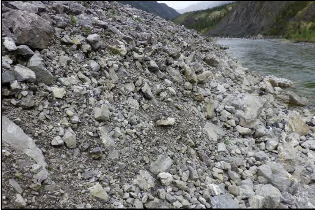
Photo A17: Flood Protection Berm, middle of creek side slope looking downstream near Monitoring Site NHC-05. Riprap erosion and oversteepening shown. (photo taken August 20, 2024)
