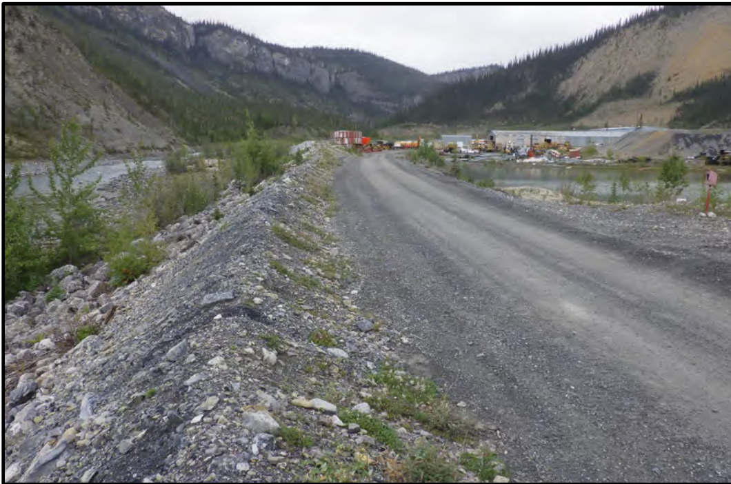
Photo A2: Flood Protection Berm Crest of creek side slope looking upstream from Harrison Creek culverts. (photo taken August 20, 2024)
