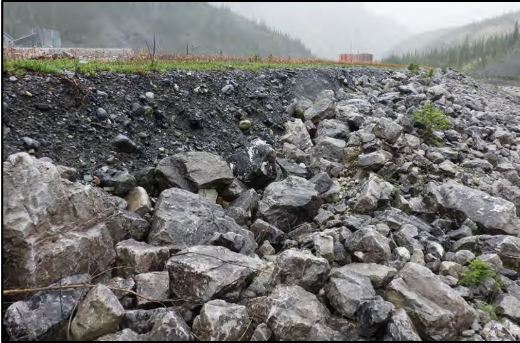
Photo A9: Flood Protection Berm, crest of creek side slope looking downstream from near Monitoring Site NHC-03. Riprap settlement shown along crest of berm. (photo taken August 20, 2024)
